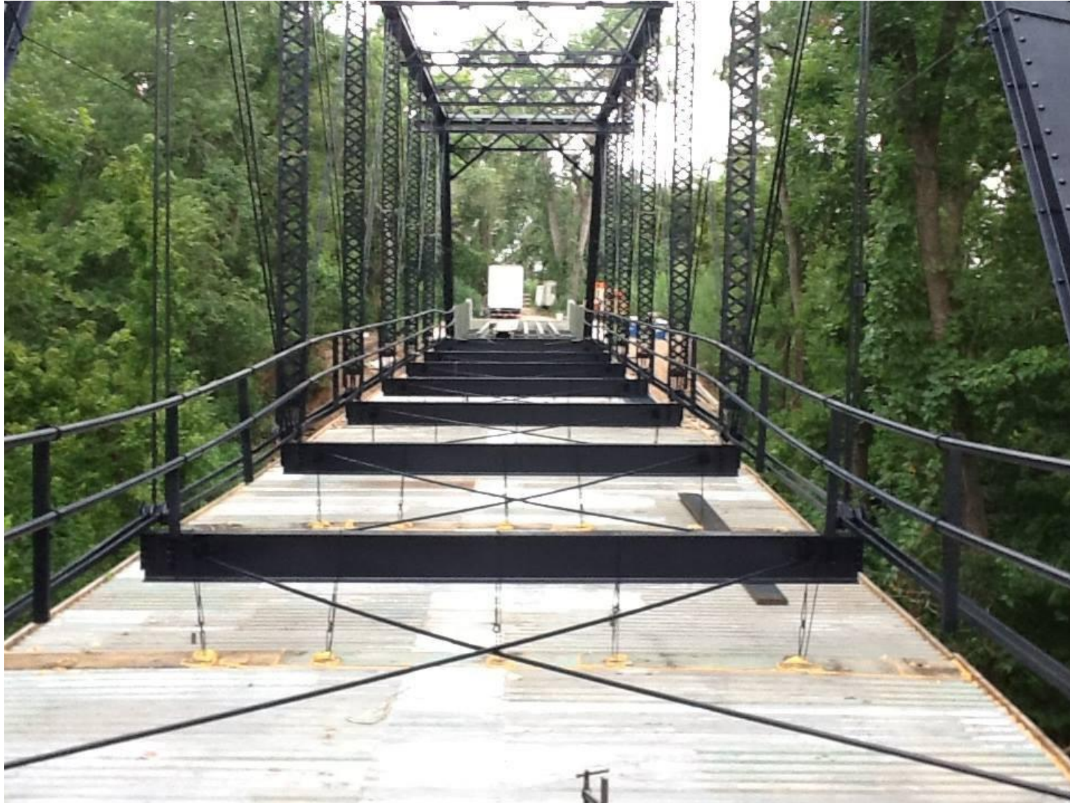
Restored and repainted truss awaiting deck stringers and a new deck.
