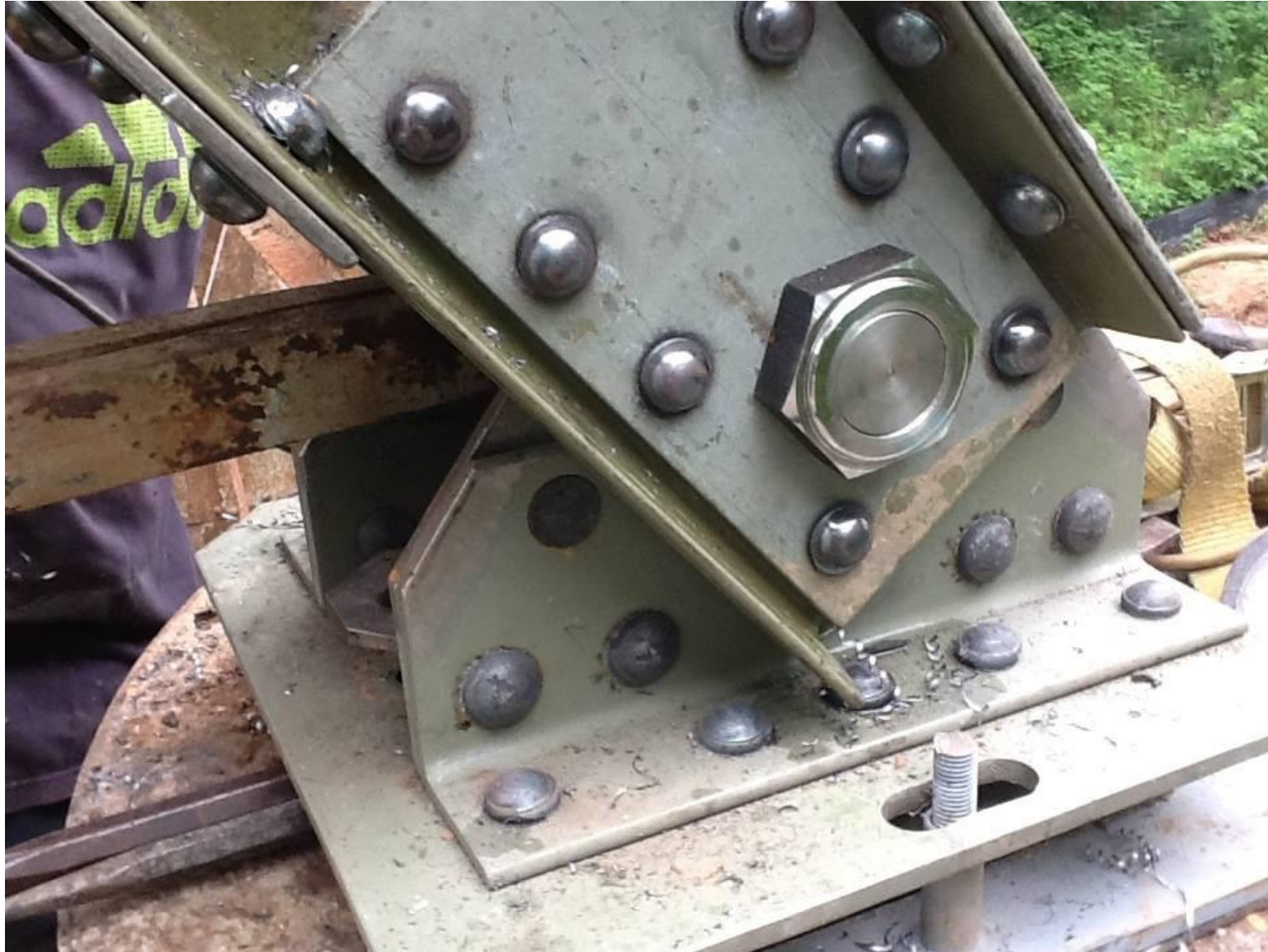
Replicated bridge shoe and endpost base.
