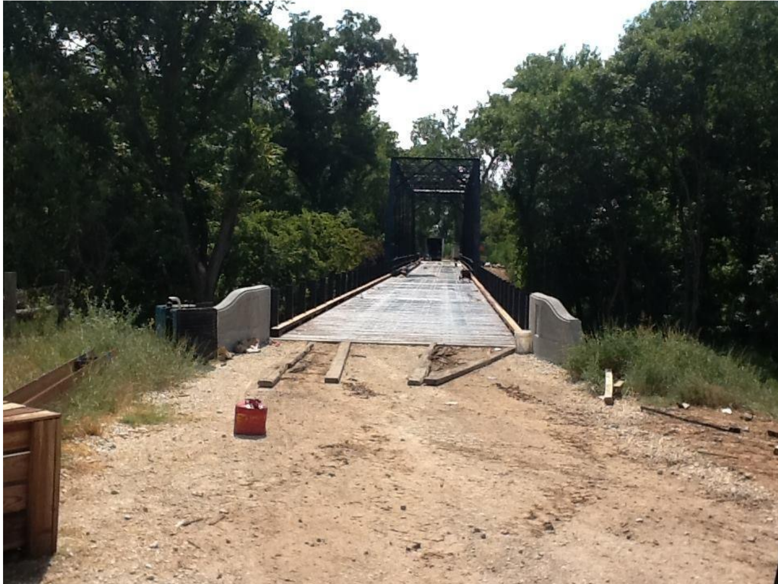
Bridge with new deck in place.
