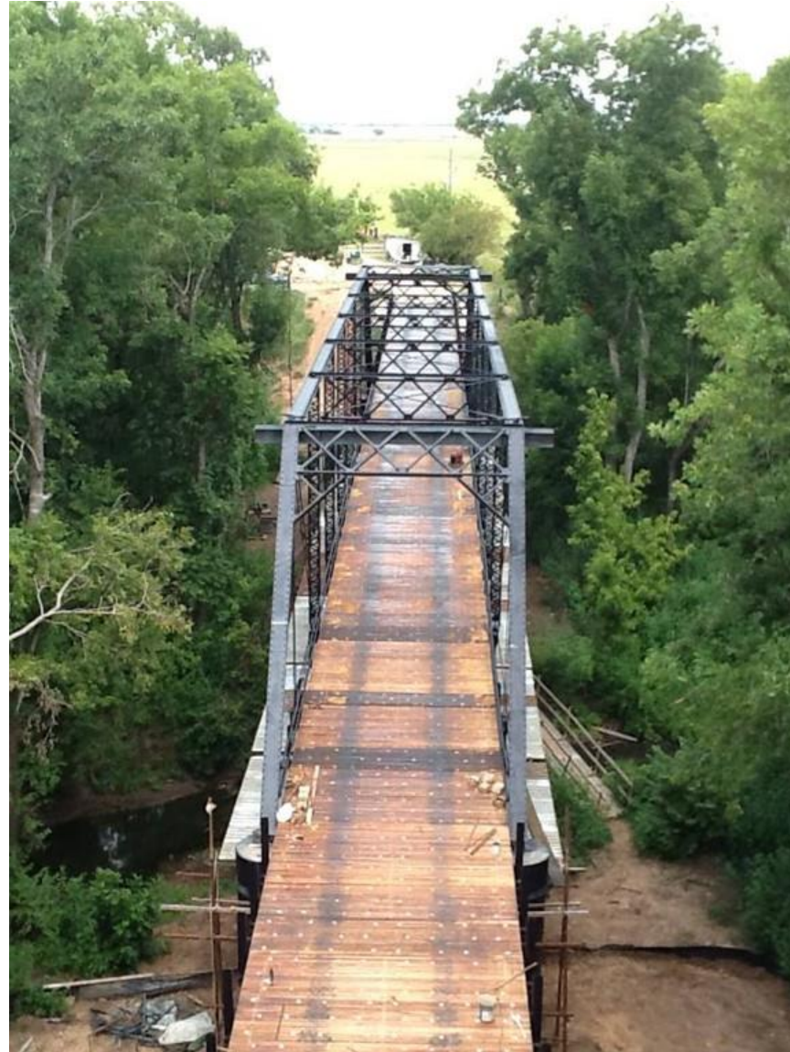
Bridge with new deck in place.
