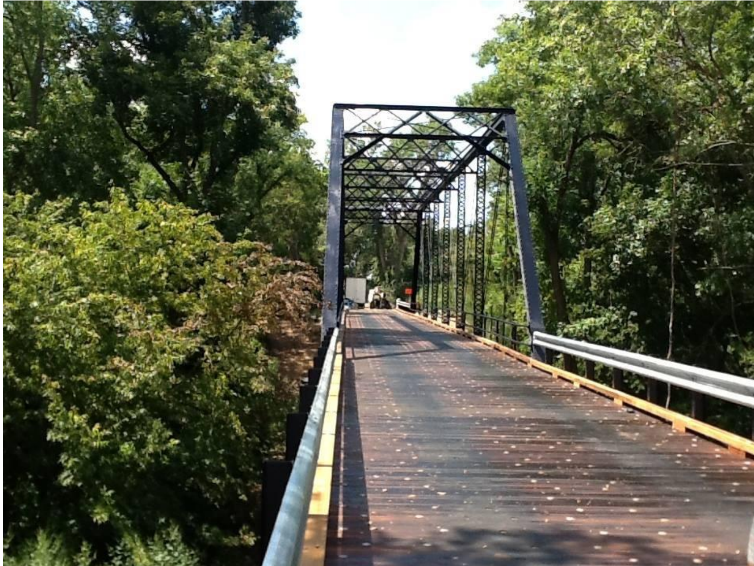
Restored truss with new deck installed.
