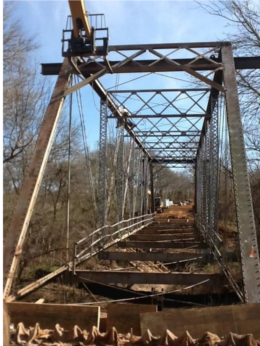
Truss before restoration, after deck removal.
