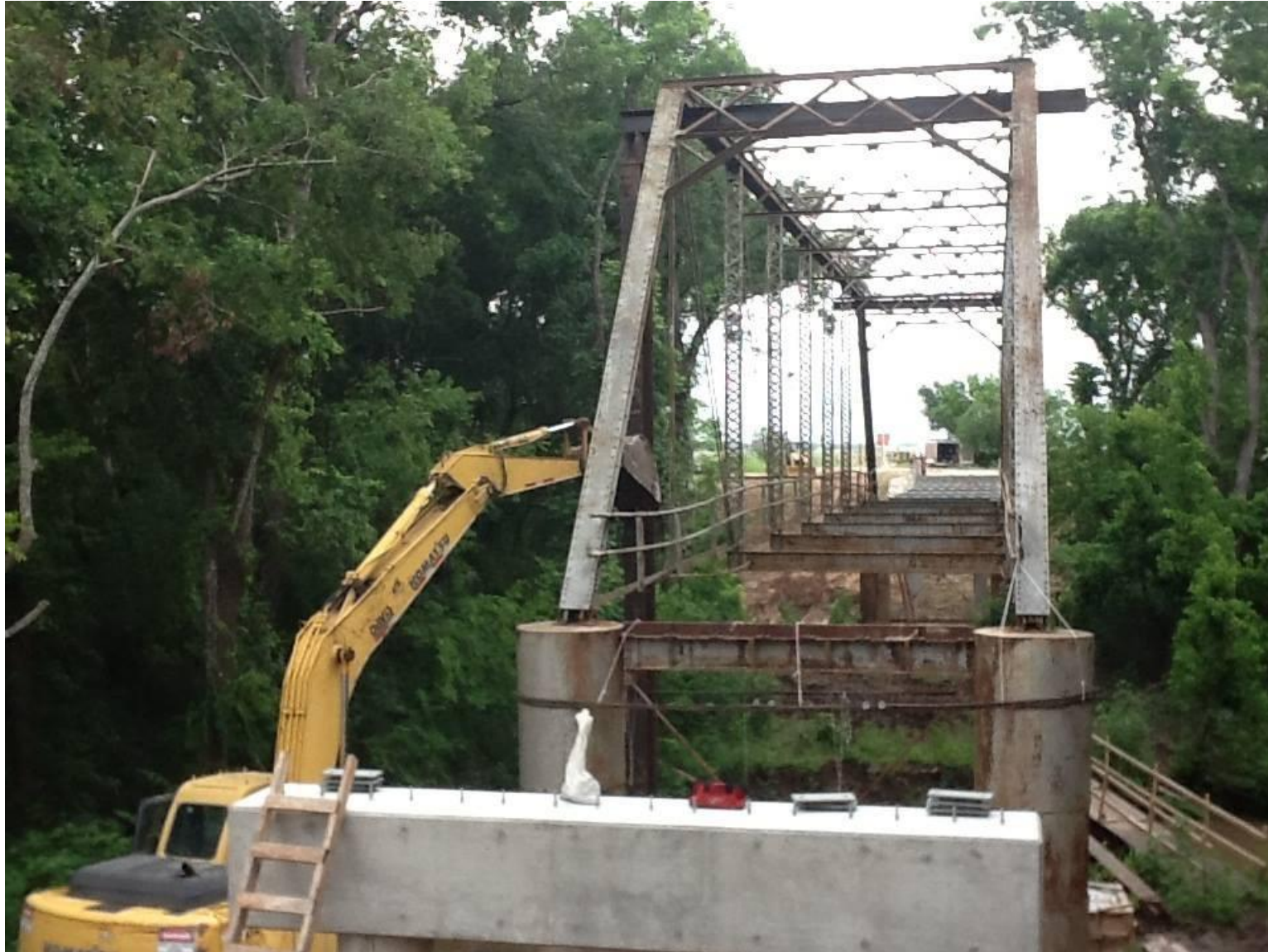
Truss before restoration, after deck removal.
