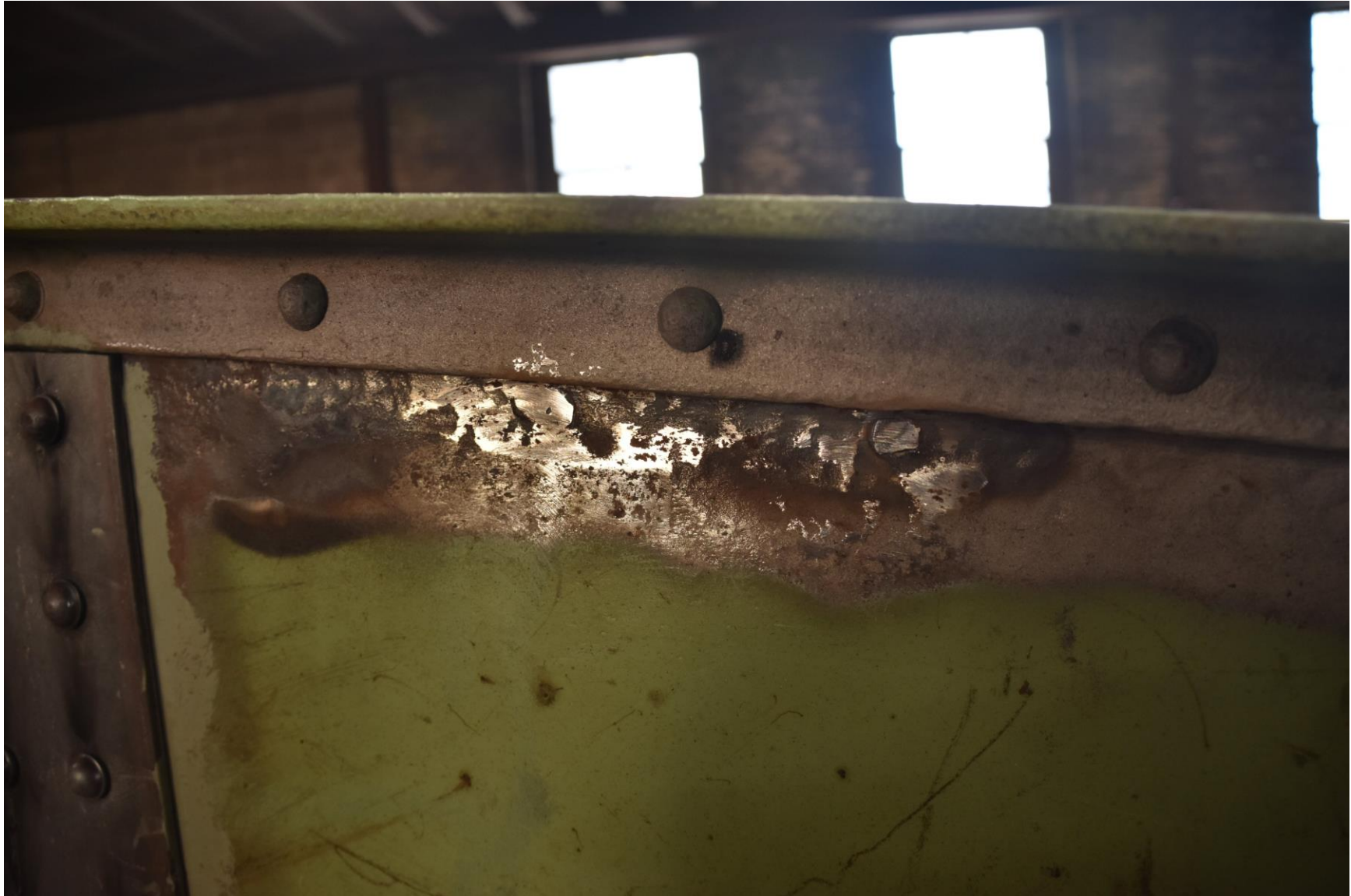
Shop Repairs (Pad Welding For Section Loss)
