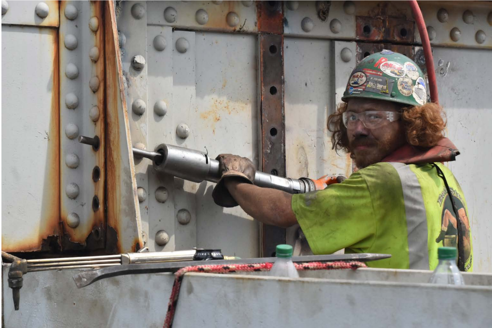
Rivet removal without damage to parent metal.
