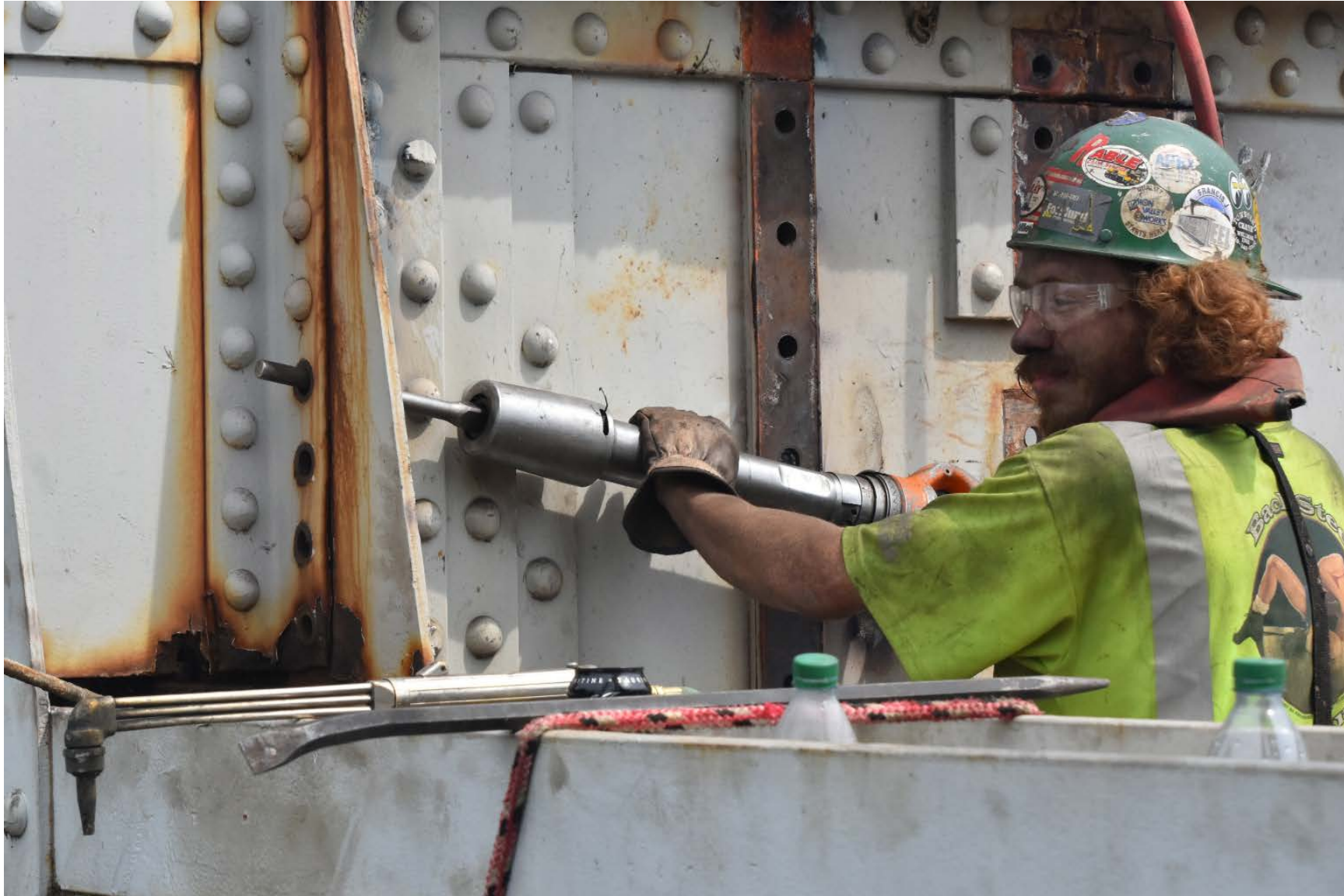
Rivet removal without damage to parent metal.
