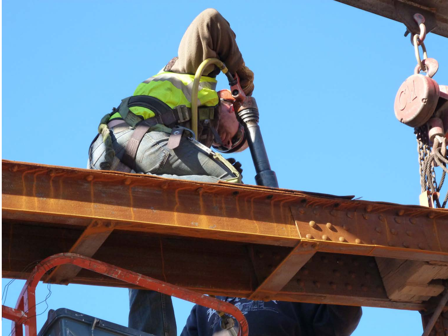
Rivet removal without damage to parent metal.
