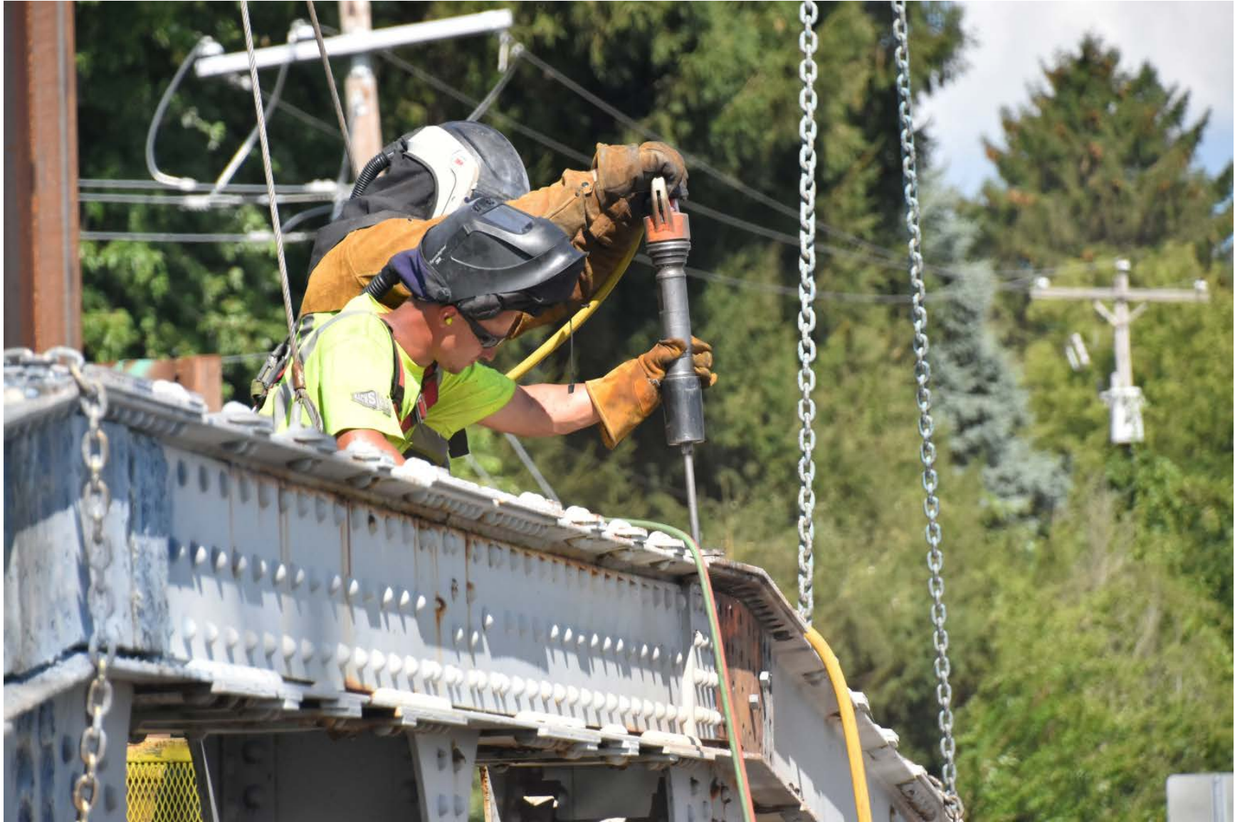
Rivet removal without damage to parent metal.
