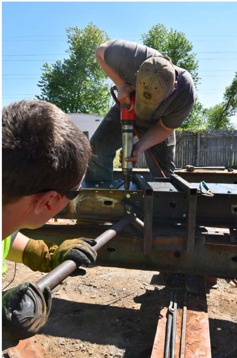
Hot riveting with manual bucking bar.
