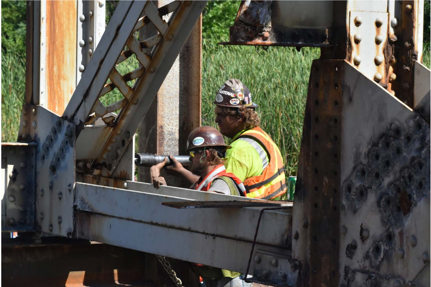
Rivet removal without damage to parent metal.
