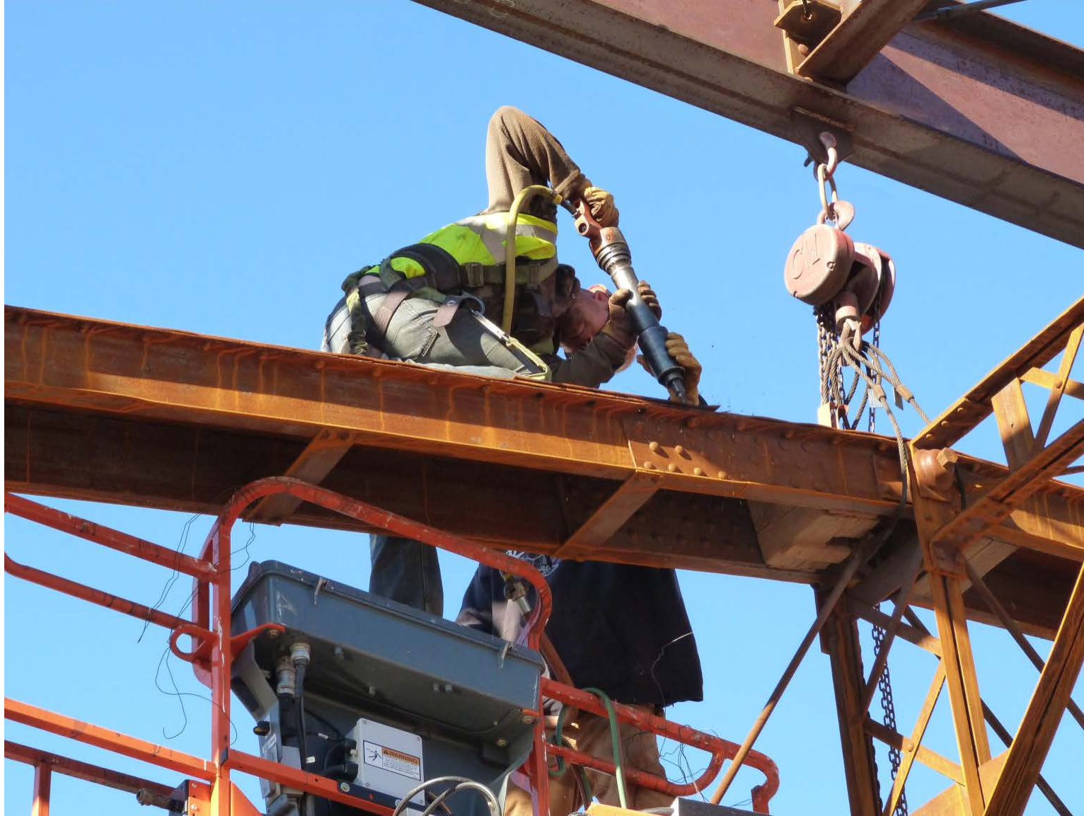
Rivet removal without damage to parent metal.
