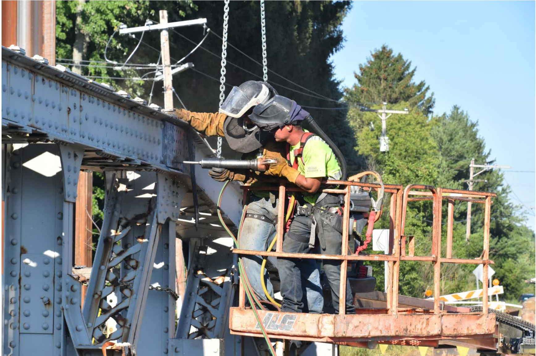
Rivet removal without damage to parent metal.
