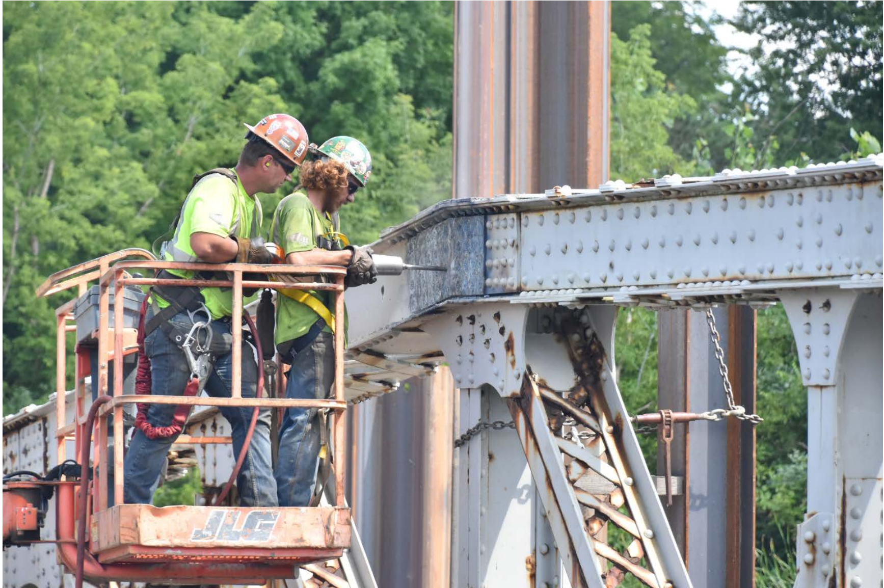
Rivet removal without damage to parent metal.
