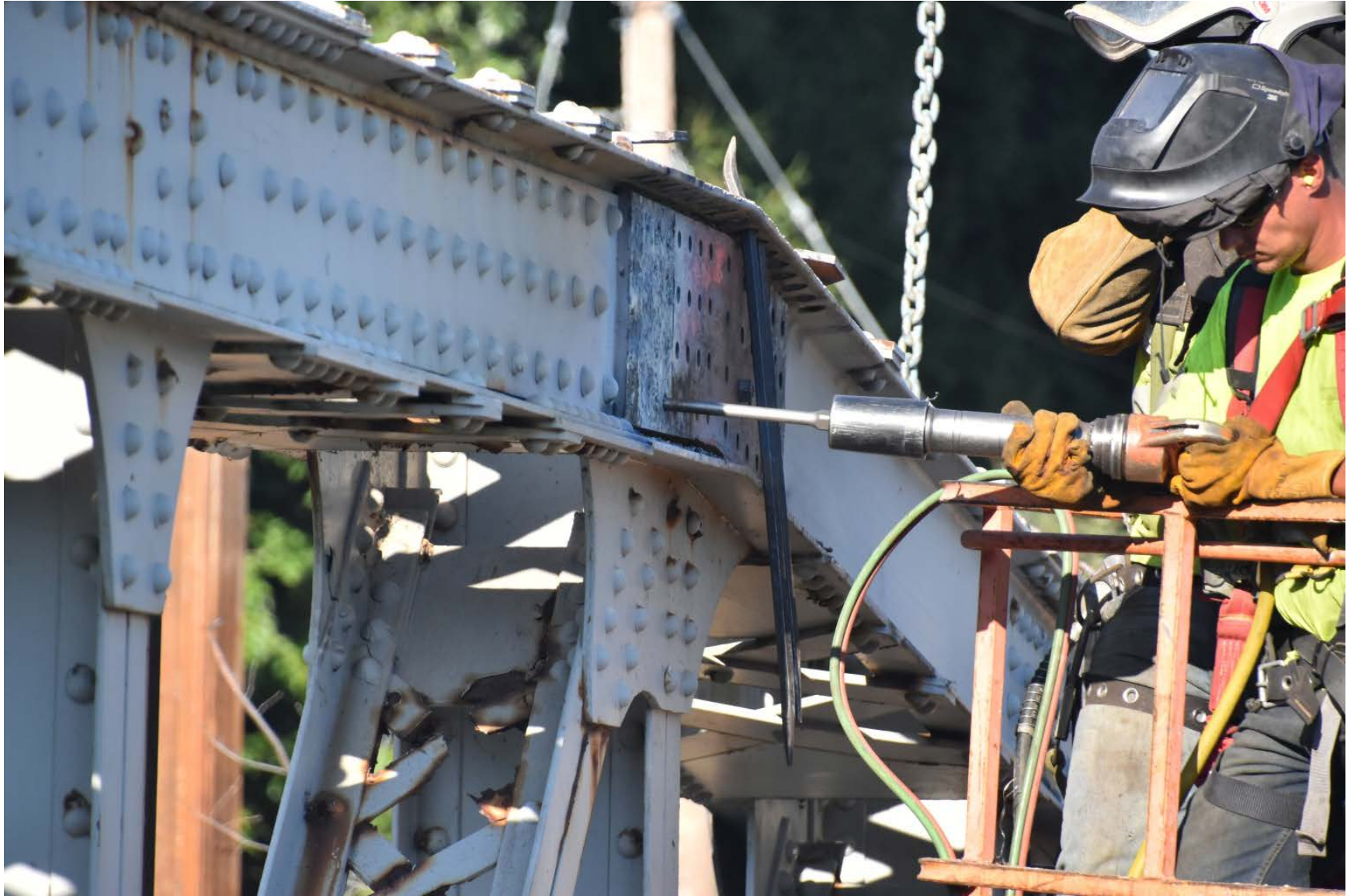
Rivet removal without damage to parent metal.
