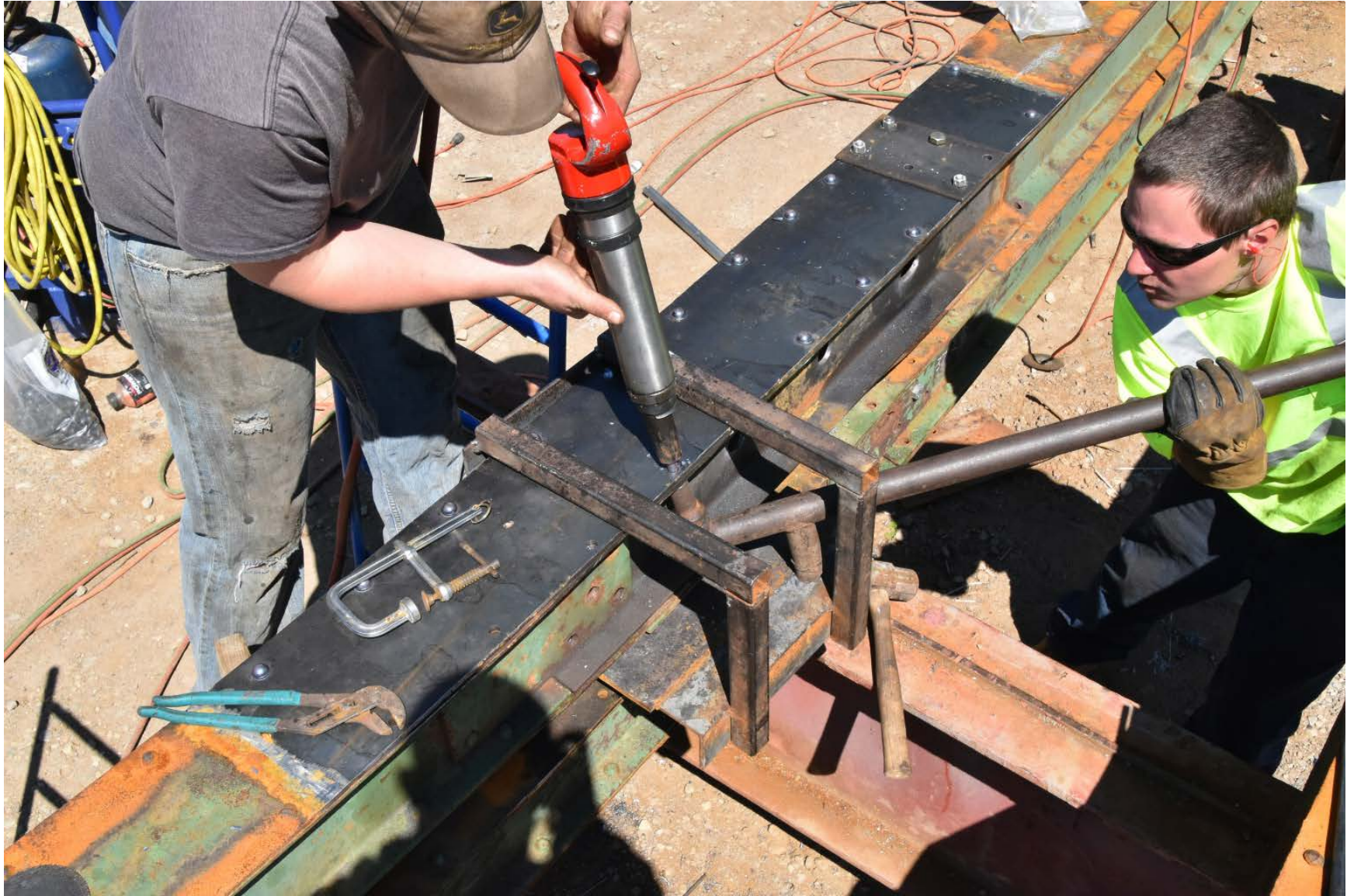
Hot riveting with manual bucking bar.
