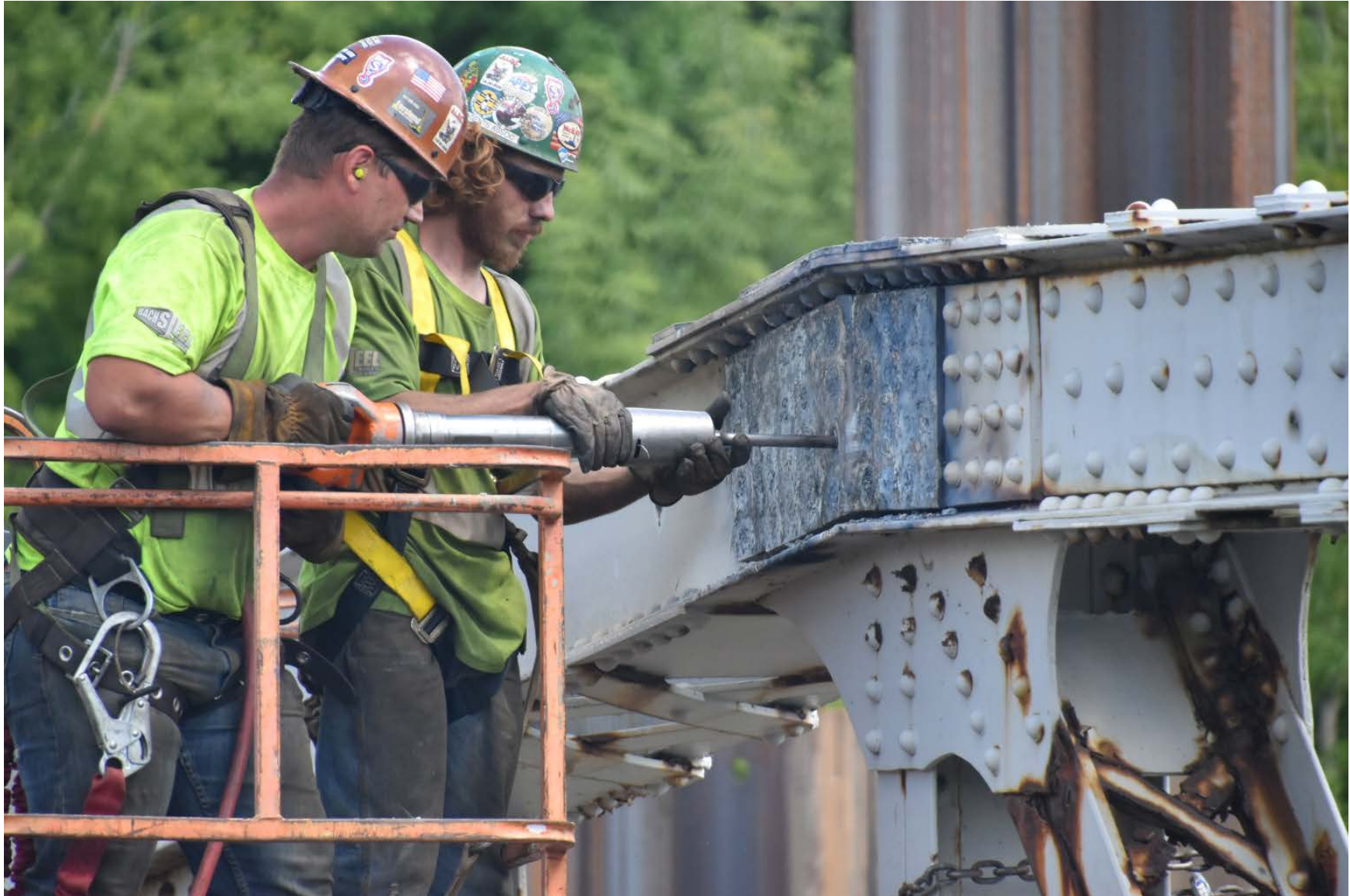
Rivet removal without damage to parent metal.
