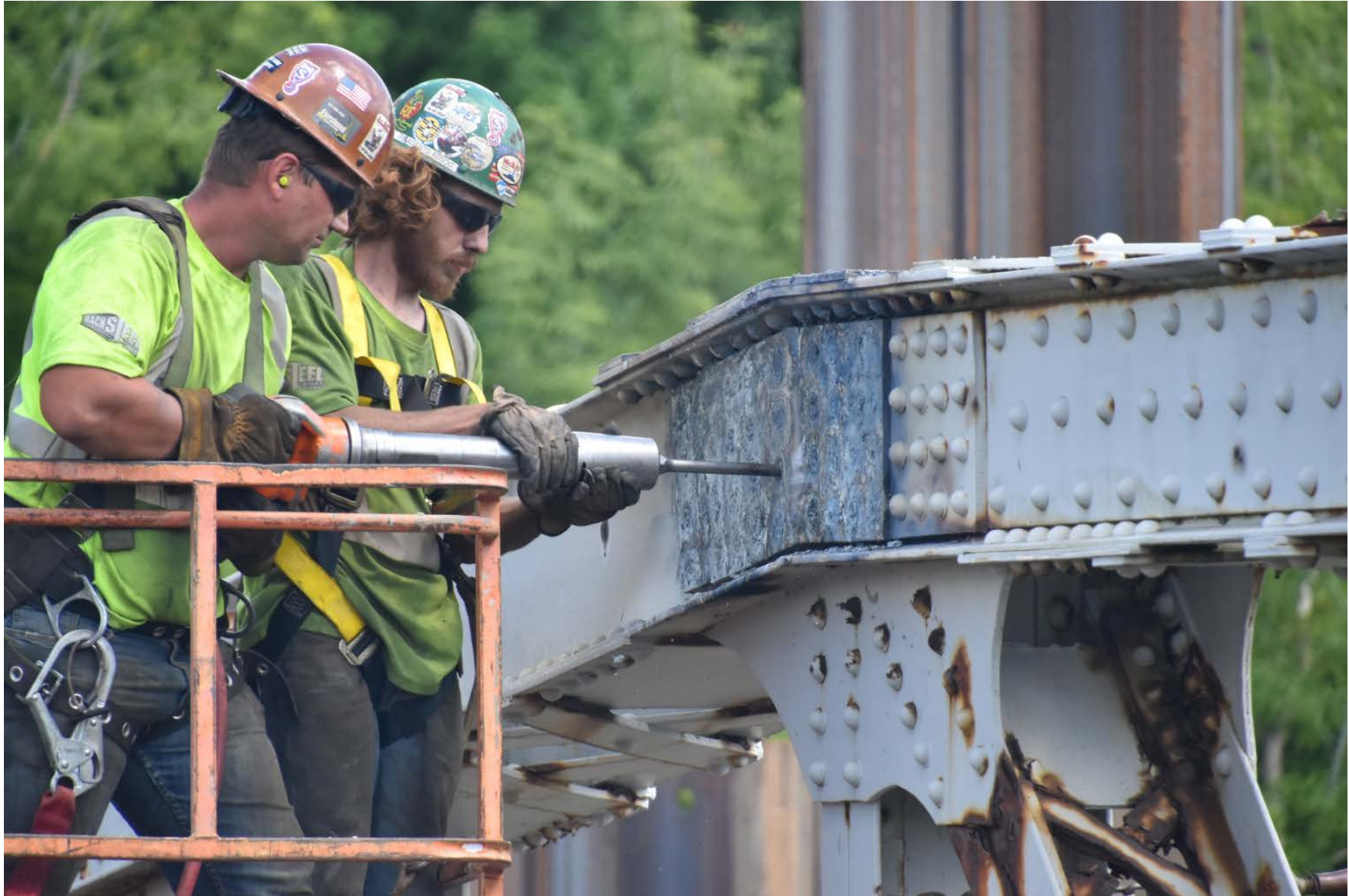
Rivet removal without damage to parent metal.
