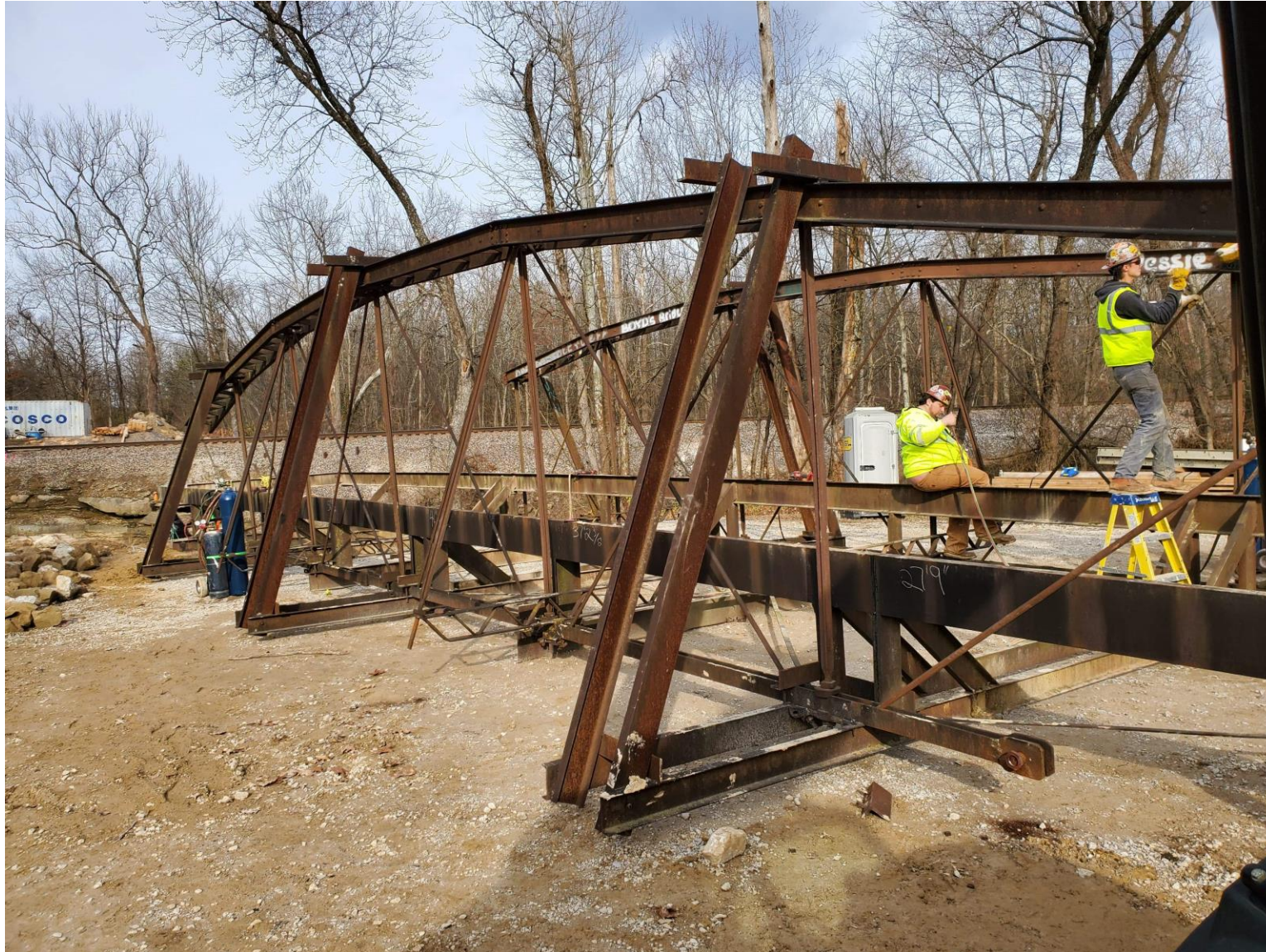
Disassembly including removal of modern outriggers.
