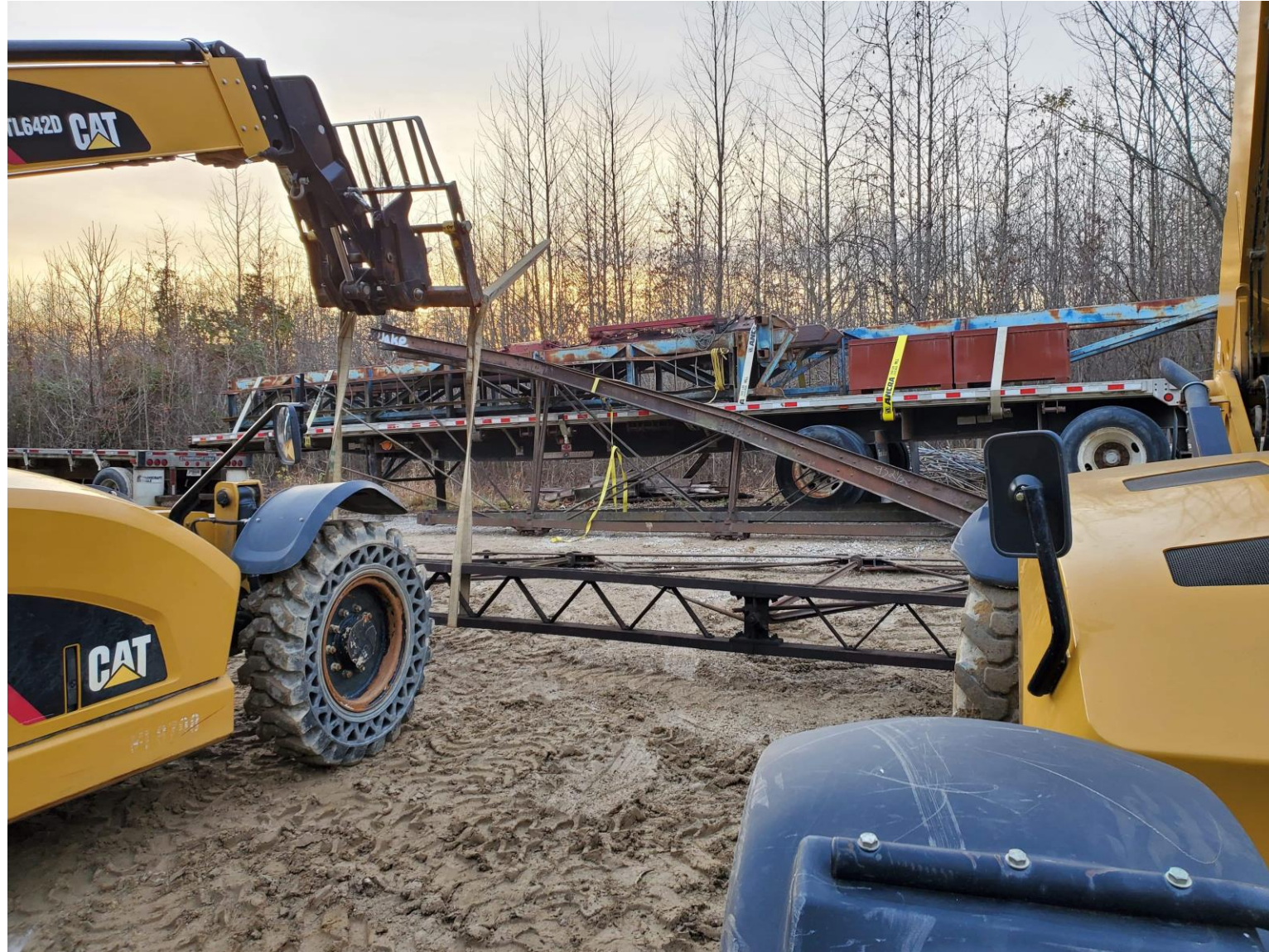
Disassembly including removal of modern outriggers.
