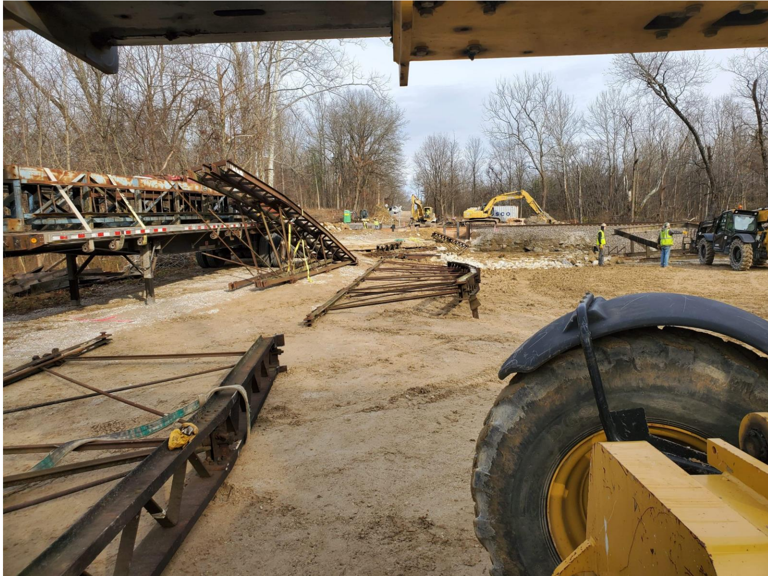
Disassembly including removal of modern outriggers.
