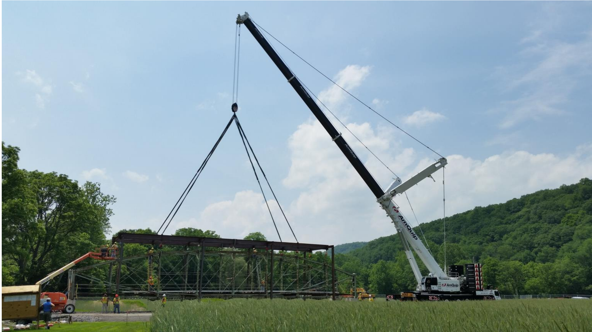
Truss Removal
