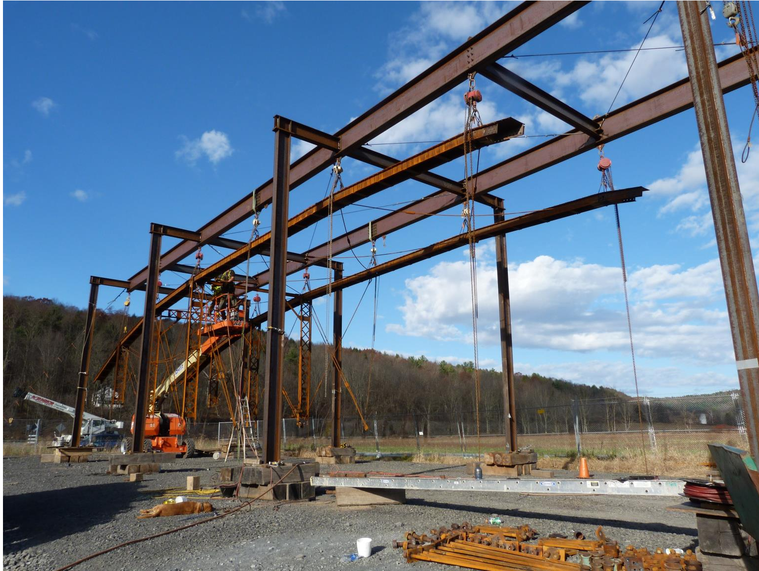
Truss Disassembly
