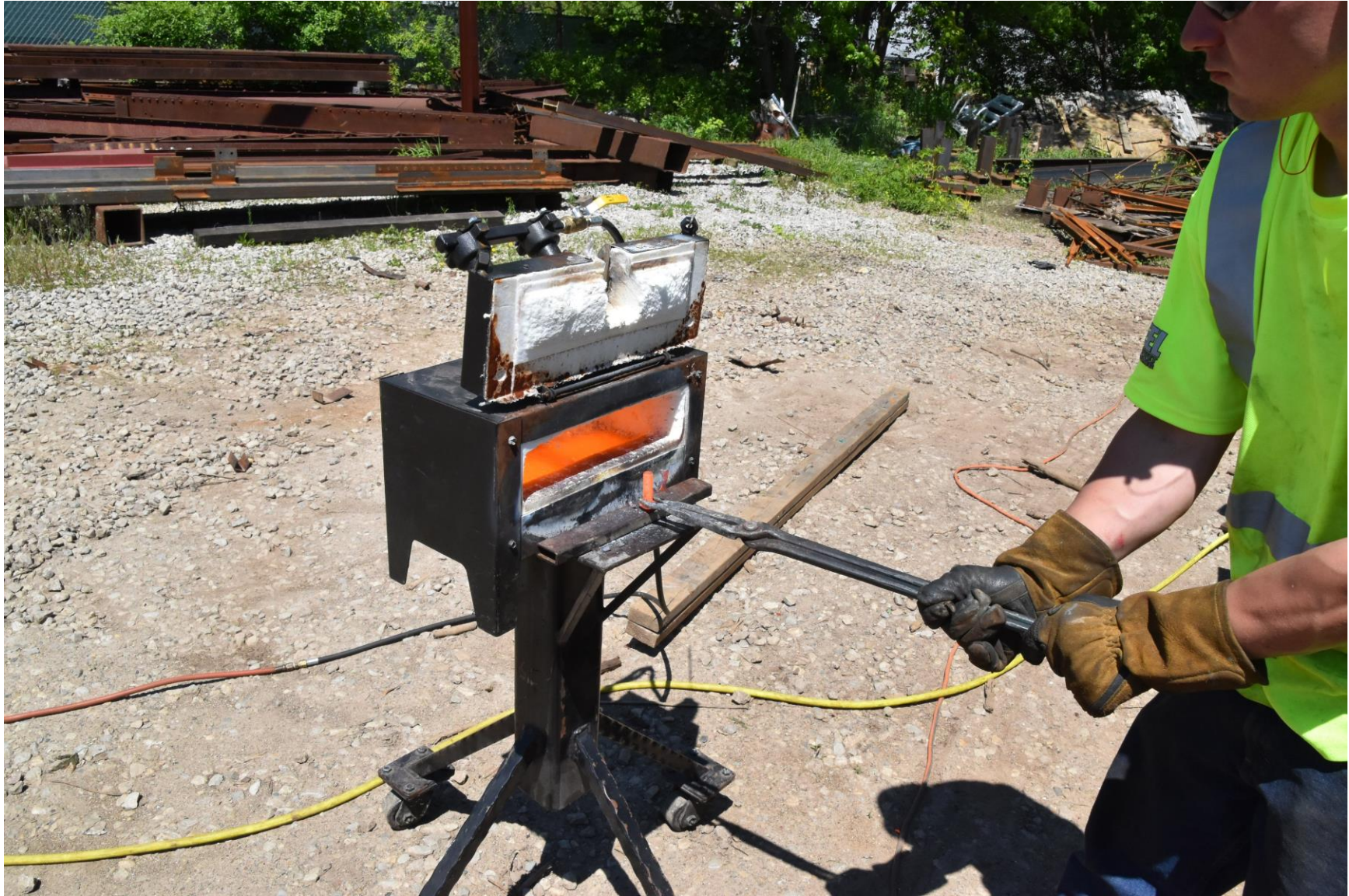
Hot riveting upper chord.
