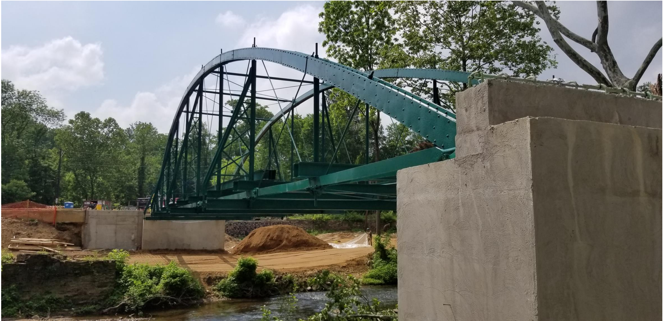
Truss on new abutments.
