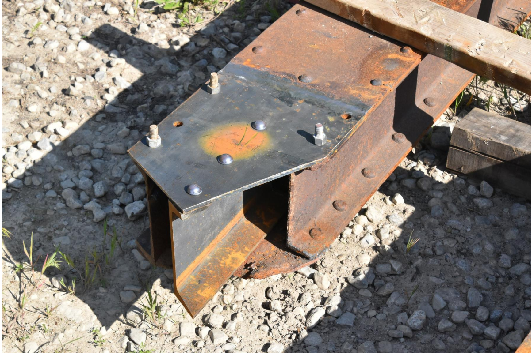
Upper chord repairs showing new rivets.
