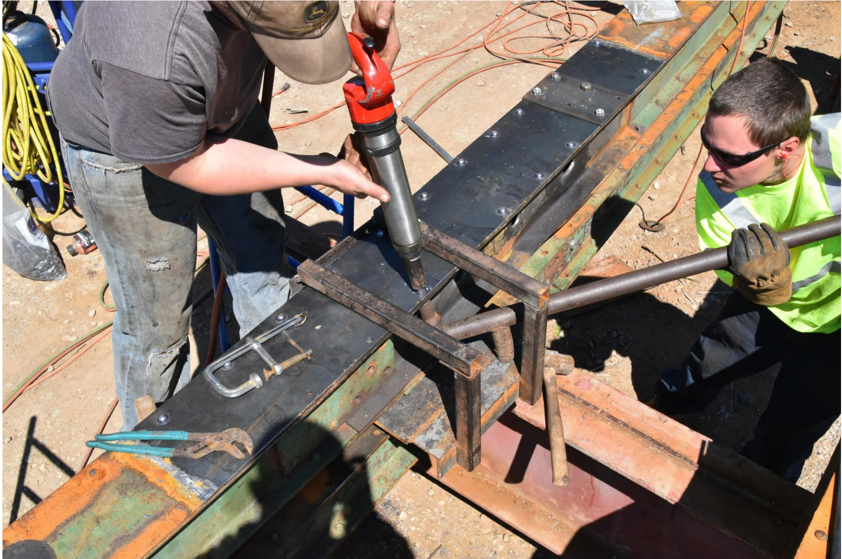
Hot riveting upper chord.
