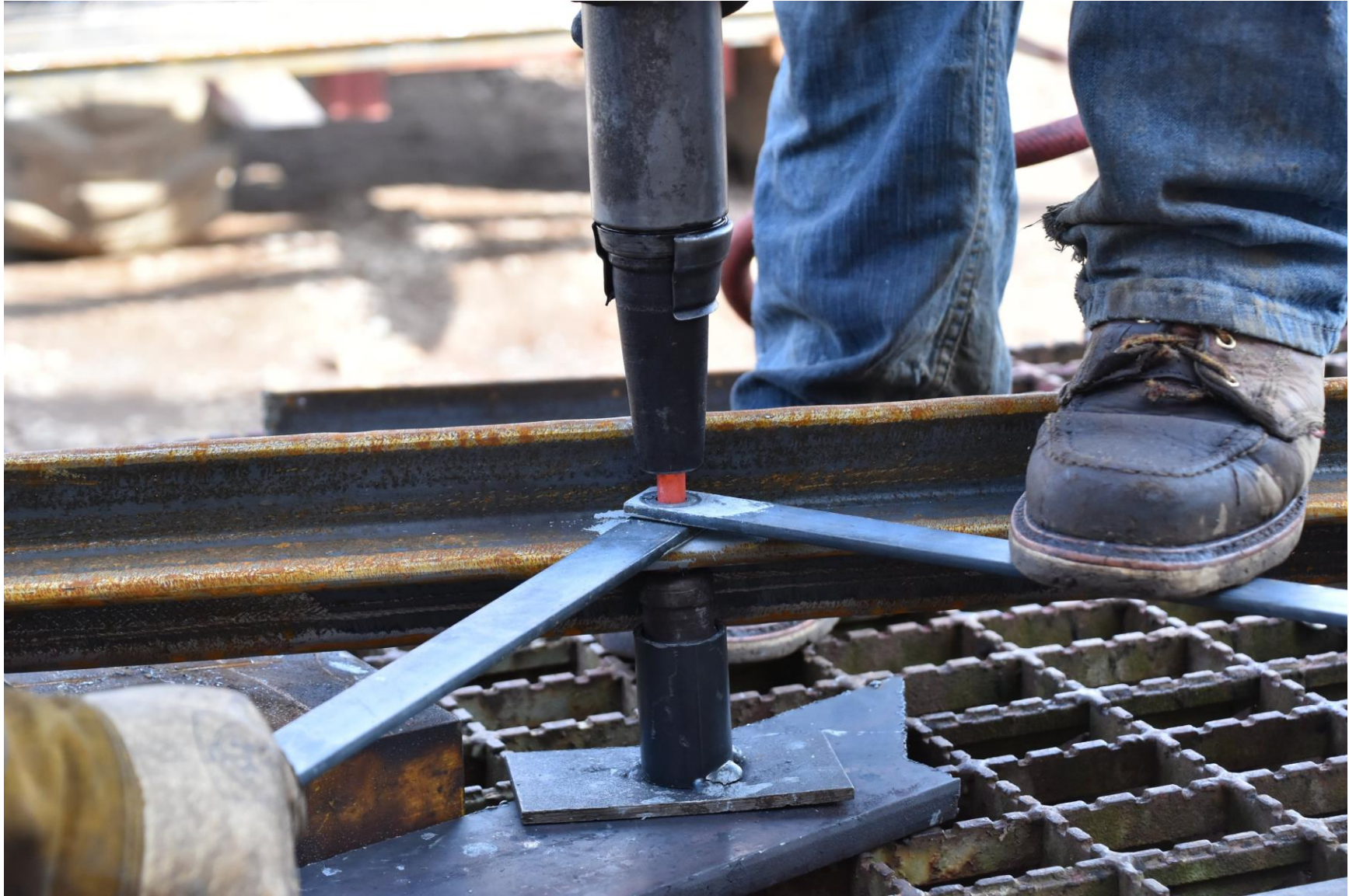
Hot riveting outriggers.
