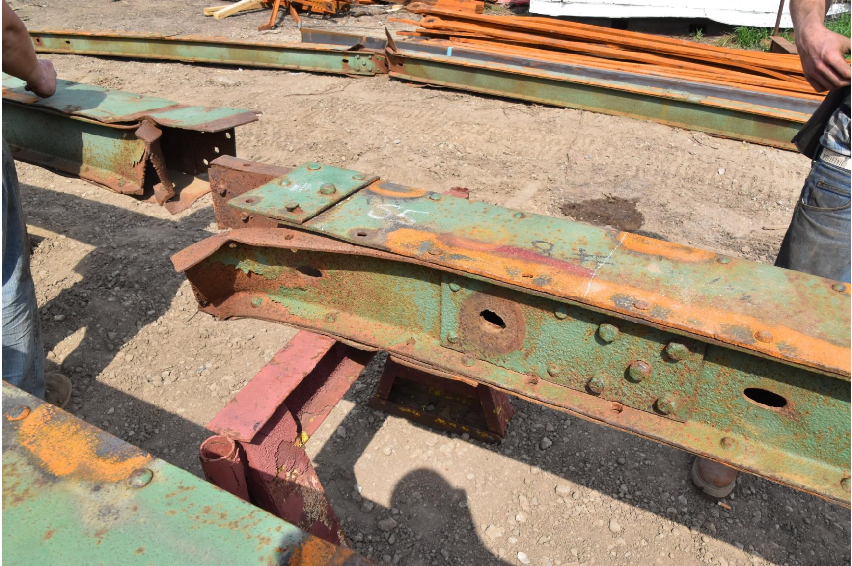
Upper chord damage prior to repairs.
