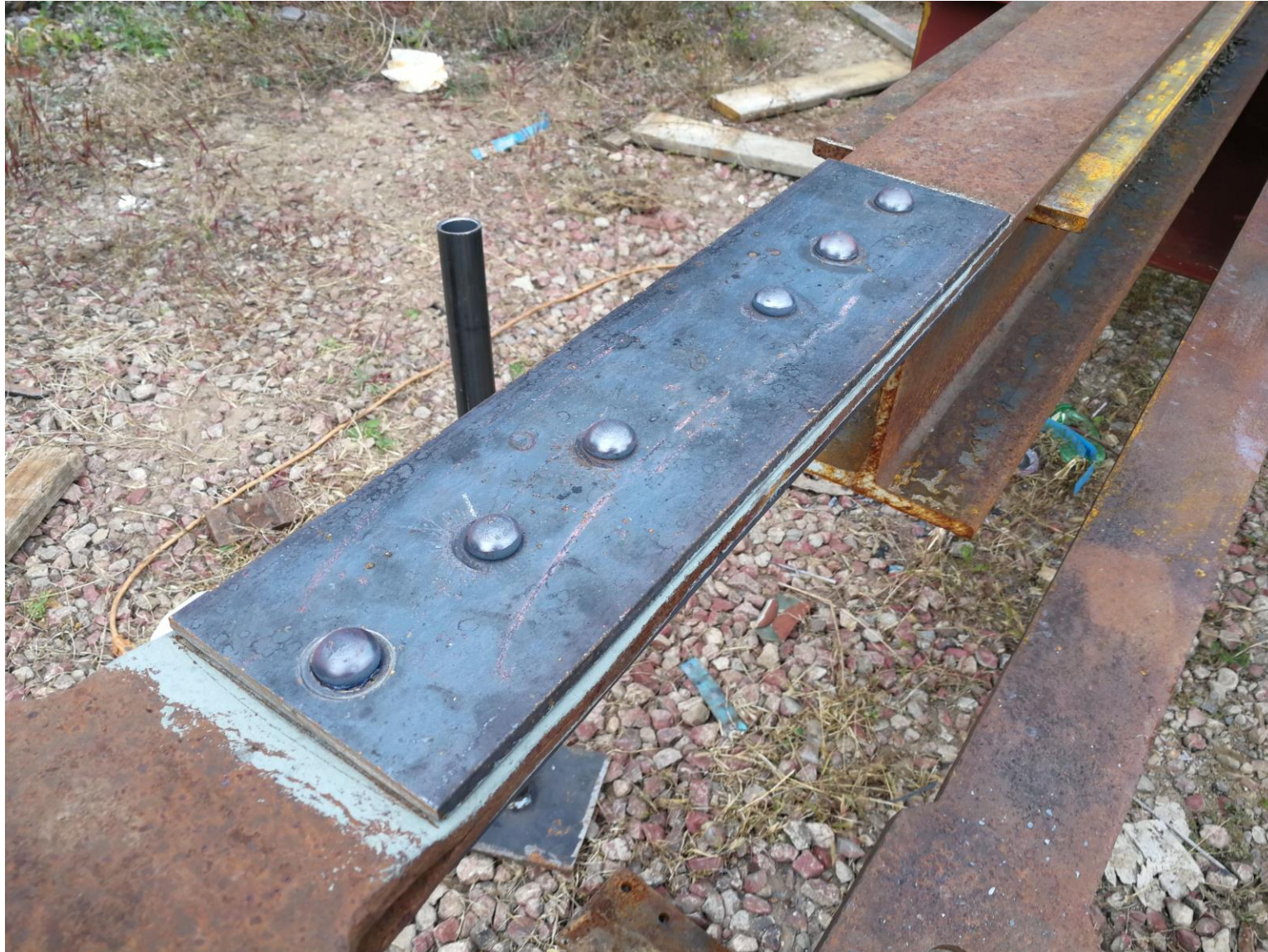
Bottom chord repairs showing new rivets.
