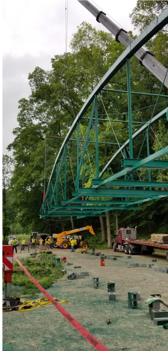
Picking the truss.
