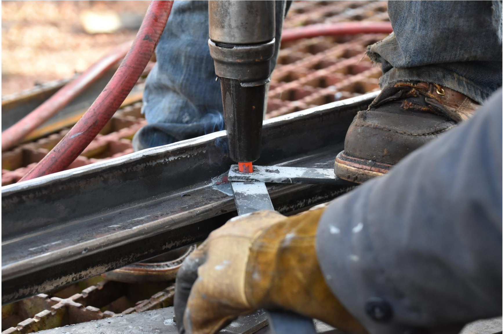
Hot riveting outriggers.
