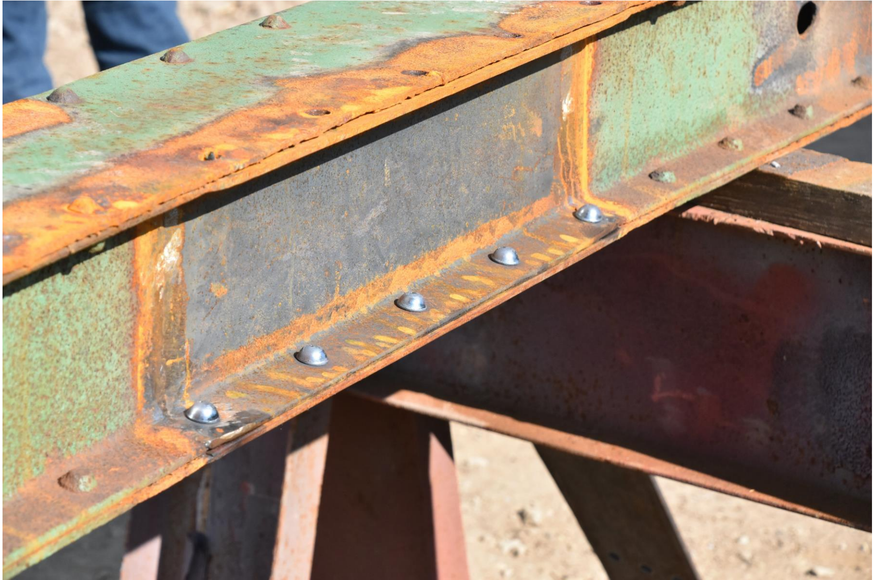
Upper chord repairs showing new rivets.
