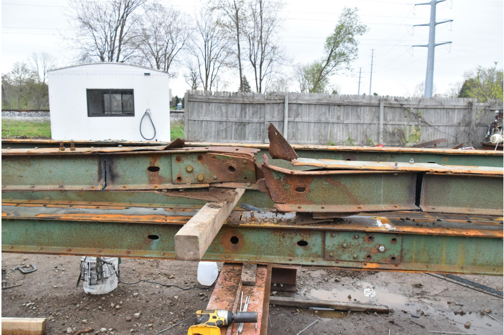
Upper chord damage prior to repairs.
