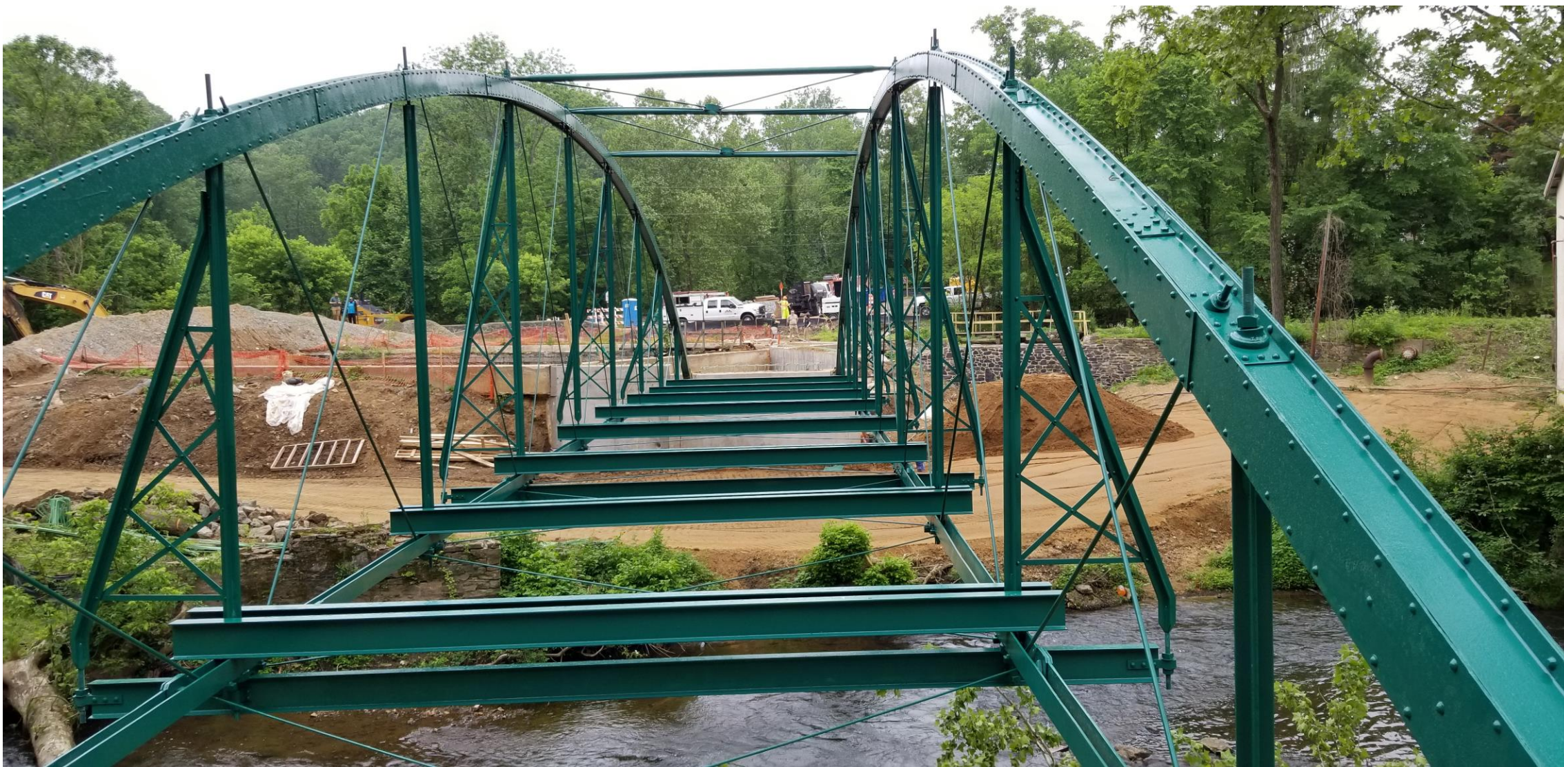
Truss on new abutments.
