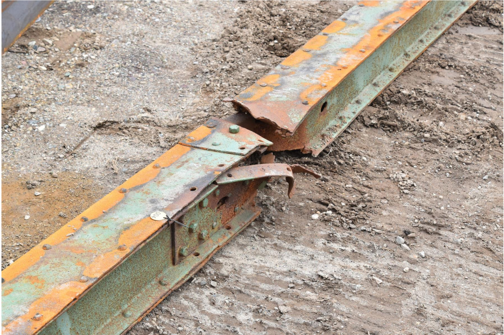
Upper chord damage prior to repairs.
