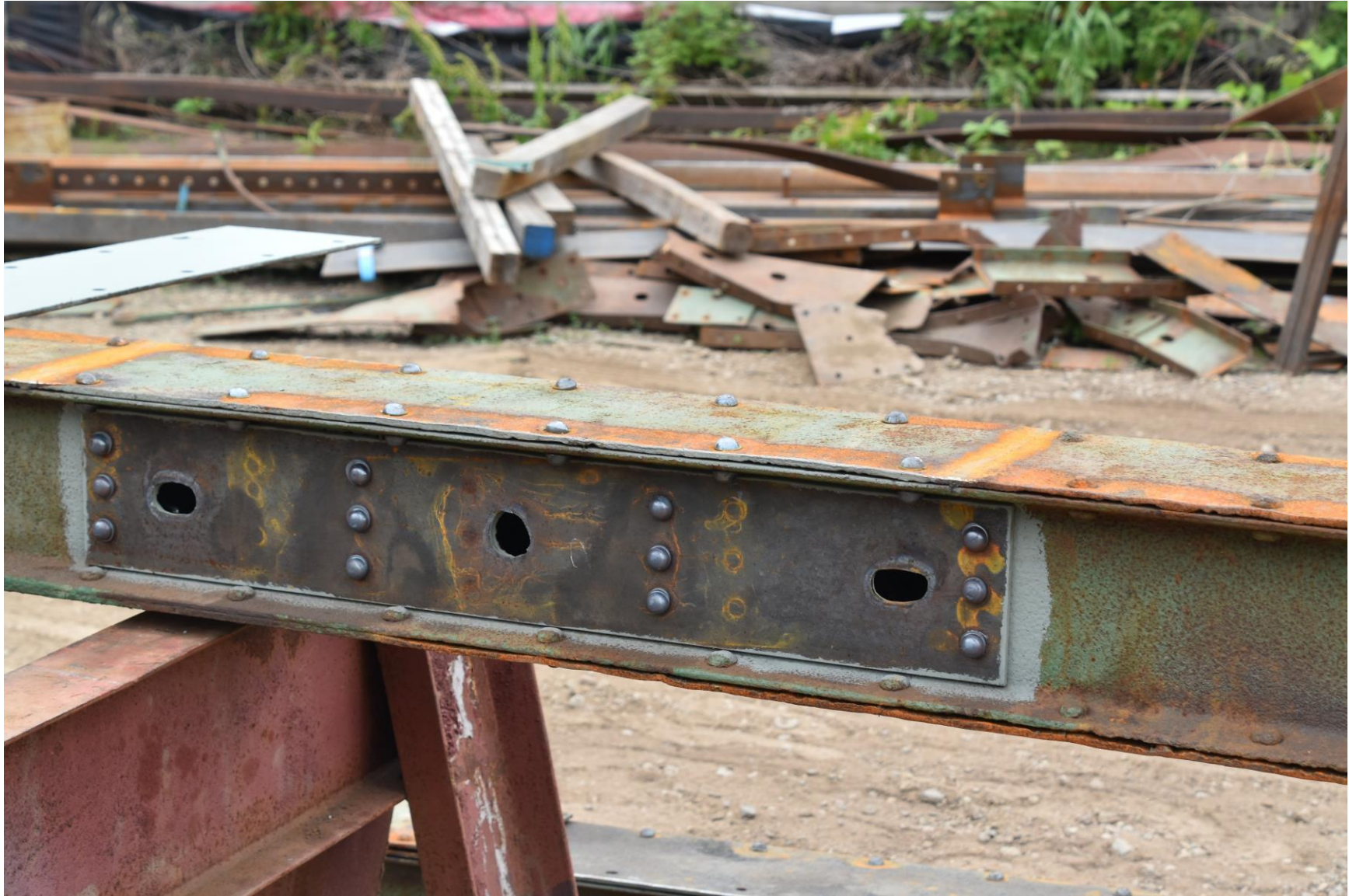
Upper chord repairs showing new rivets.
