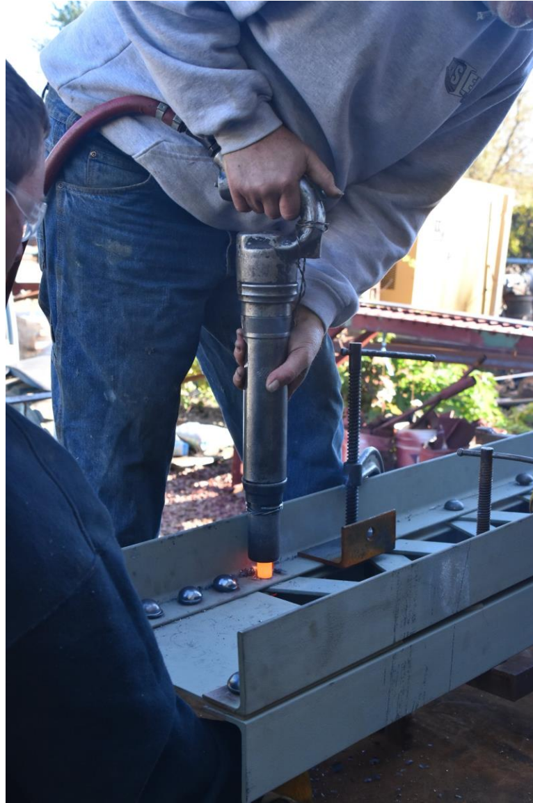
Hot riveting sway bracing.
