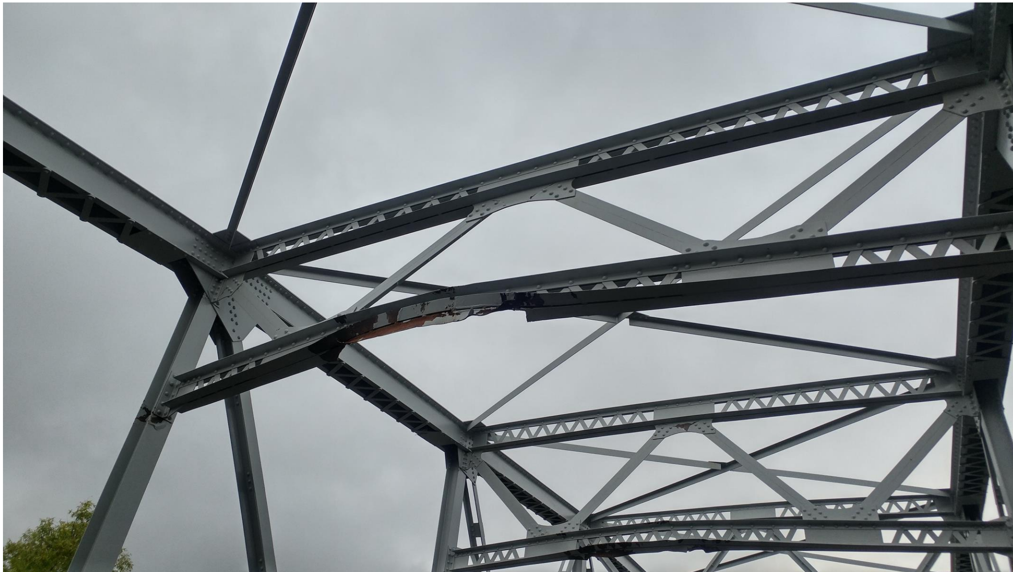
Bridge before repairs showing bracing damage.
