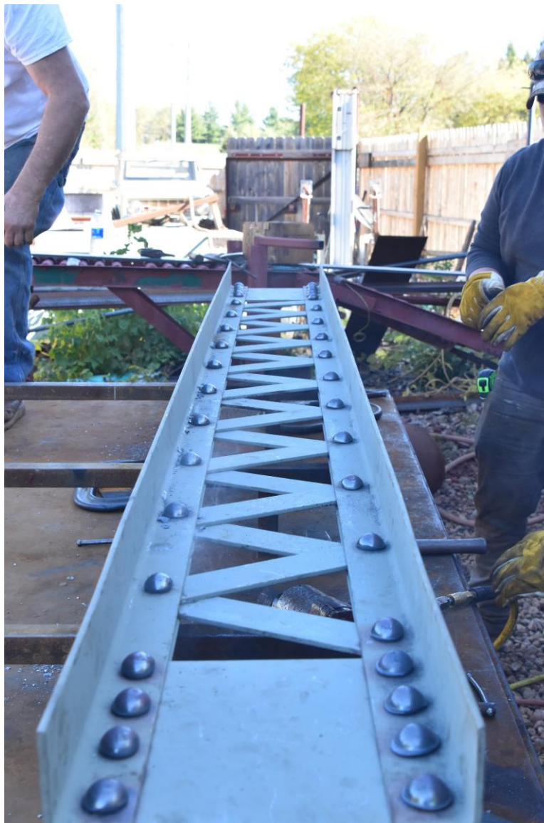
Completed replica bracing beam.
