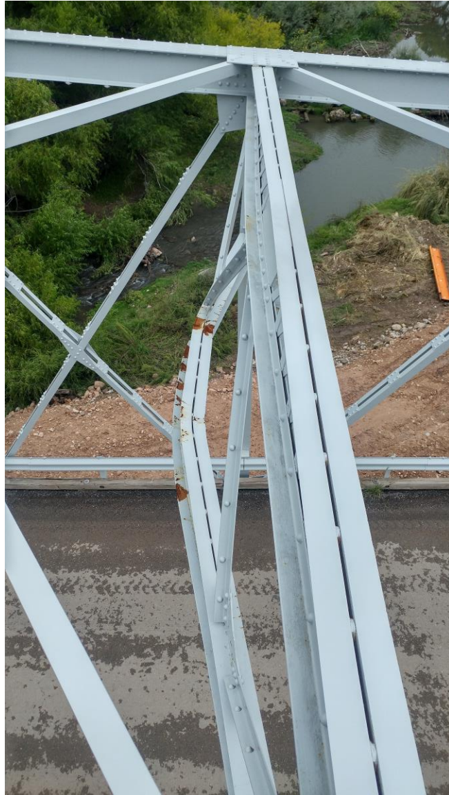
Bridge before repairs showing bracing damage.
