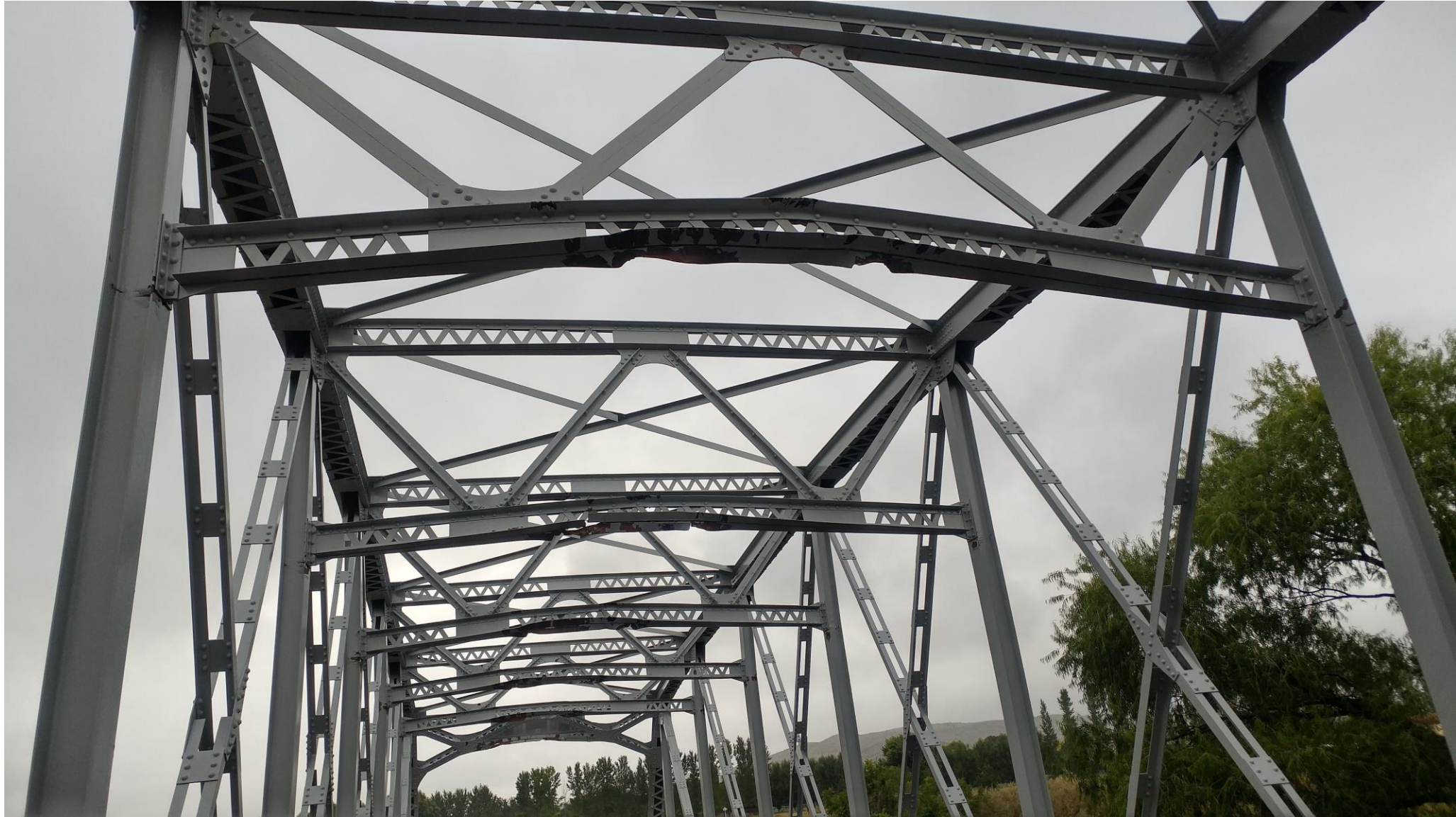
Bridge before repairs showing bracing damage.
