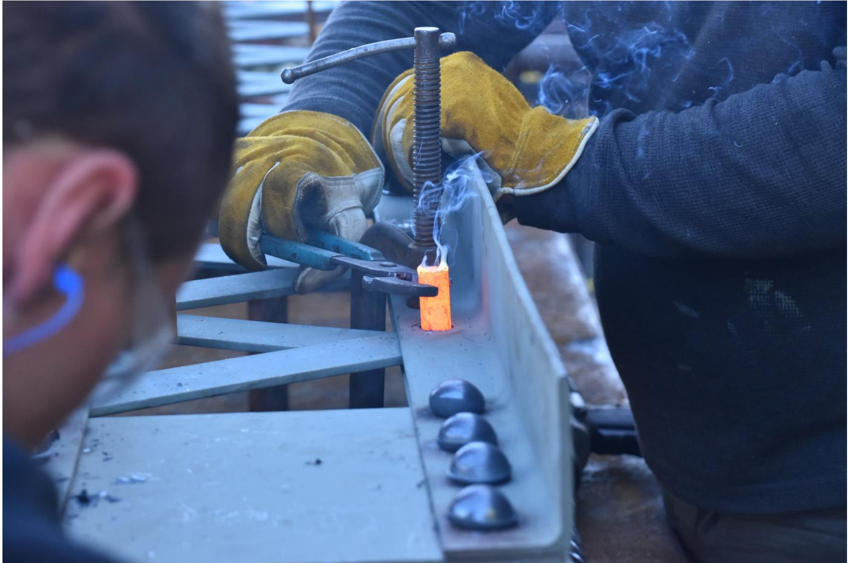
Hot riveting sway bracing.
