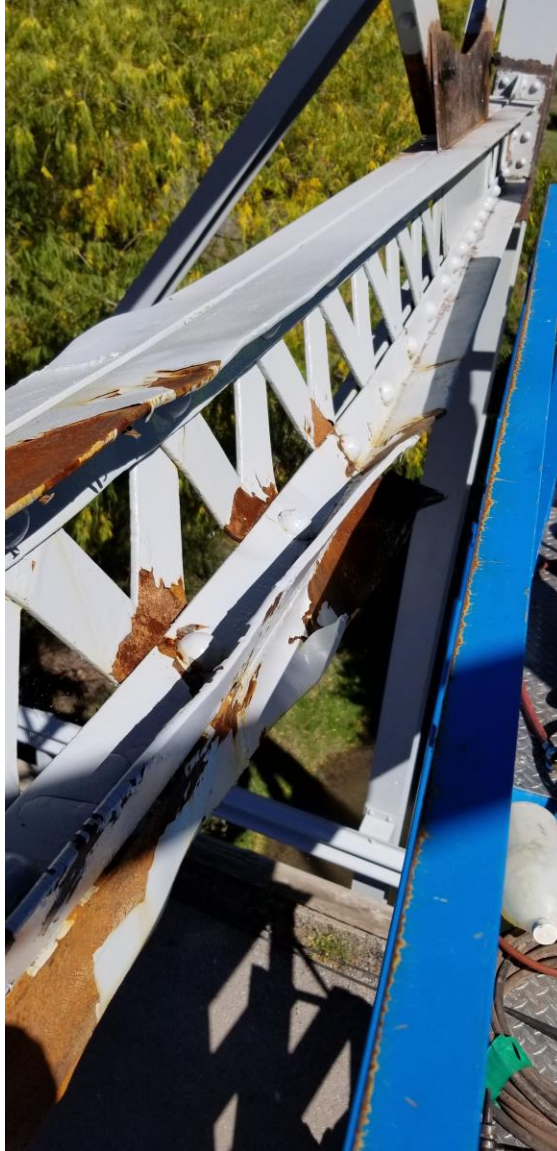
Bridge before repairs showing bracing damage.
