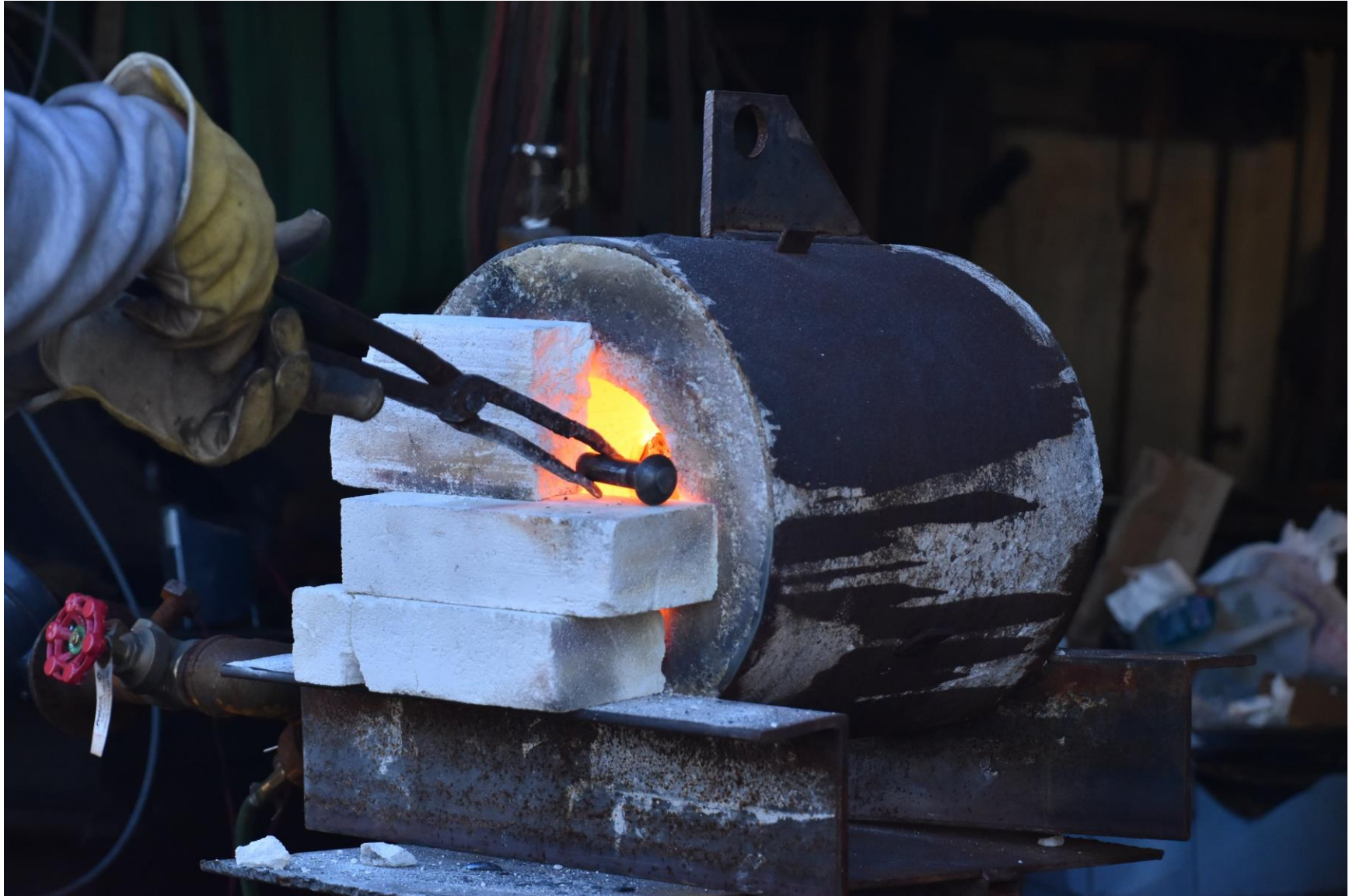
Hot riveting sway bracing.
