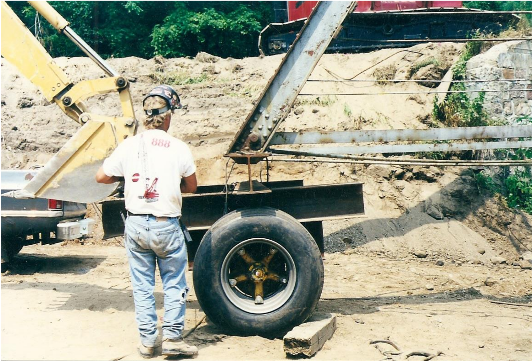
Detail showing the dolly system used to roll the bridge away from the abutments.
