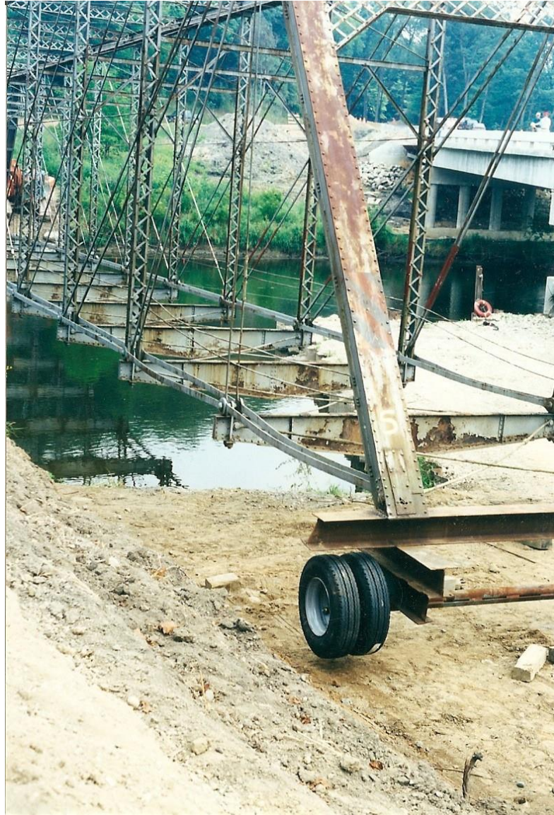
Detail showing the dolly system used to roll the bridge away from the abutments.
