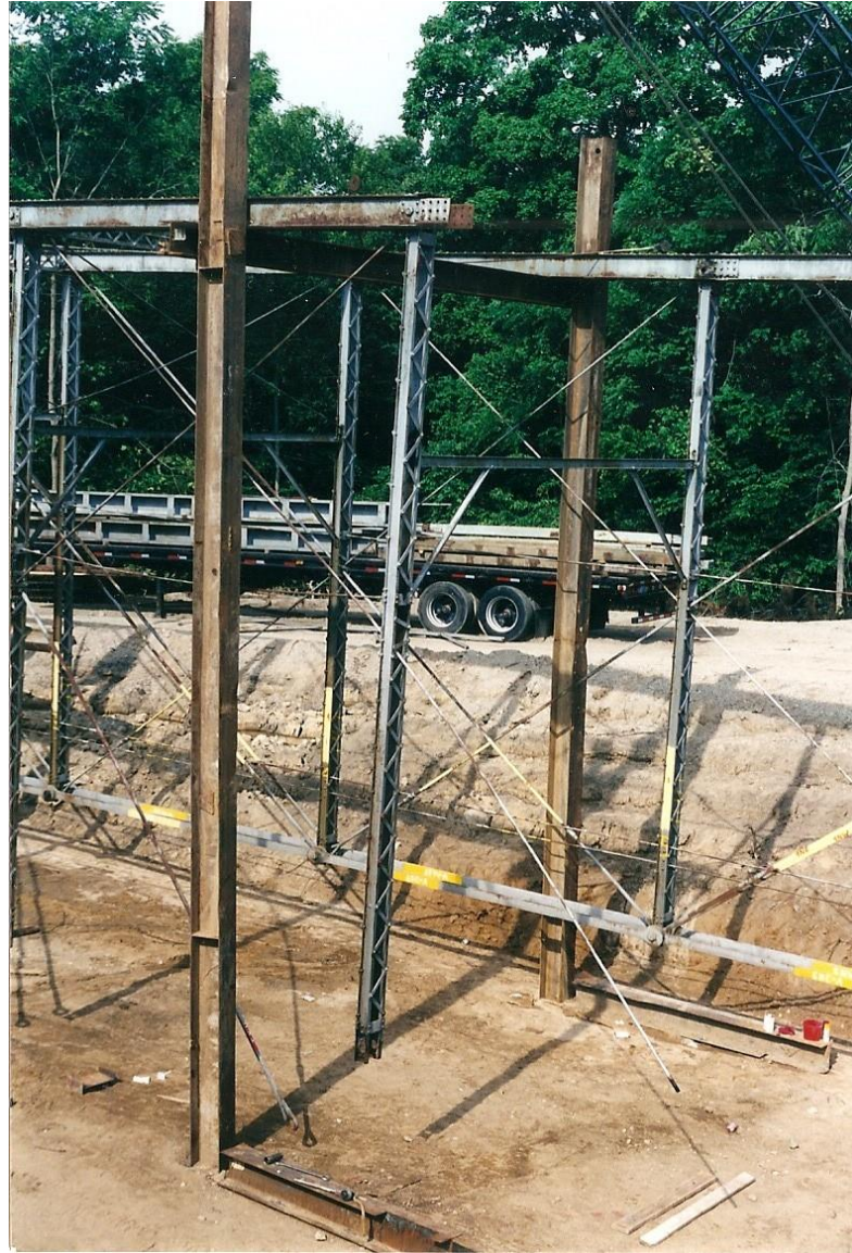
Dismantling the bridge. Note the temporary beams under the top chord and beside the truss added for stability.
