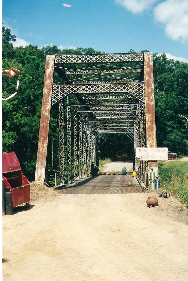
Bridge during deck removal.
