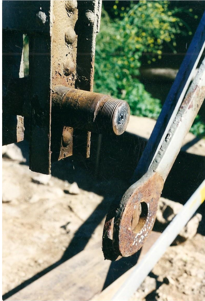
Dismantling the bridge. Detail showing a pin nut removed, as well as the associated eye bars.
