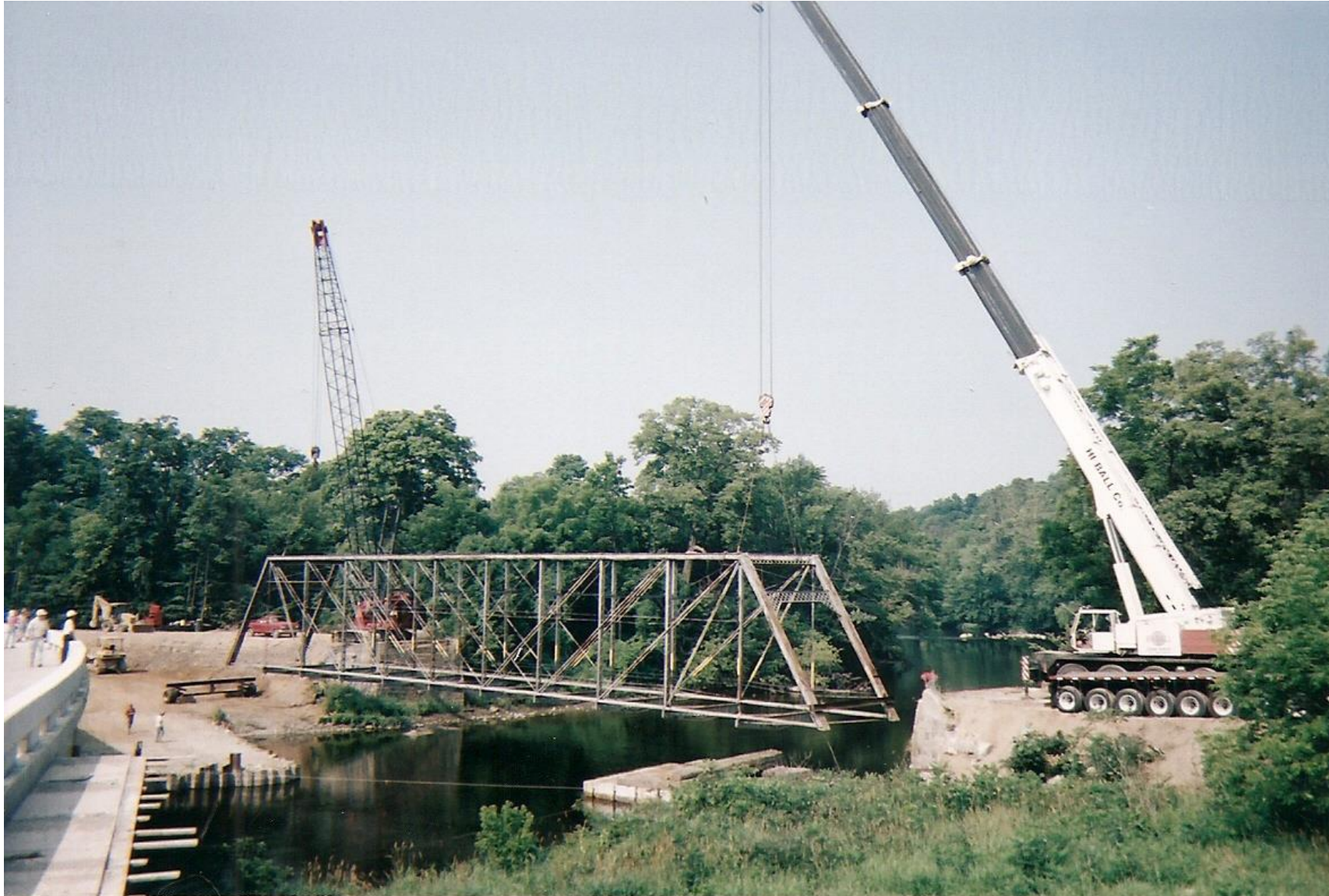
Using two cranes to lift the bridge from its abutments.
