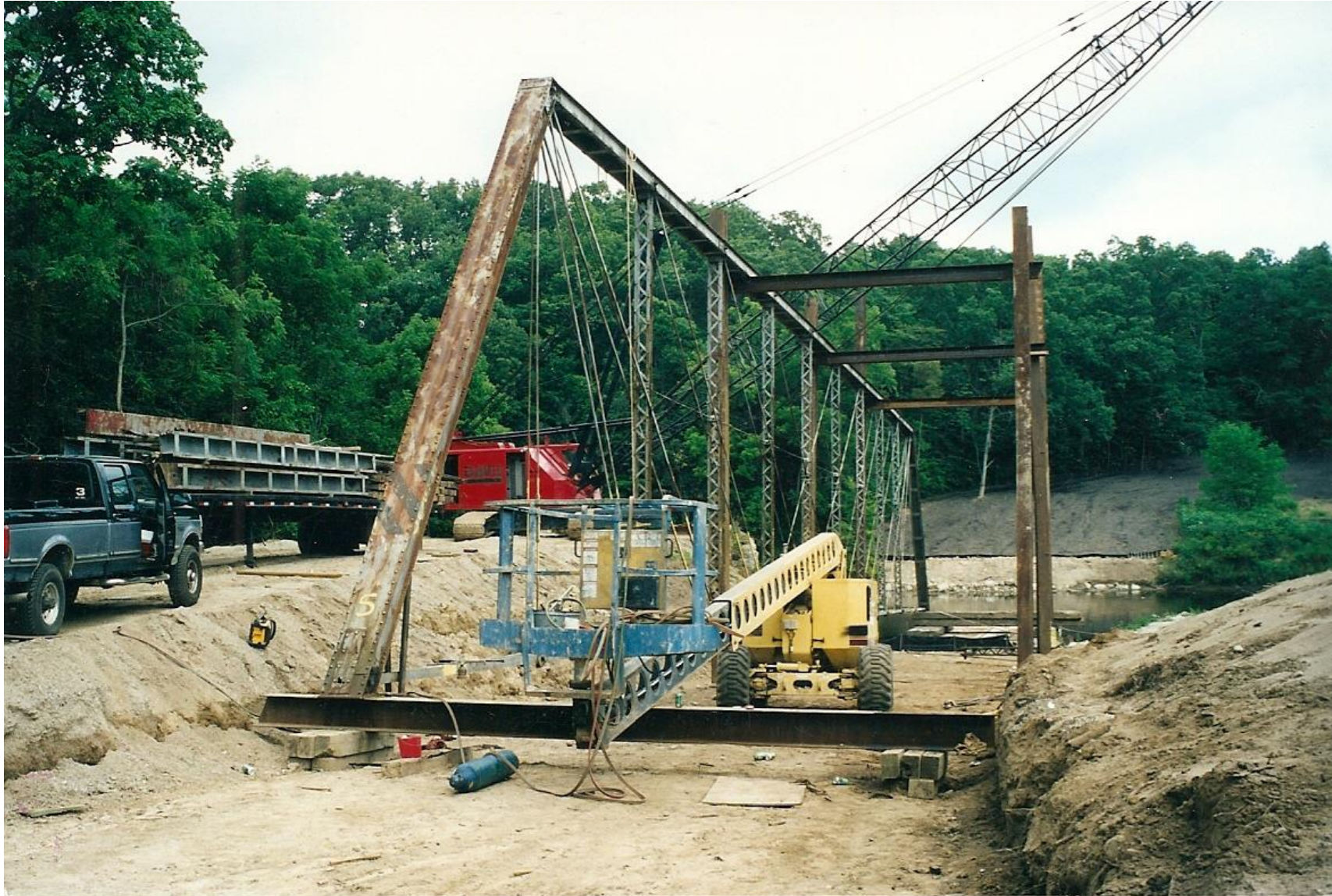
Dismantling the bridge. Note the temporary beams under the top chord and beside the truss added for stability.
