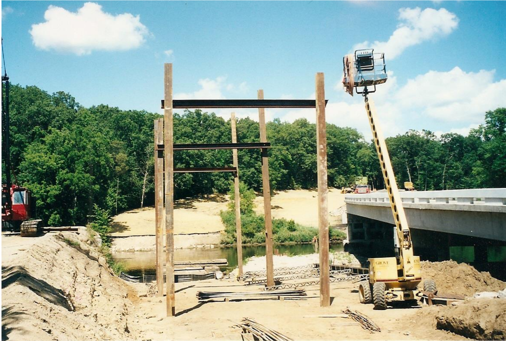
Dismantling the bridge. Bridge completely on the ground, with temporary beams ready to be removed. Photo Courtesy Vern Mesler
