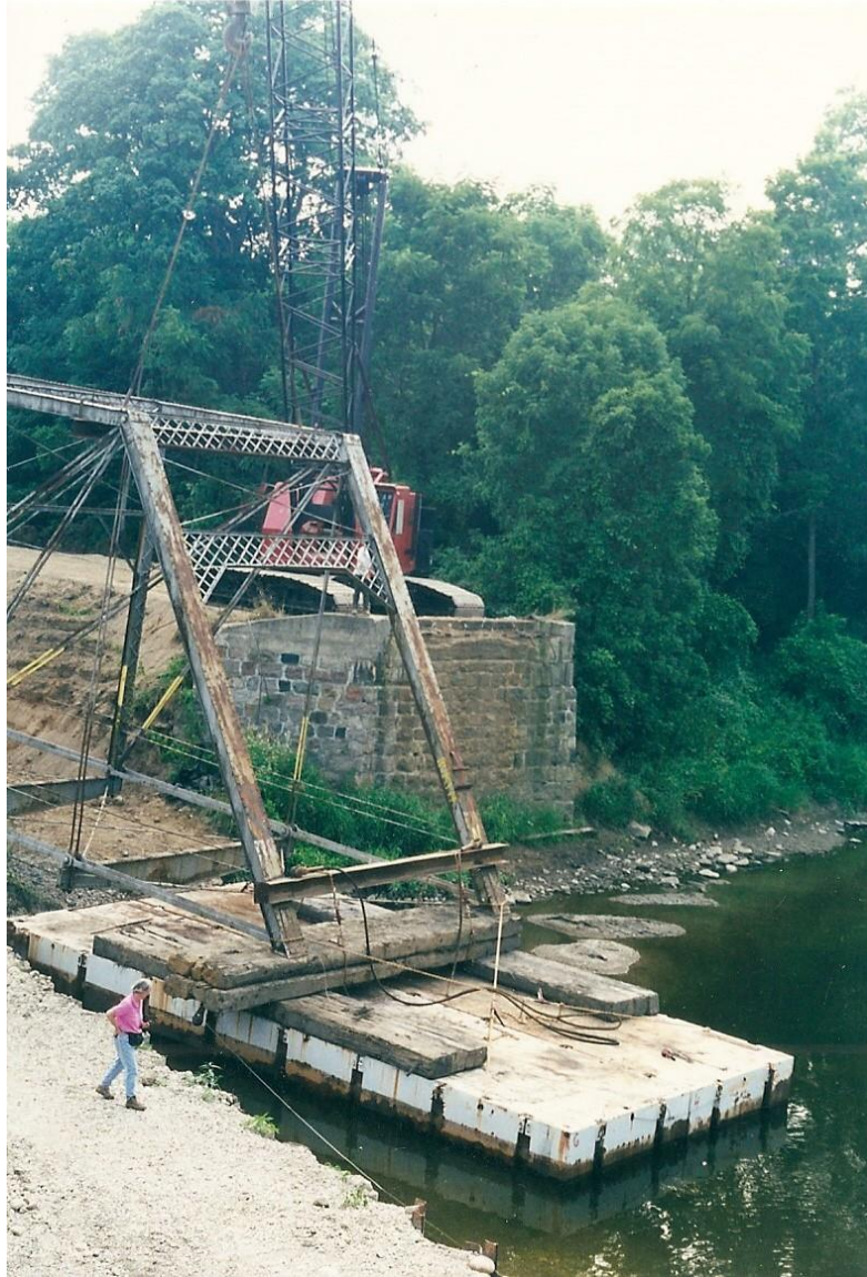
For this particular bridge, a barge was used on the other end for a portion of the removal process.
