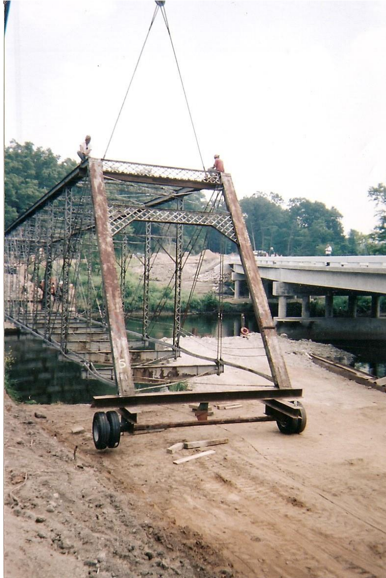
Placing one end of the bridge on a dolly which will roll the bridge back.
