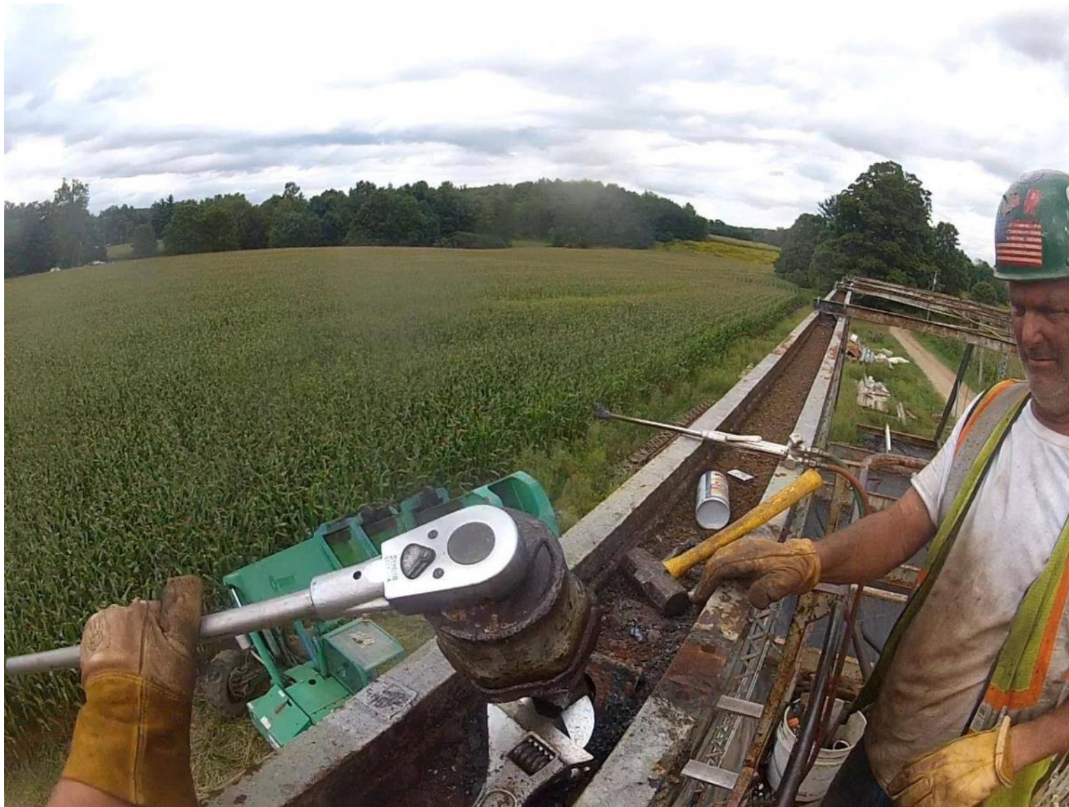
Removing the nut from a diagonal member.
