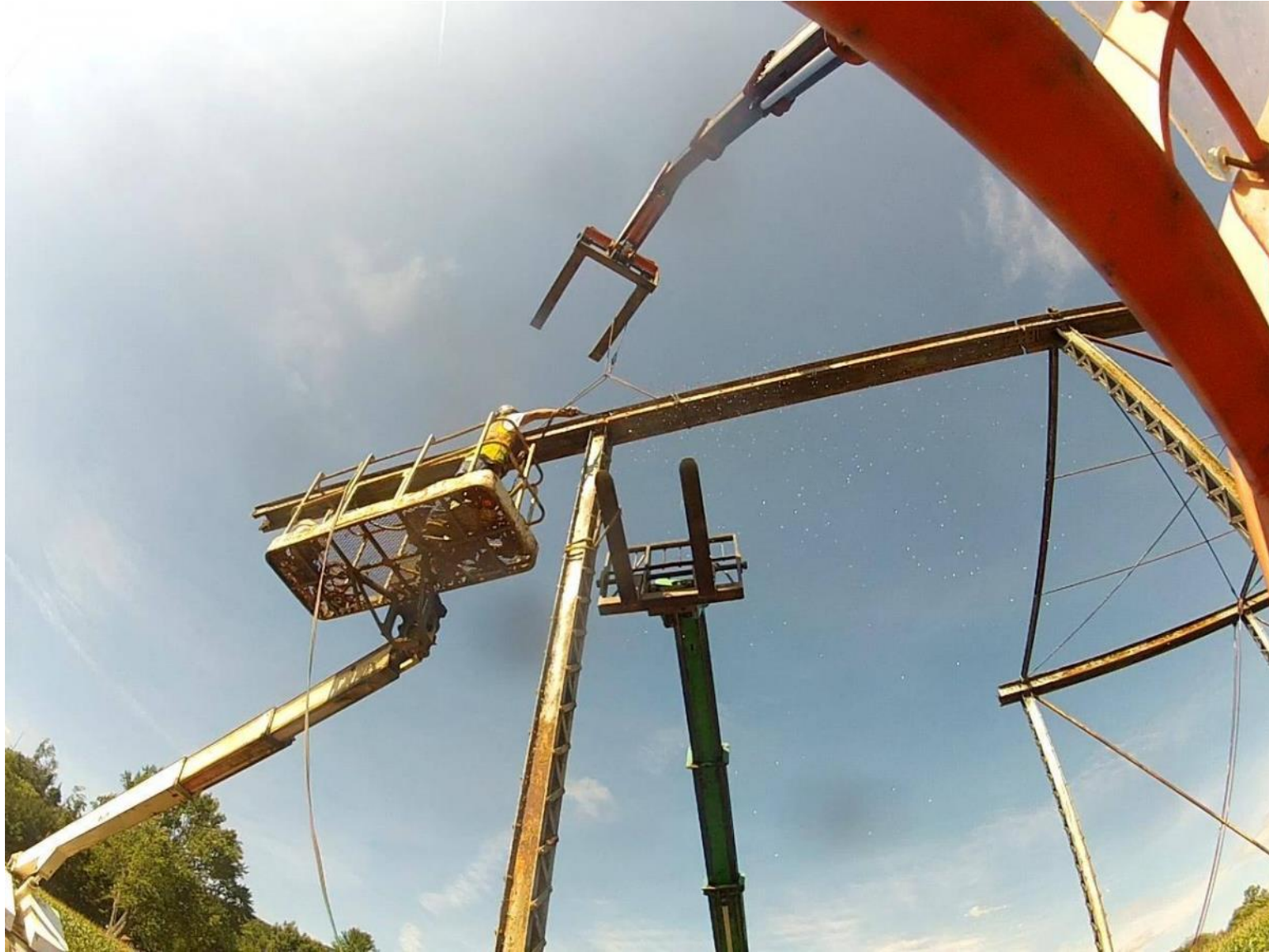
Preparing to remove a top chord section.
