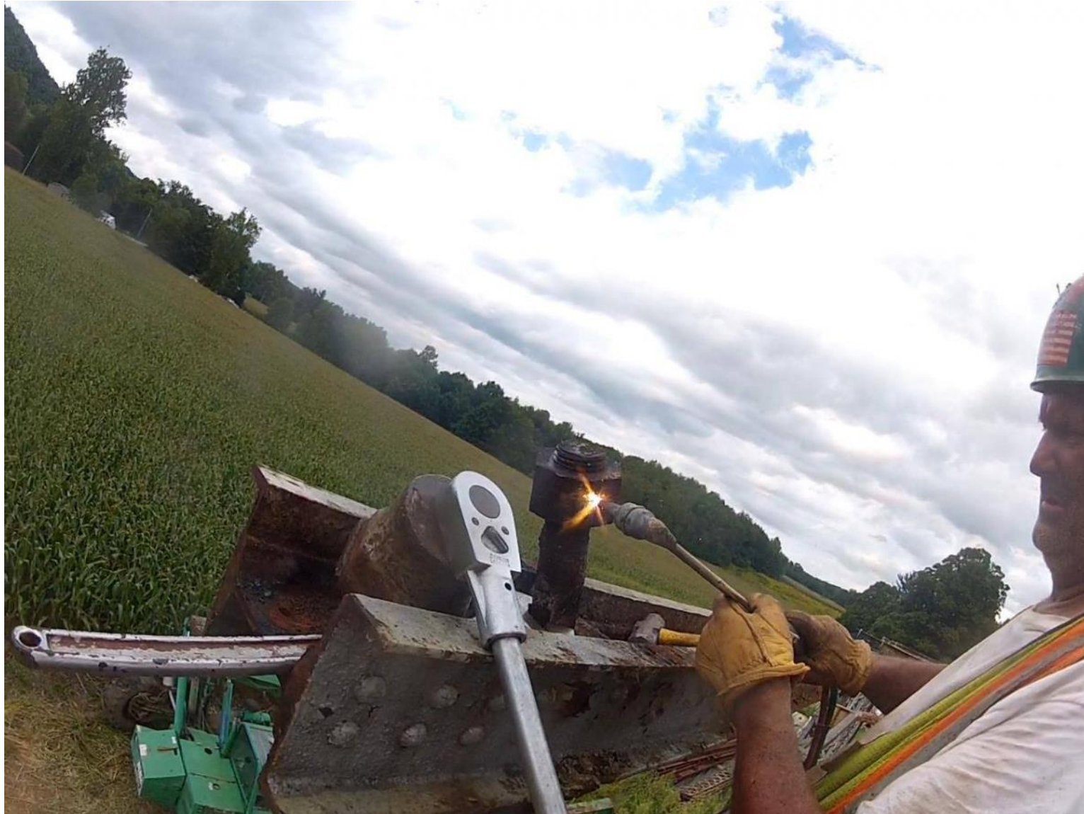
Heating up a diagonal member nut to facilitate removal.
