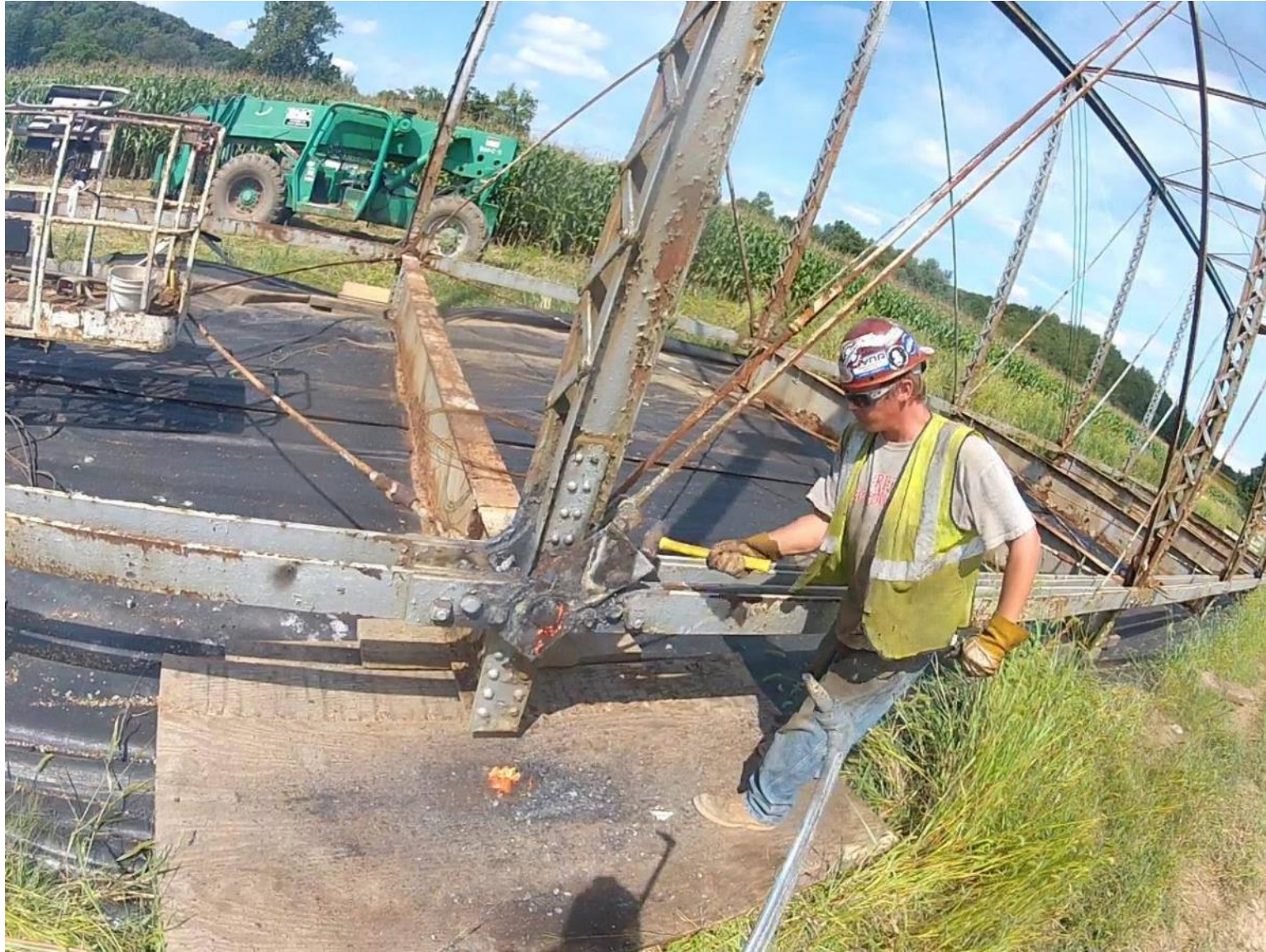
Removing an added non-original welded plate at the bottom chord connection.
