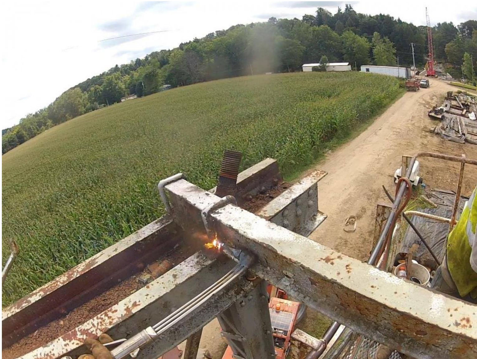
Removing a strut.
