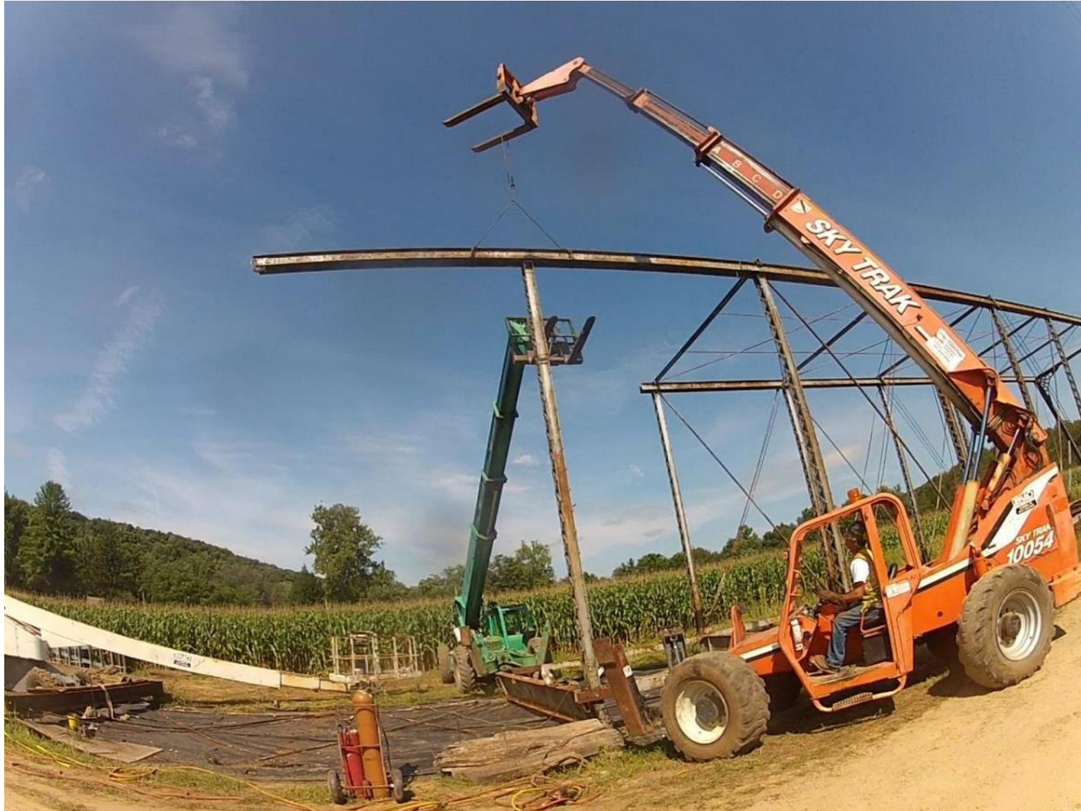
Preparing to remove a top chord section.
