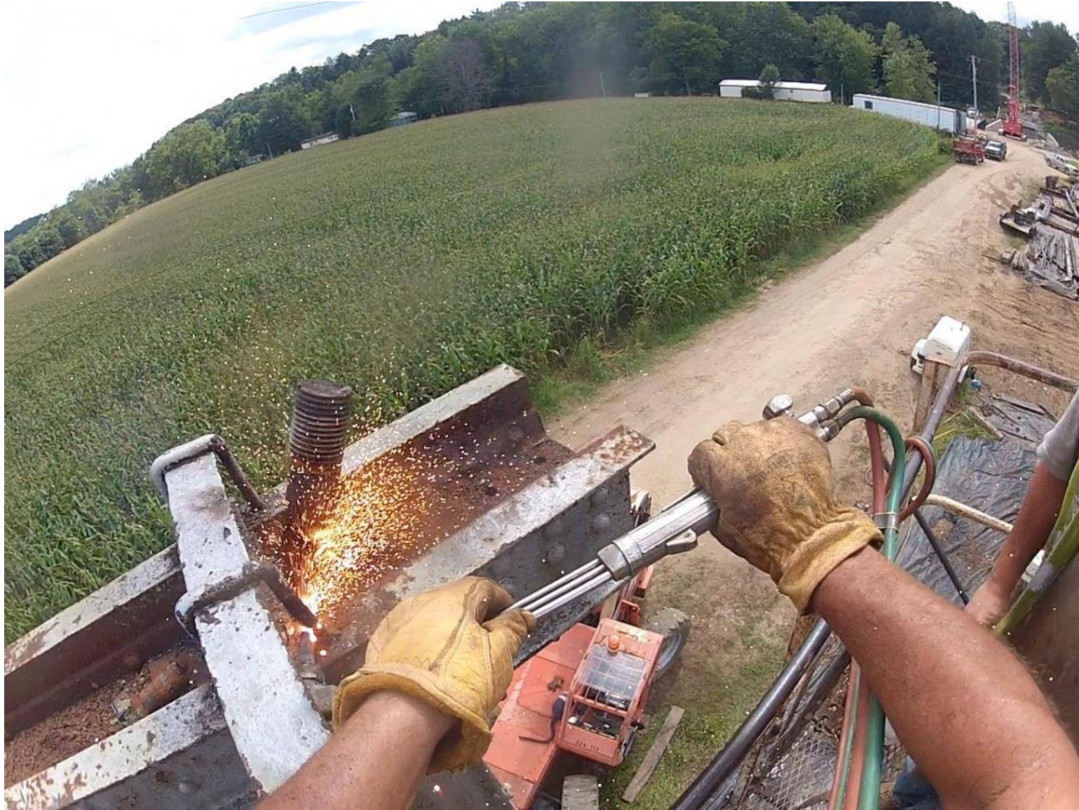
Removing a strut.
