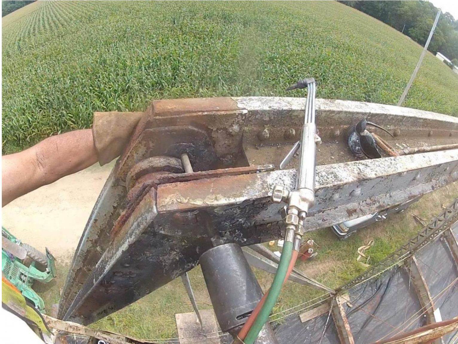
Driving the remains of a pin out of the top chord.
