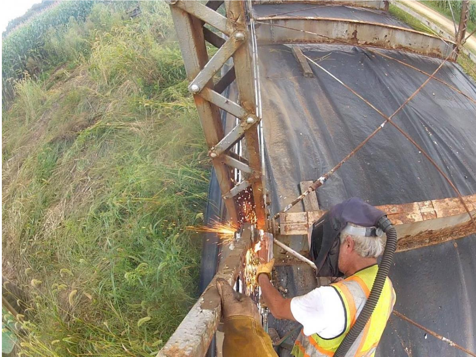
Removing diagonal.
