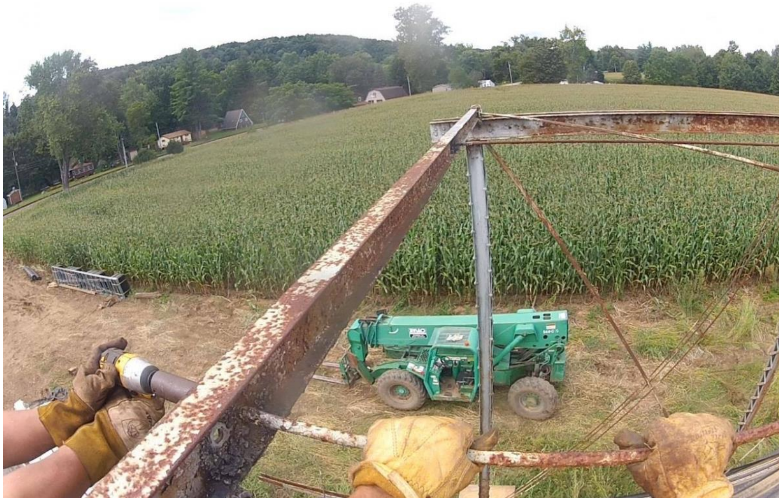
Removing bracing.
