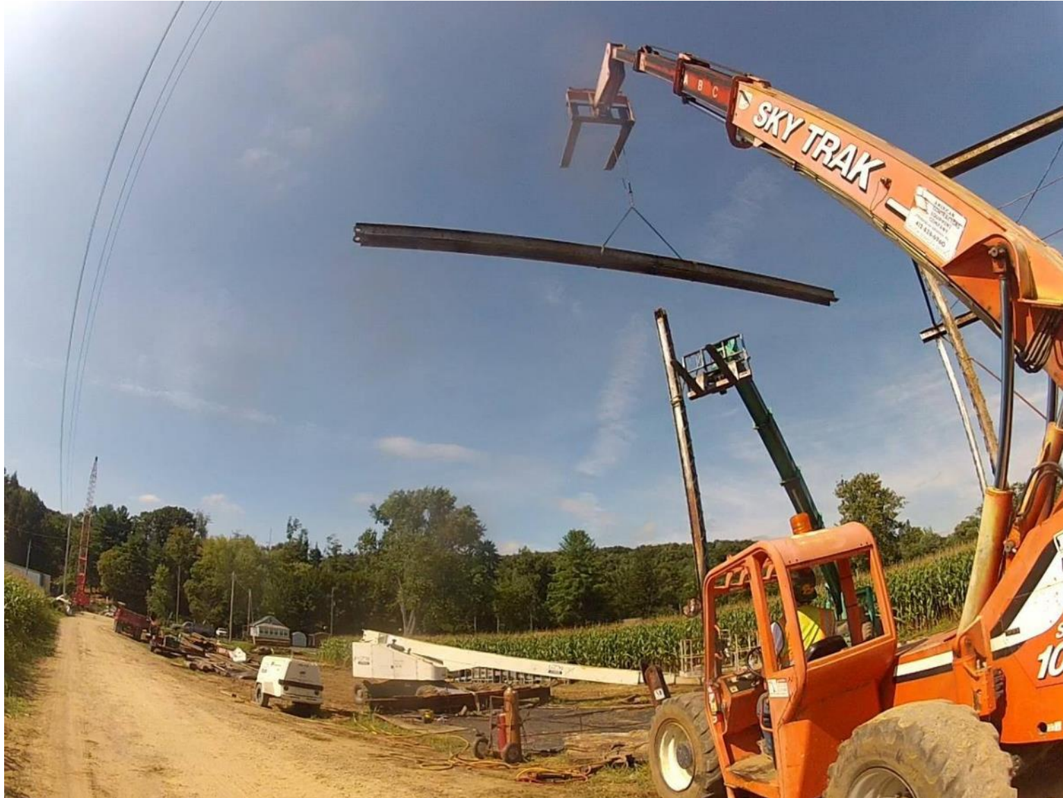
A top chord section is lowered to the ground.
