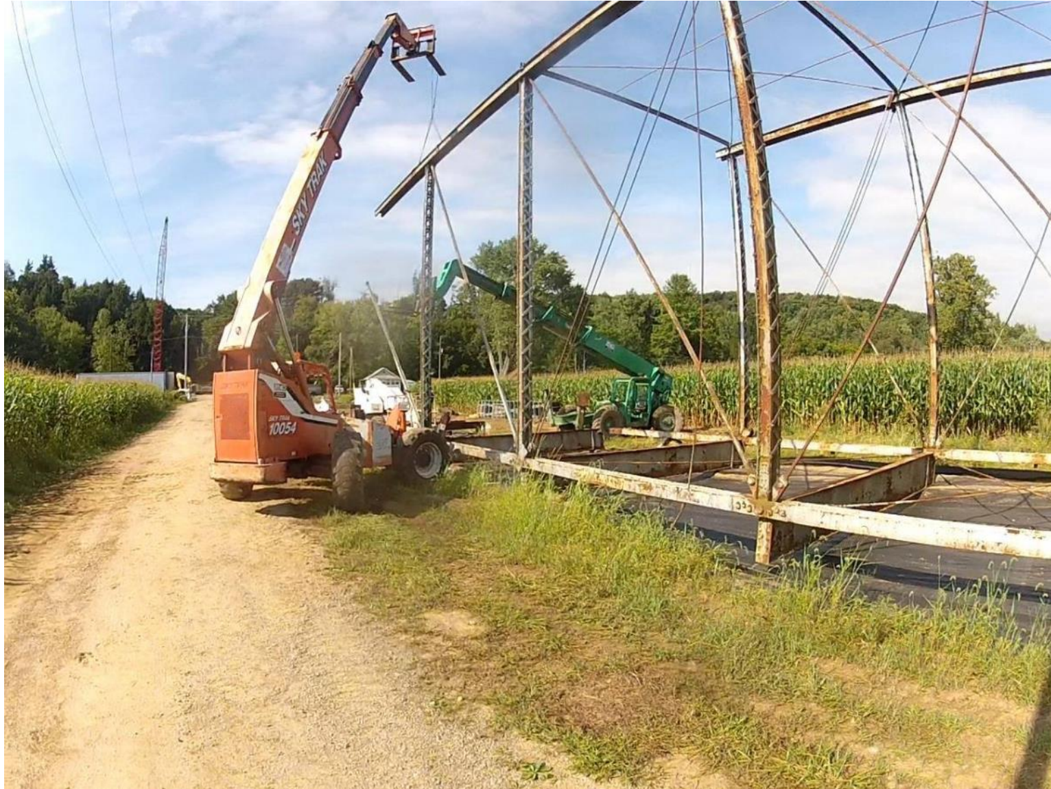
Preparing to remove a top chord section.
