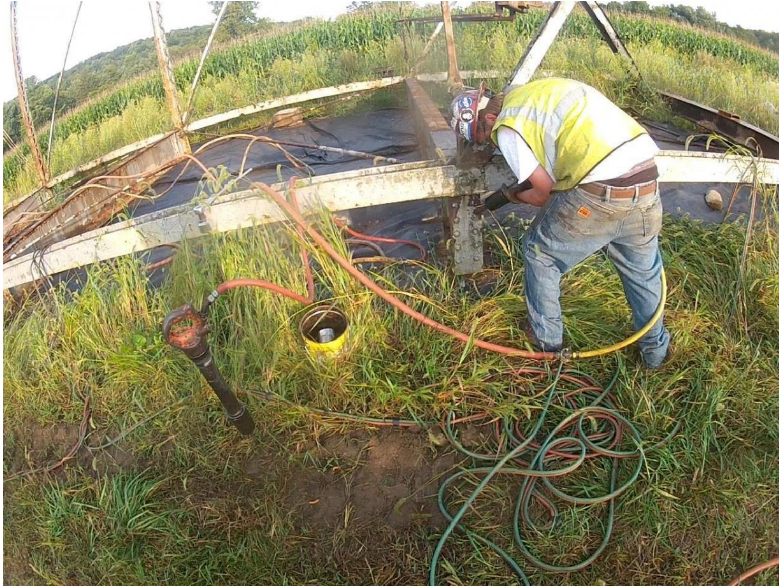
Using a rivet buster to remove rivets from a pin plate.
