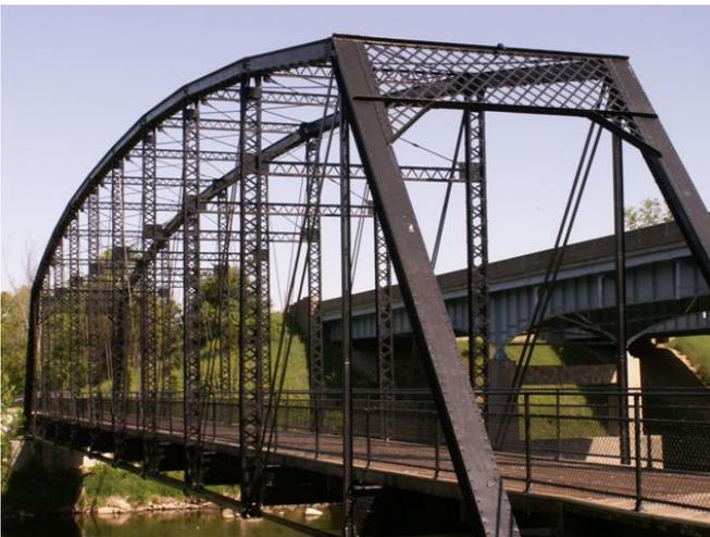
**Kent Street Bridge in Portland, Michigan** – Restored, reassembled, and reinstalled this large 220 foot through truss span in a new location over the Grand River for pedestrian use on Portland's trail system. The restored bridge is pictured to the left. Due to the size of the bridge and restrictions on the type of work that could be performed in the water, a special tramway system was designed to erect and deploy the bridge over the river in sections.
