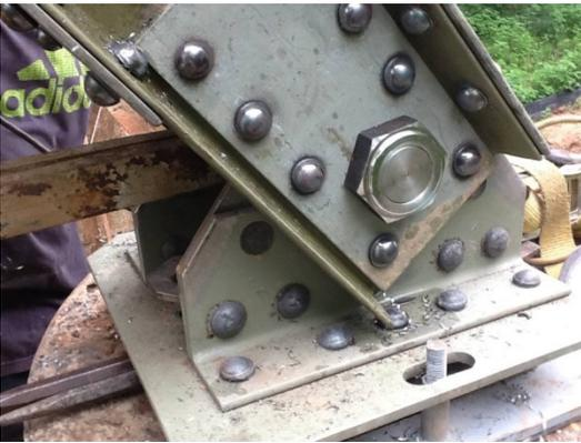
**Wildcat Bridge Road Bridge, Robertson County, Texas** – Bach Steel rehabilitated this bridge for vehicular use. A photo showing a replicated end post base and bearing for this bridge with newly driven rivets visible is shown to the left.
