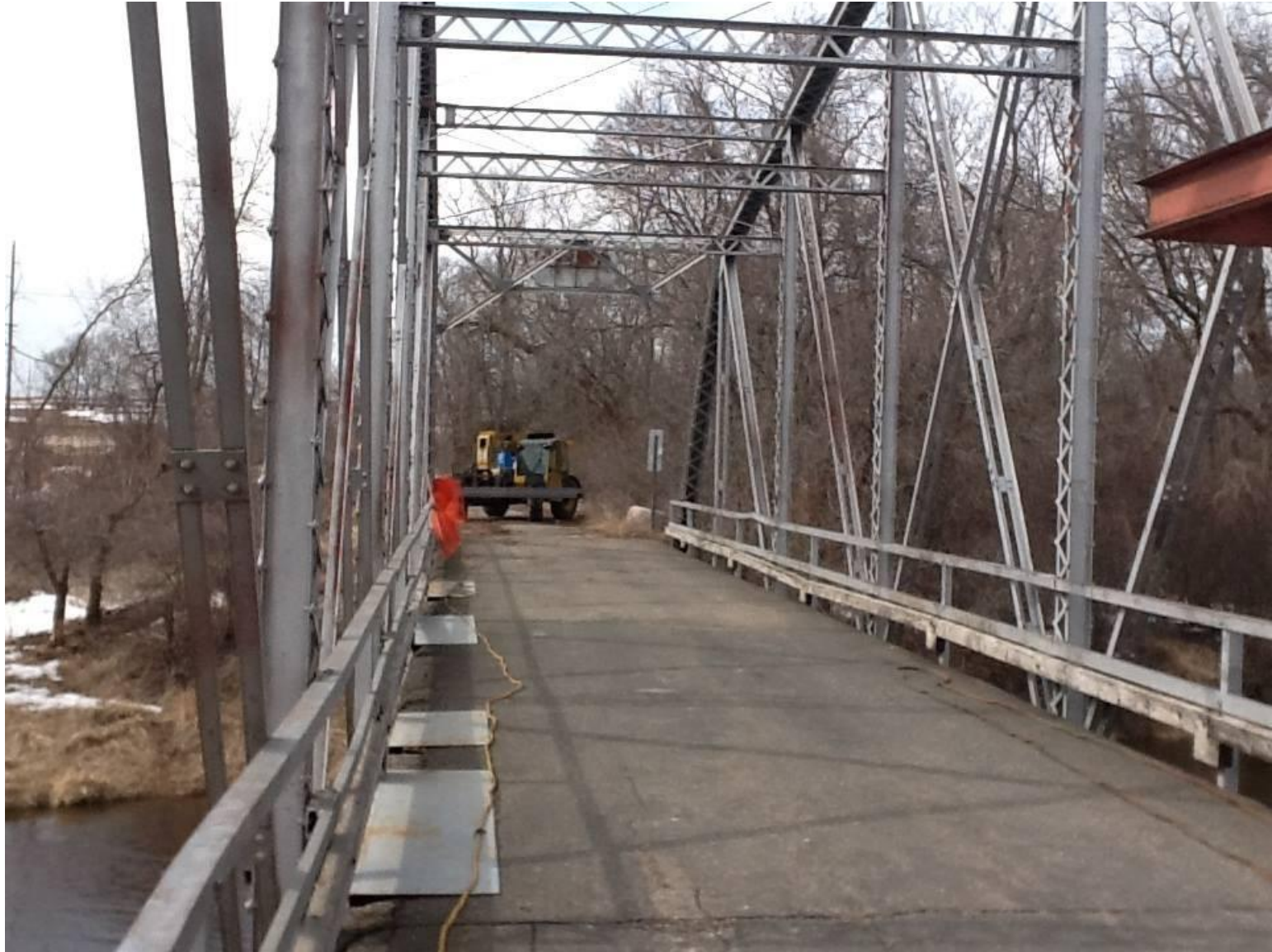
Arrival at the bridge and setting up.
