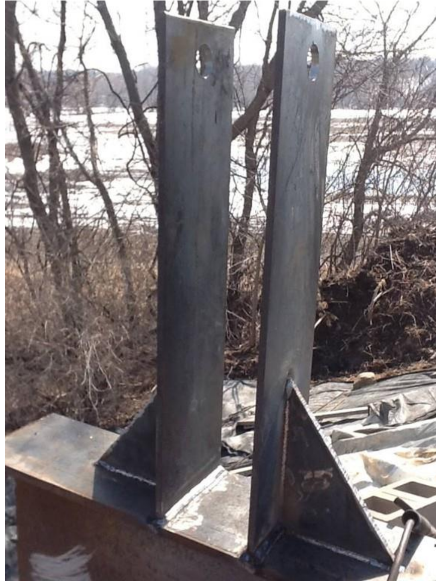
Detail of the temporary beam as fabricated by Bach Steel.
