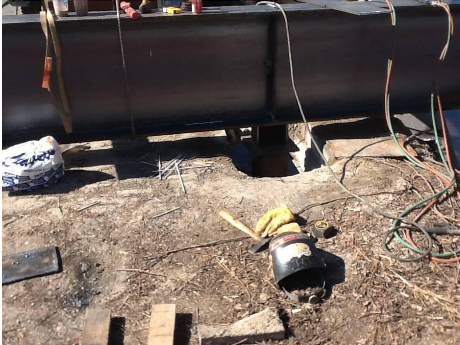
Detail of the temporary beam as fabricated by Bach Steel.
