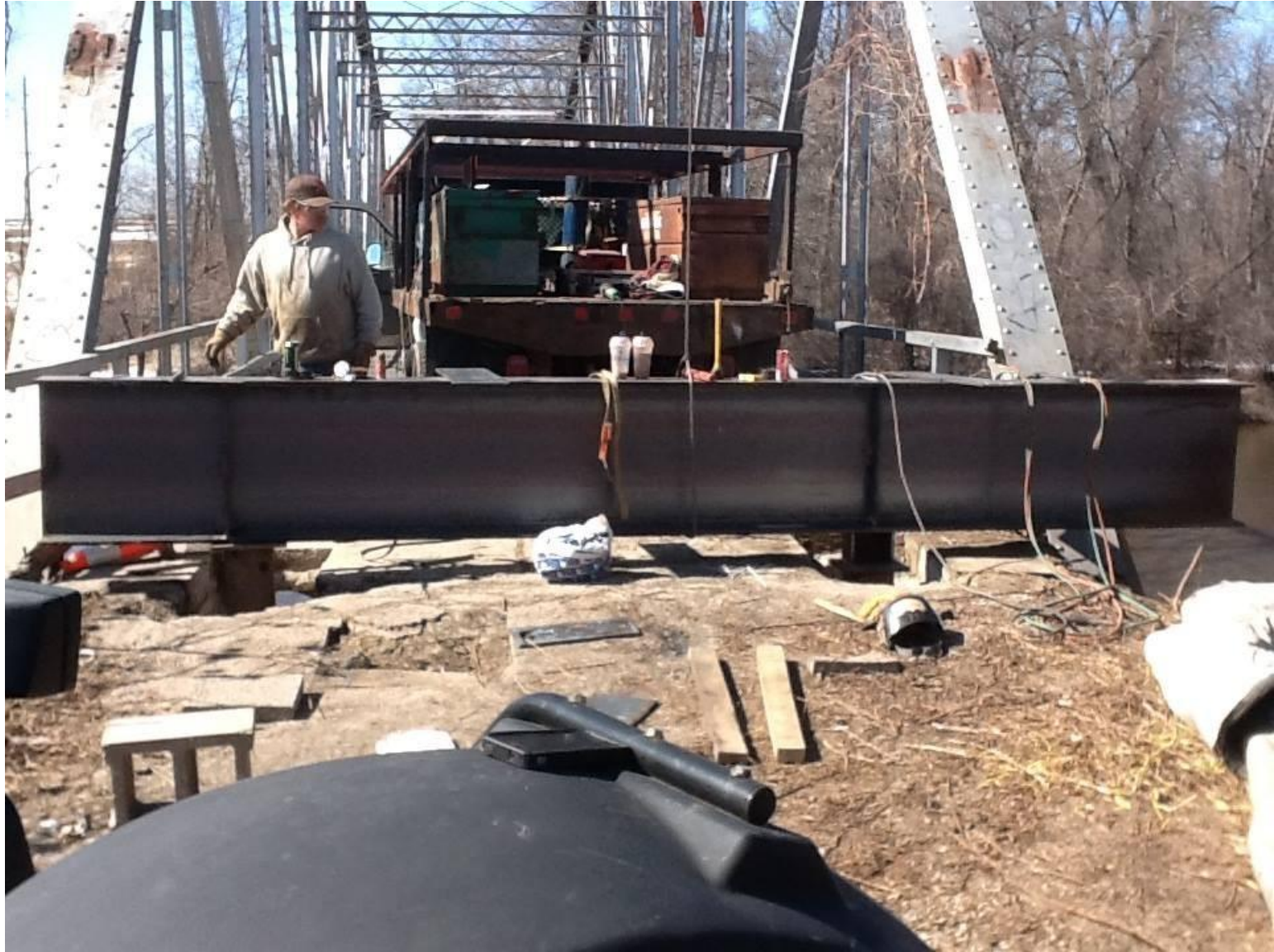
View of the temporary beam as fabricated by Bach Steel.
