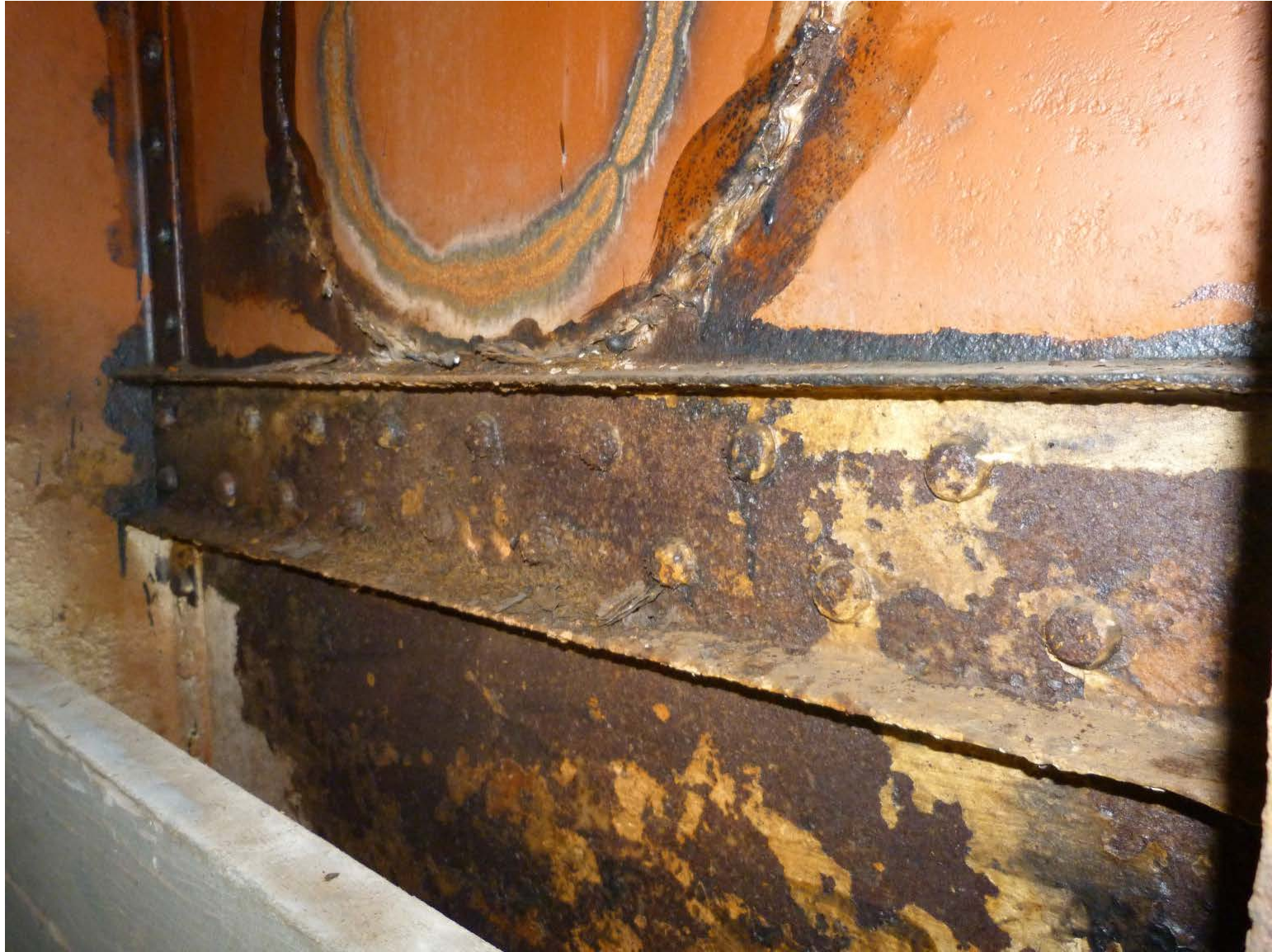
Lighthouse and Catwalks Before Project
