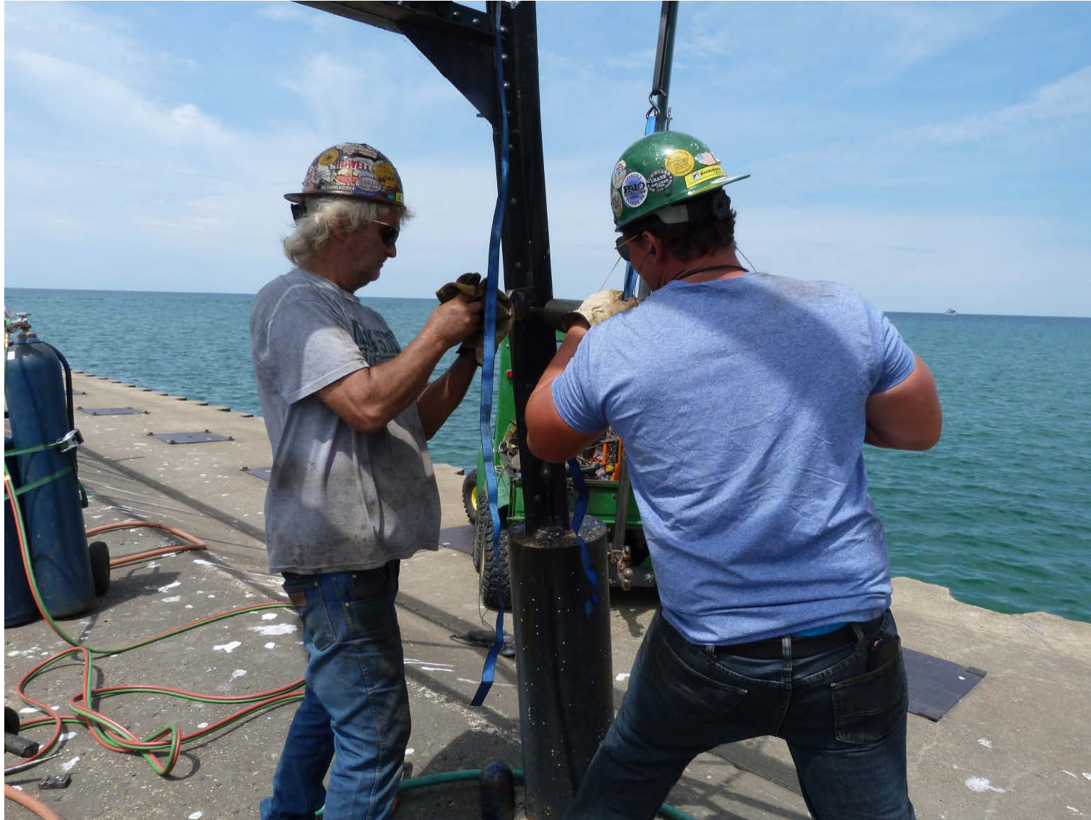
Pack rust removal on catwalks.
