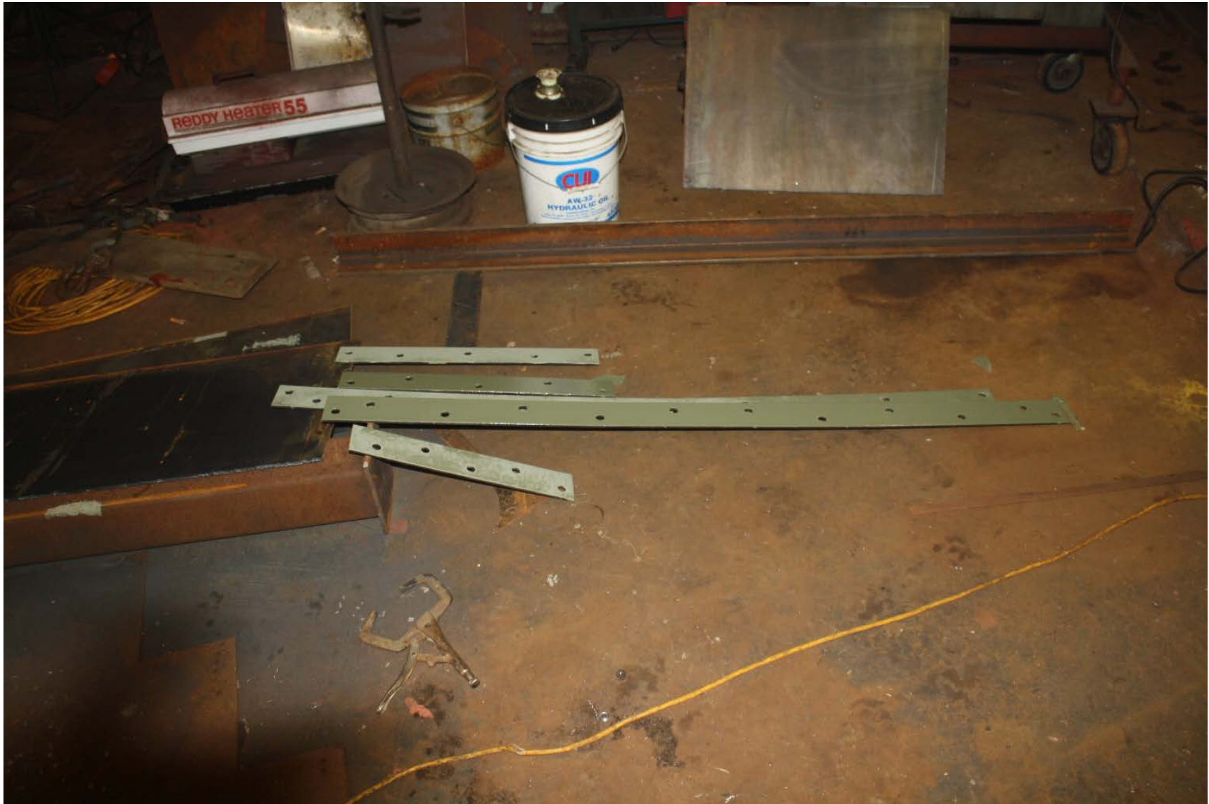
Shop fabrication and riveting of replica doors.
