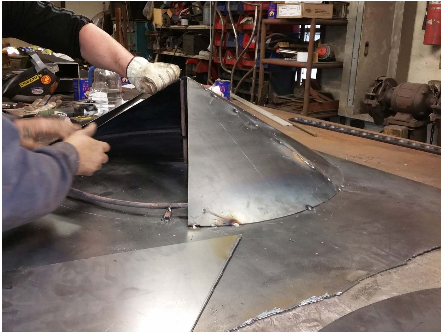
Fabrication of replica chimney cap.
