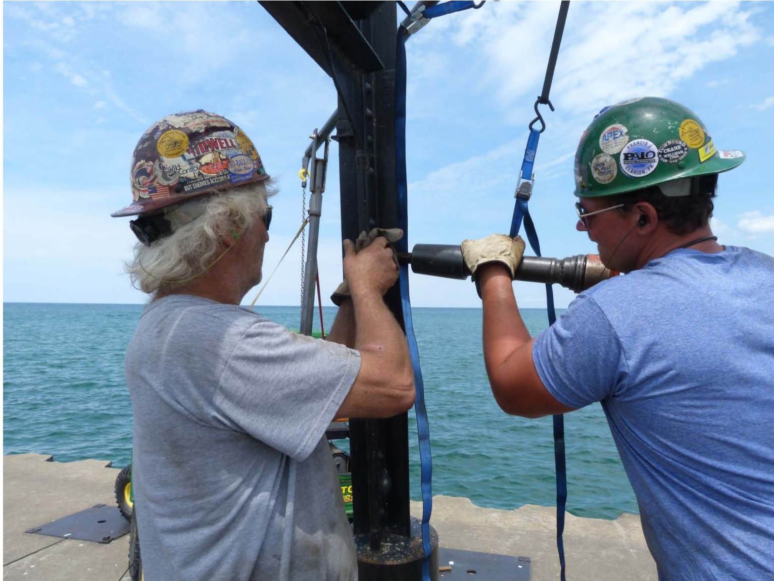
Pack rust removal on catwalks.
