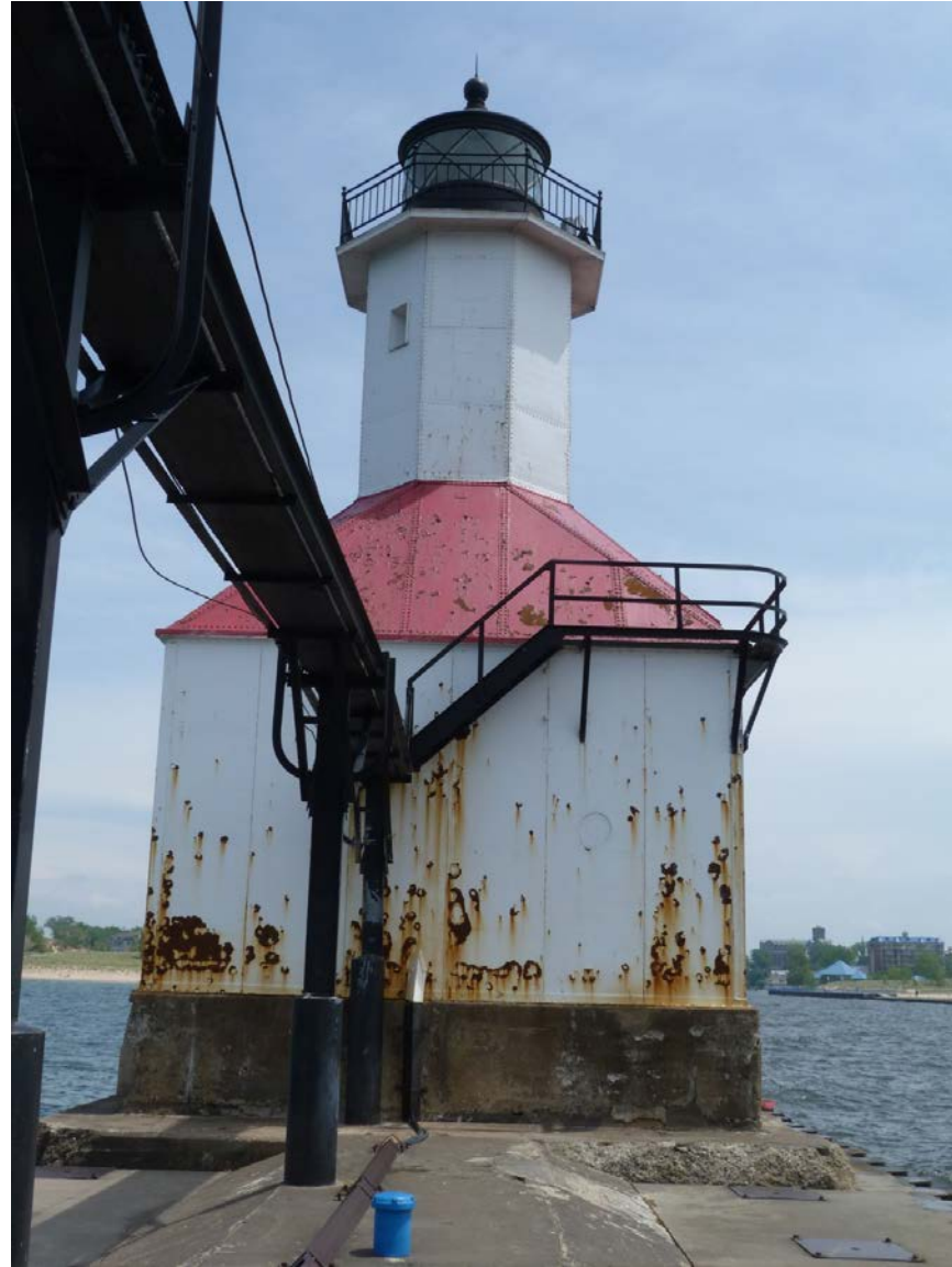
Lighthouse and Catwalks Before Project
