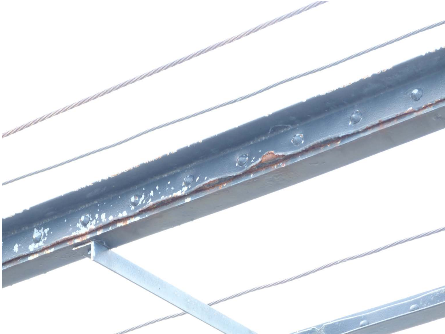
Lighthouse and Catwalks Before Project
