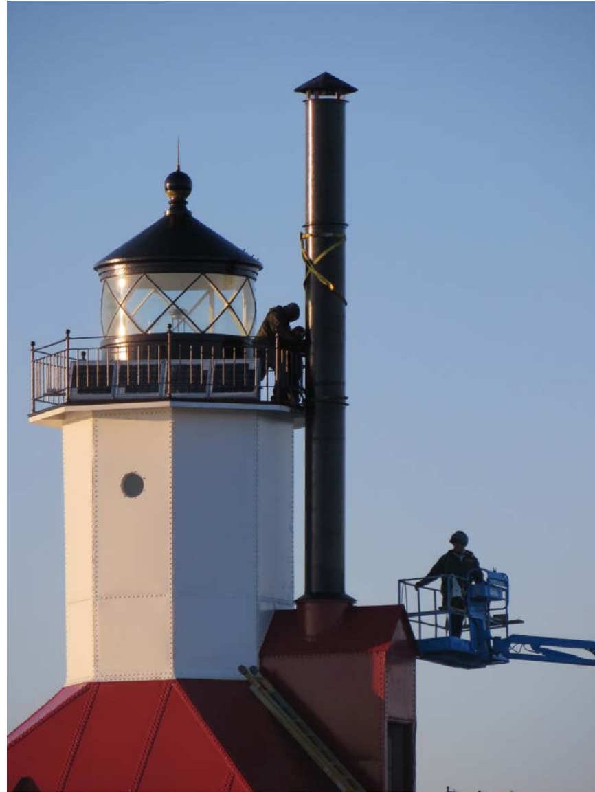
Installation of replica chimney. Lighthouse restoration mostly complete.
