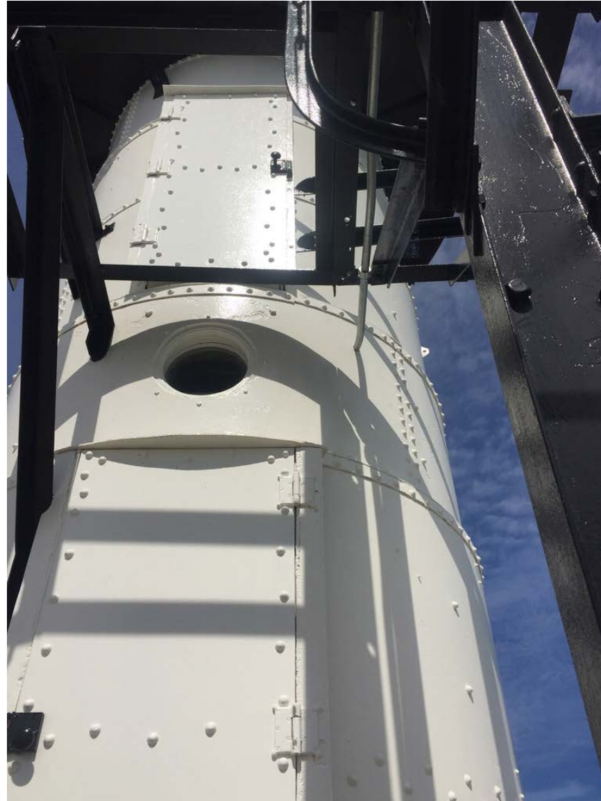
Replicated, hot-riveted doors installed, after painting.
