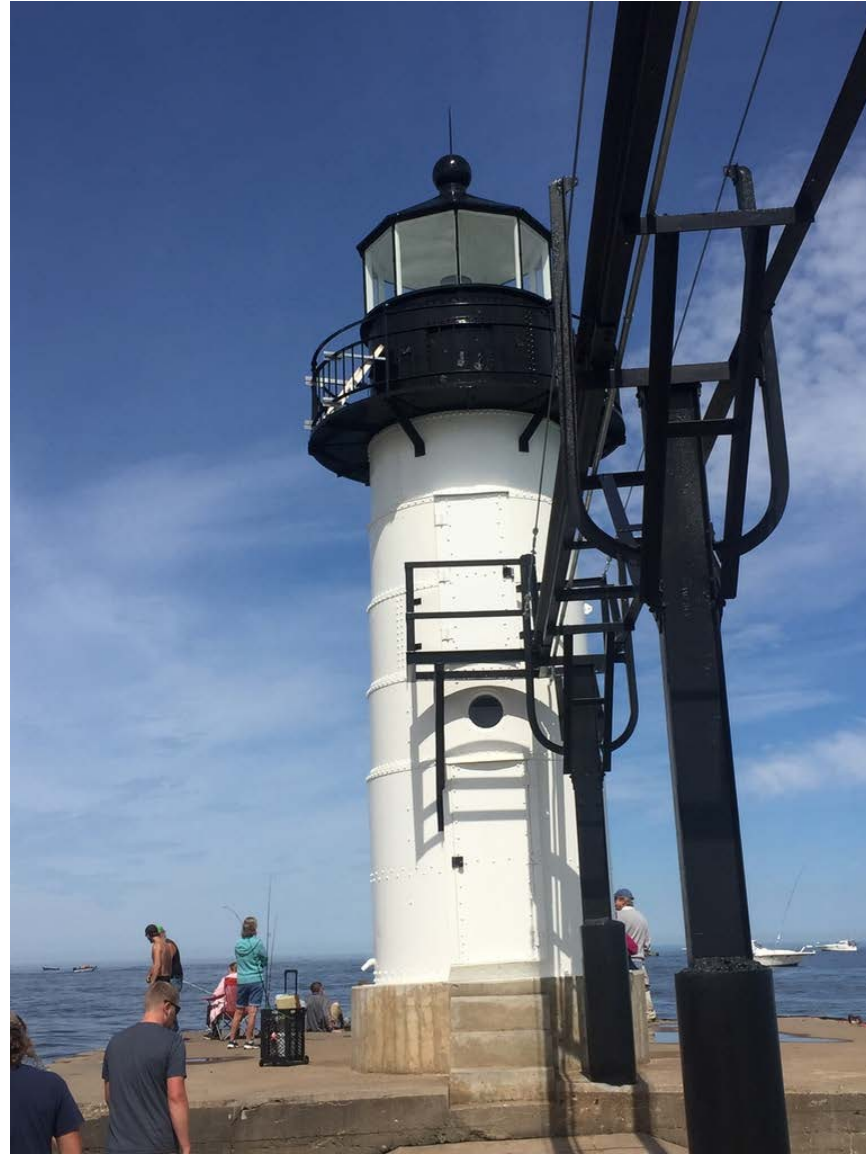
Outer light after restoration.
