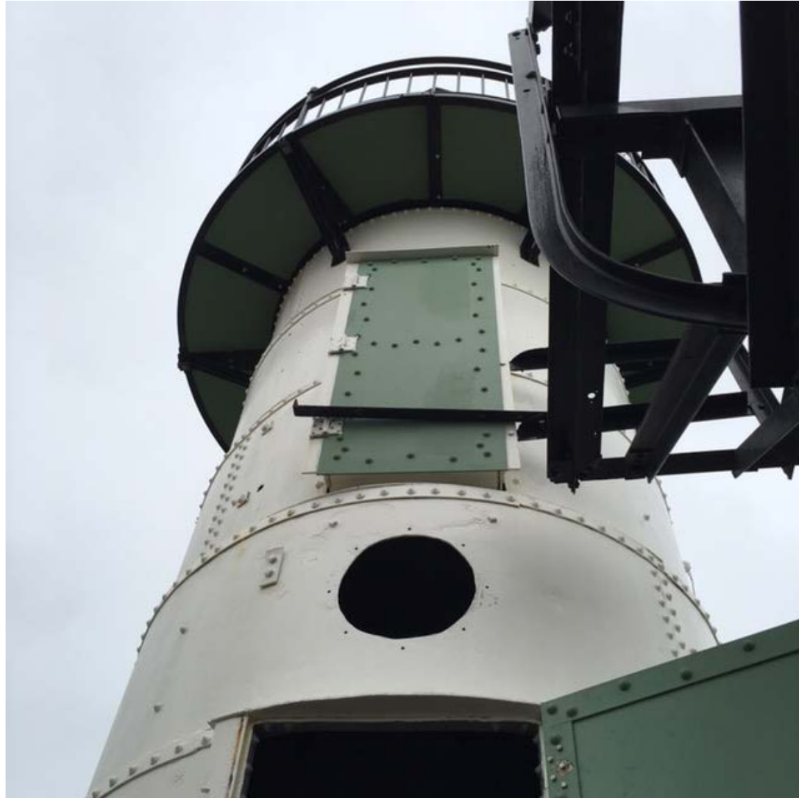
Replicated, hot-riveted doors installed.
