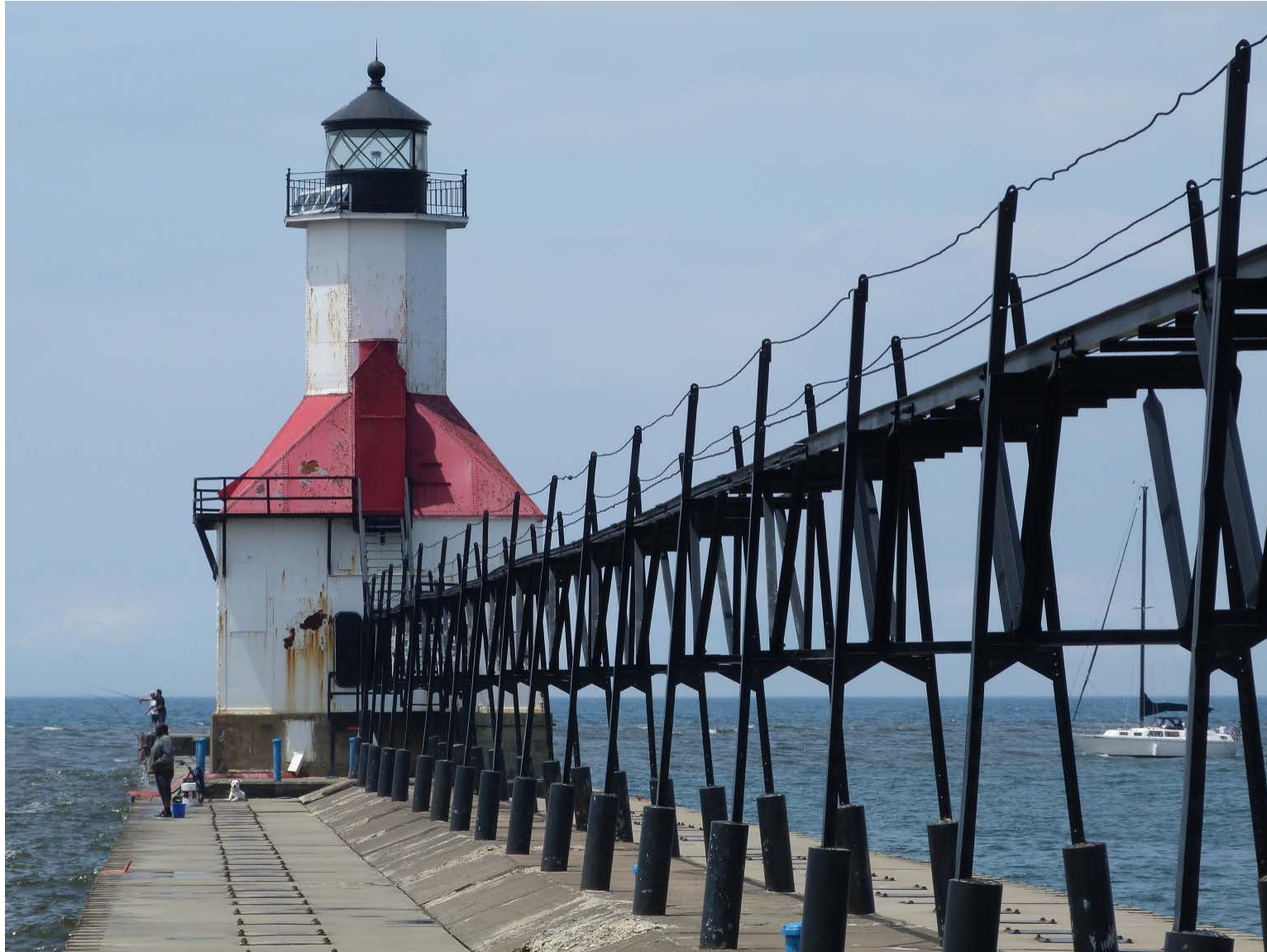
Lighthouse and Catwalks Before Project
