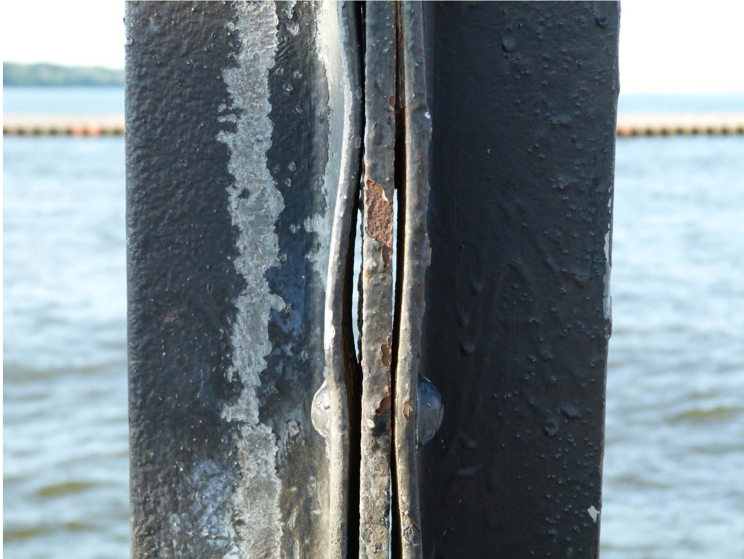
Pack rust removal completed, before bringing the bent plates back together.
