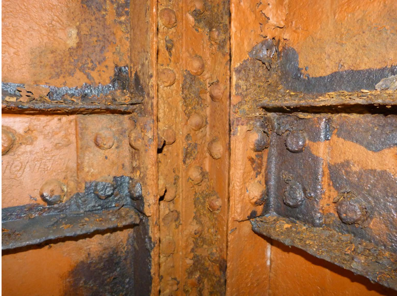
Lighthouse and Catwalks Before Project
