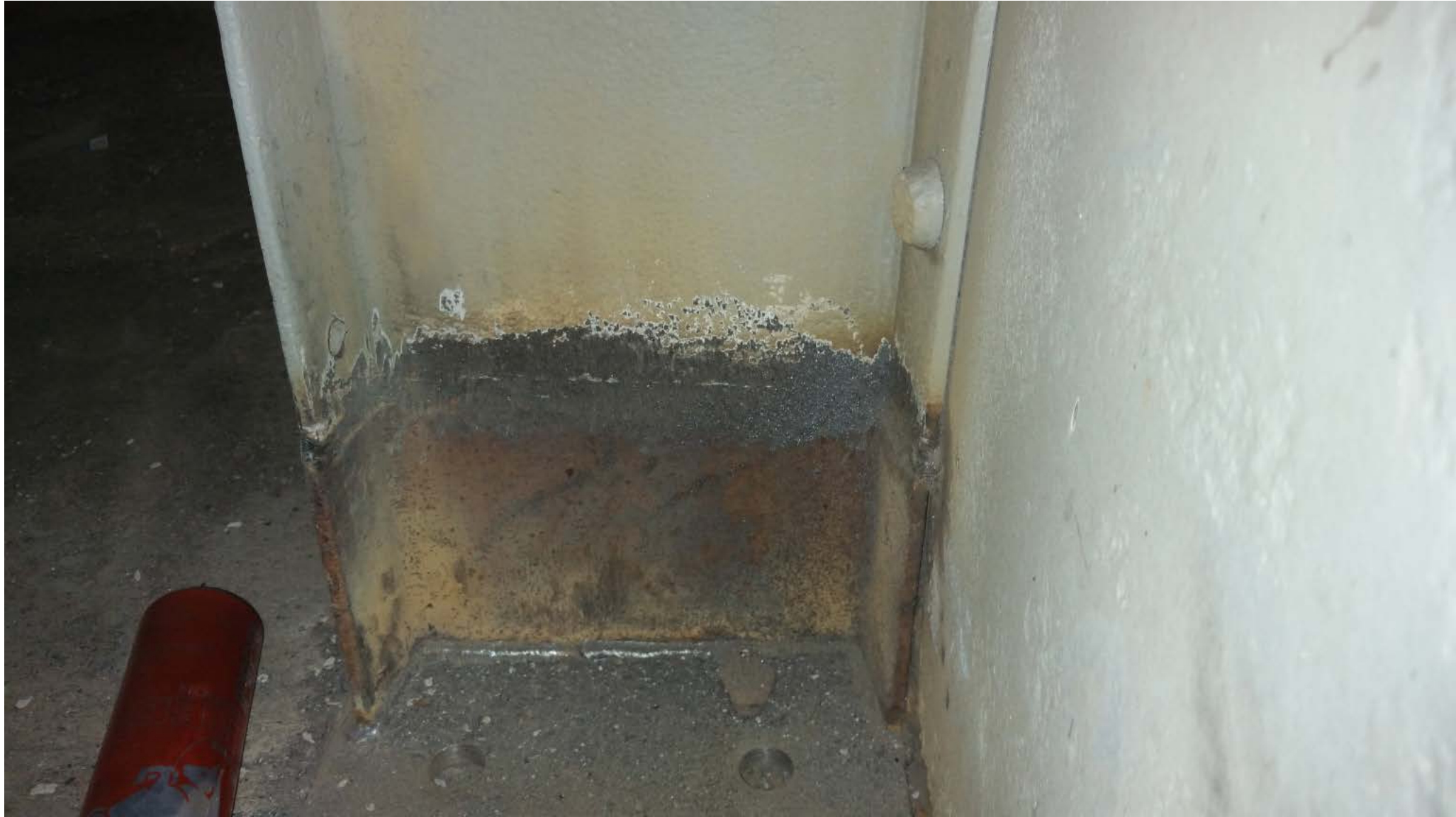
Removing and replacing deteriorated lighthouse structural elements.
