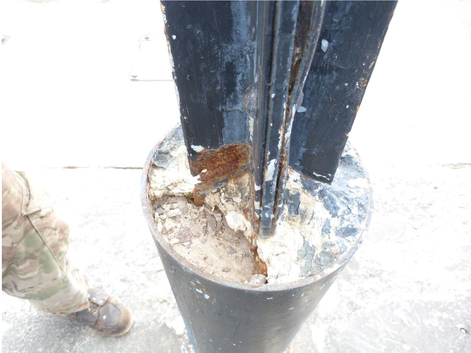
Deteriorated leg prior to work.
