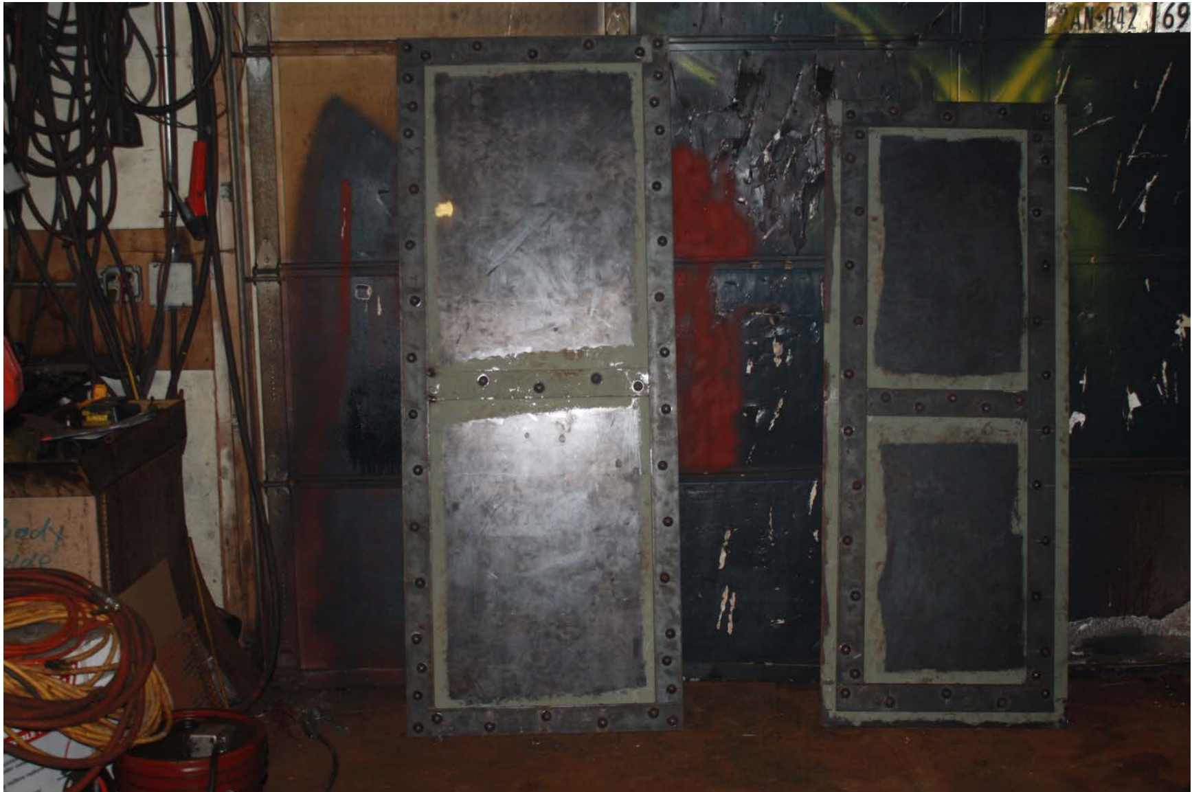
Shop fabrication and riveting of replica doors.
