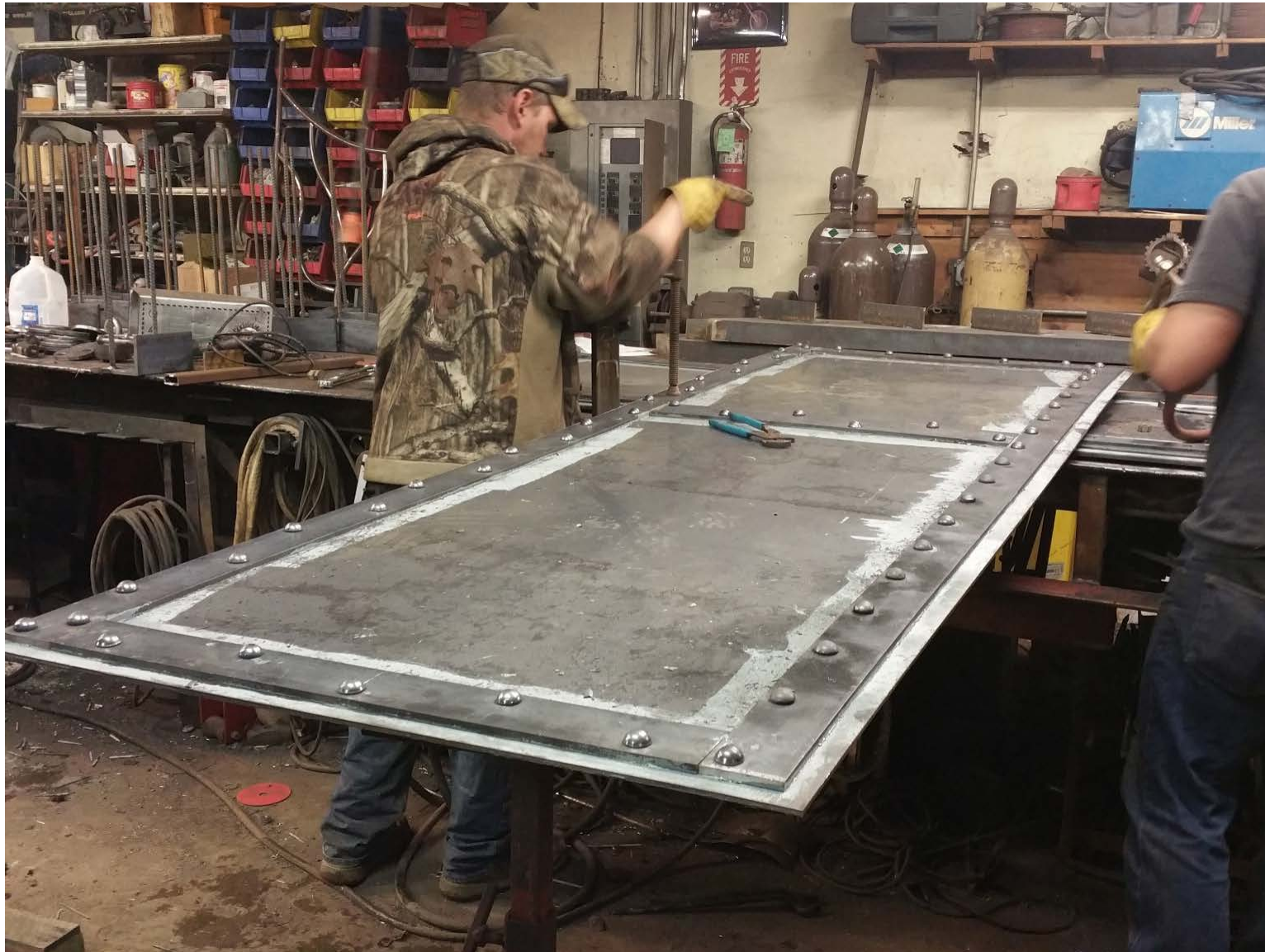
Shop fabrication and riveting of replica doors.
