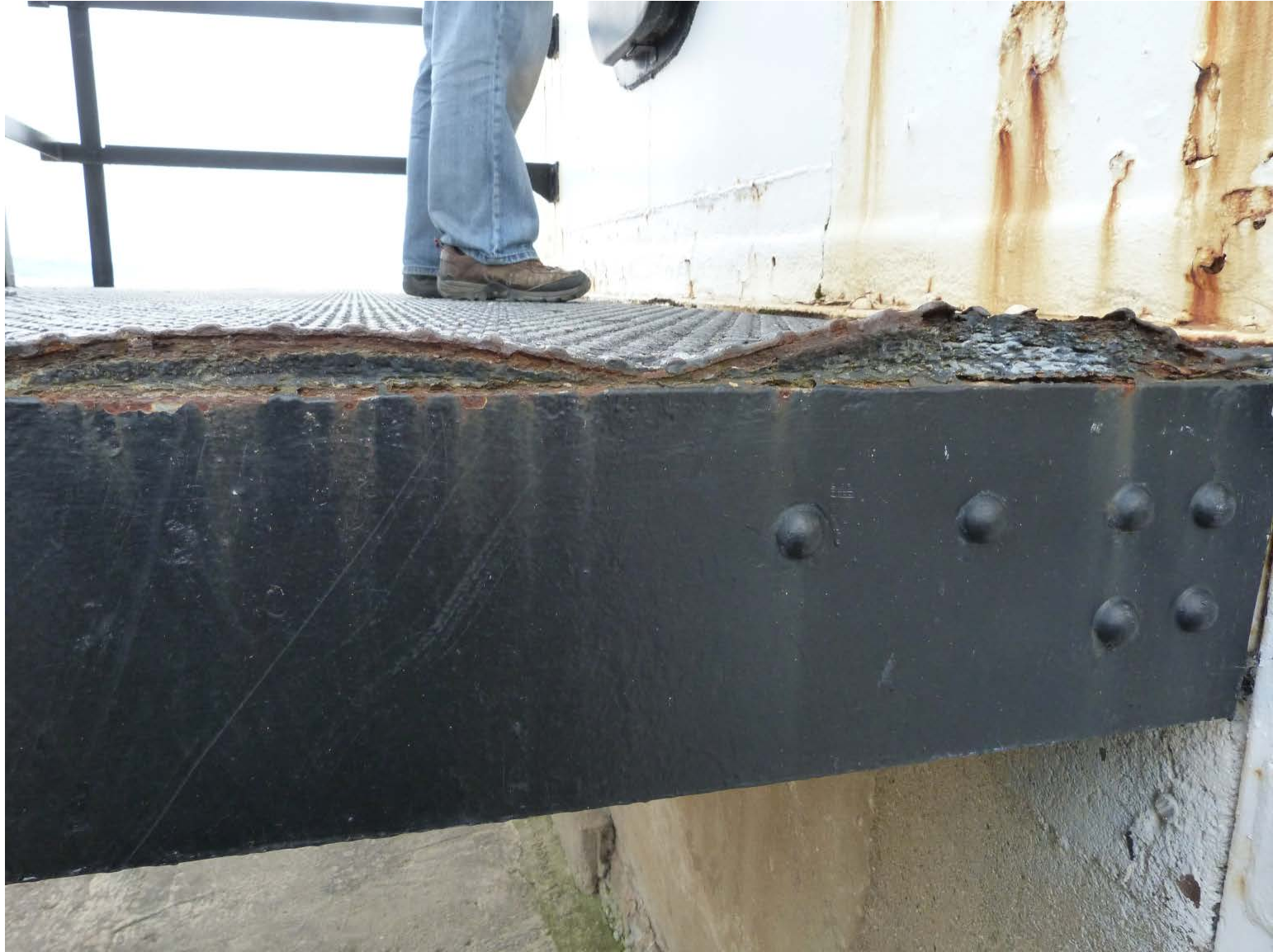
Lighthouse and Catwalks Before Project
