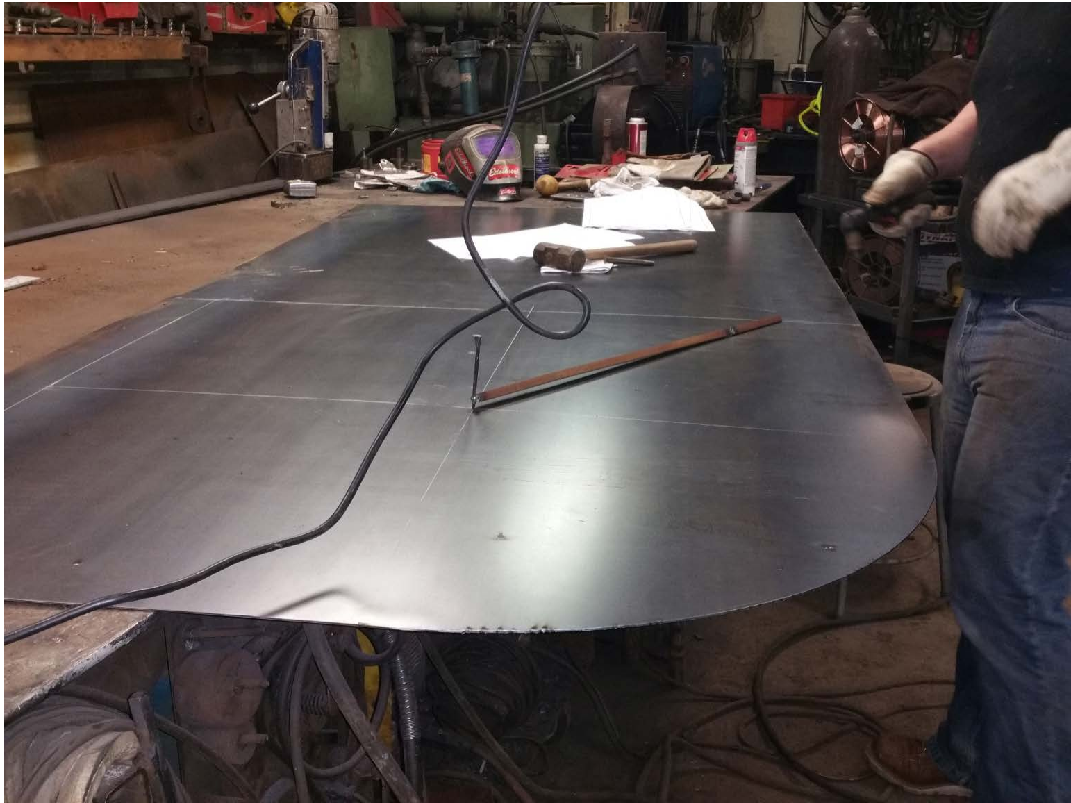
Fabrication of replica chimney cap.
