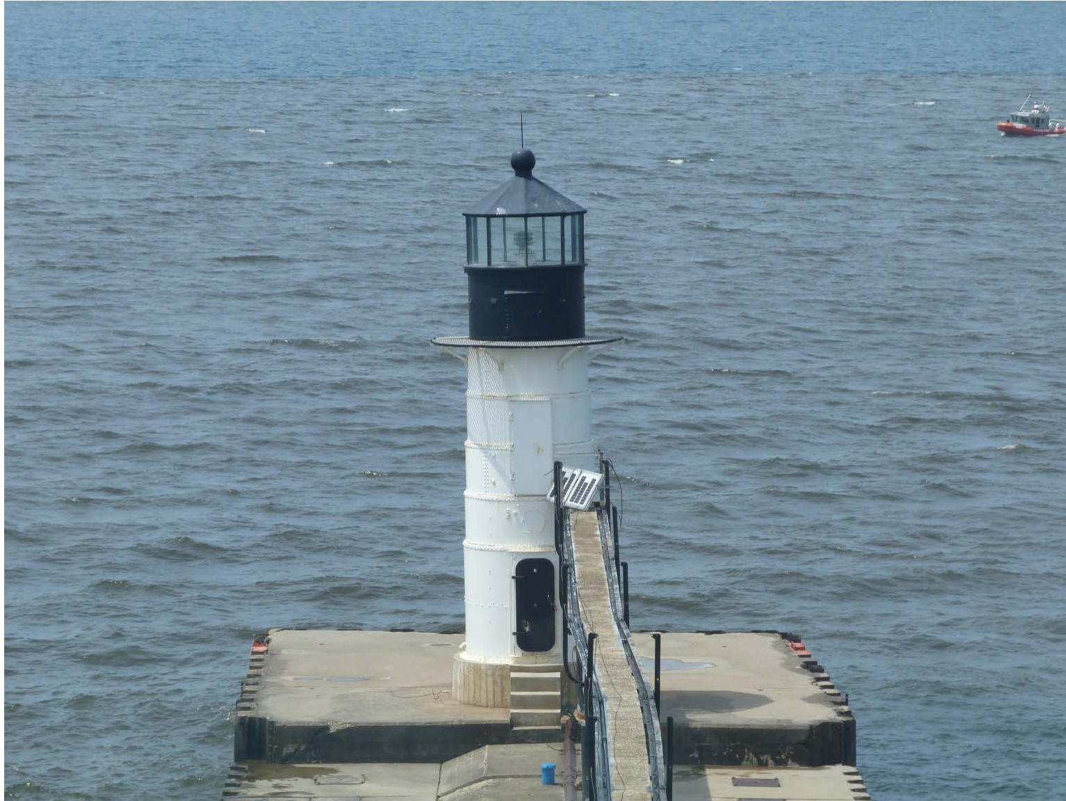
Lighthouse and Catwalks Before Project
