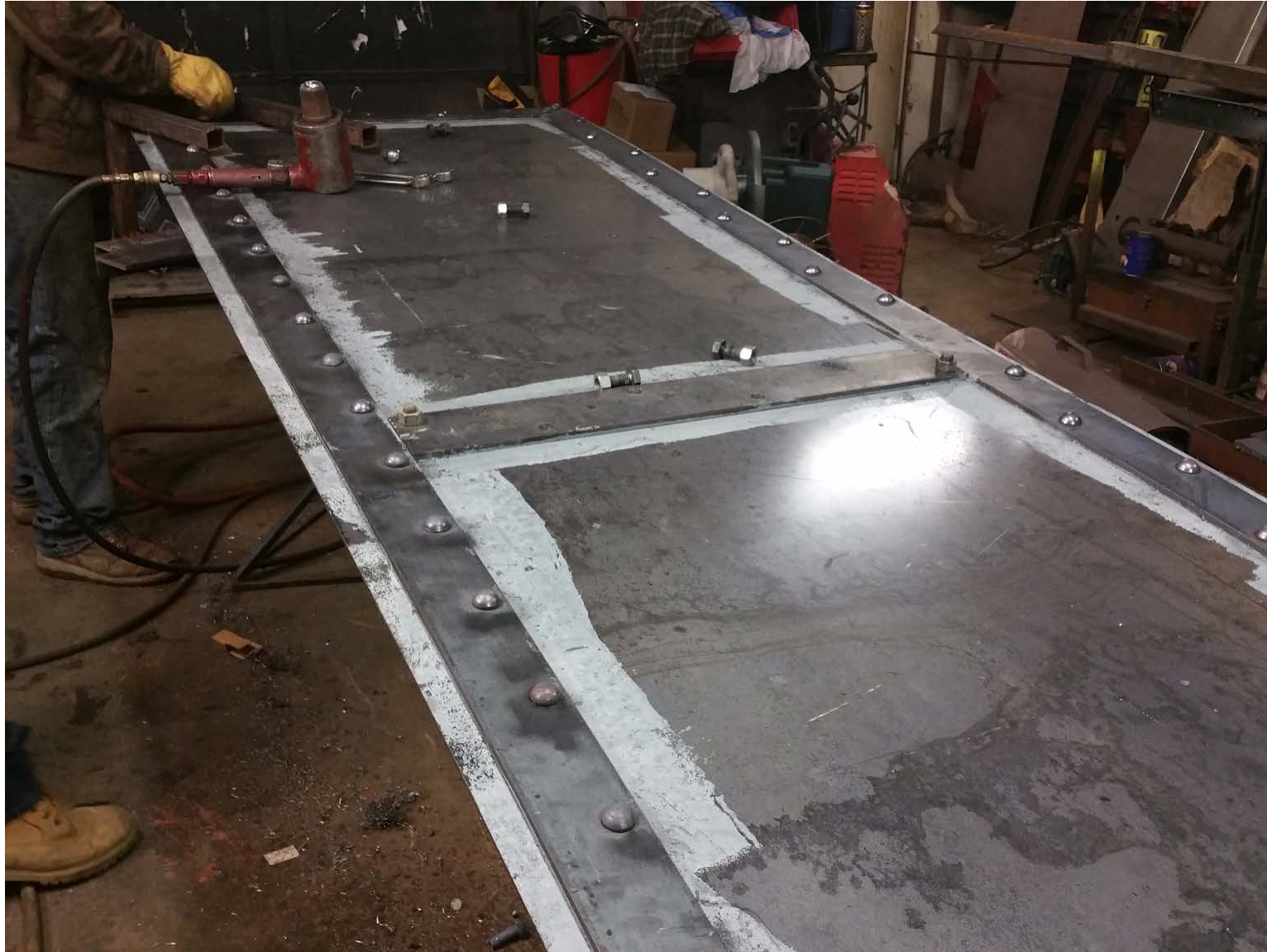
Shop fabrication and riveting of replica doors.
