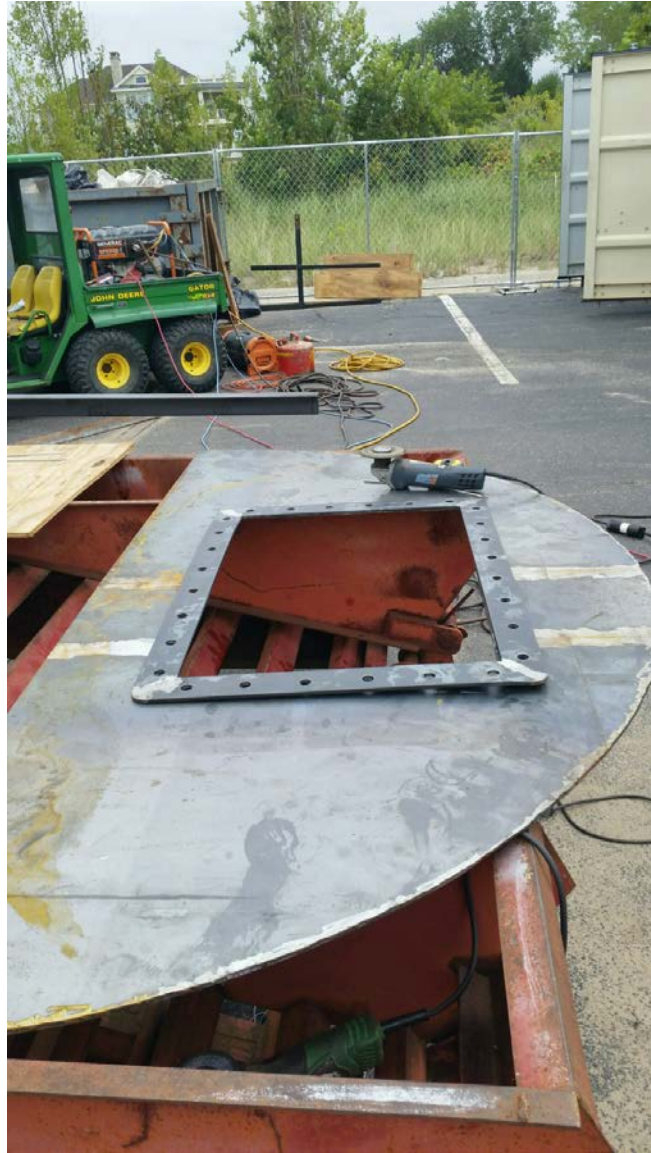
Field assembly of new deck section.
