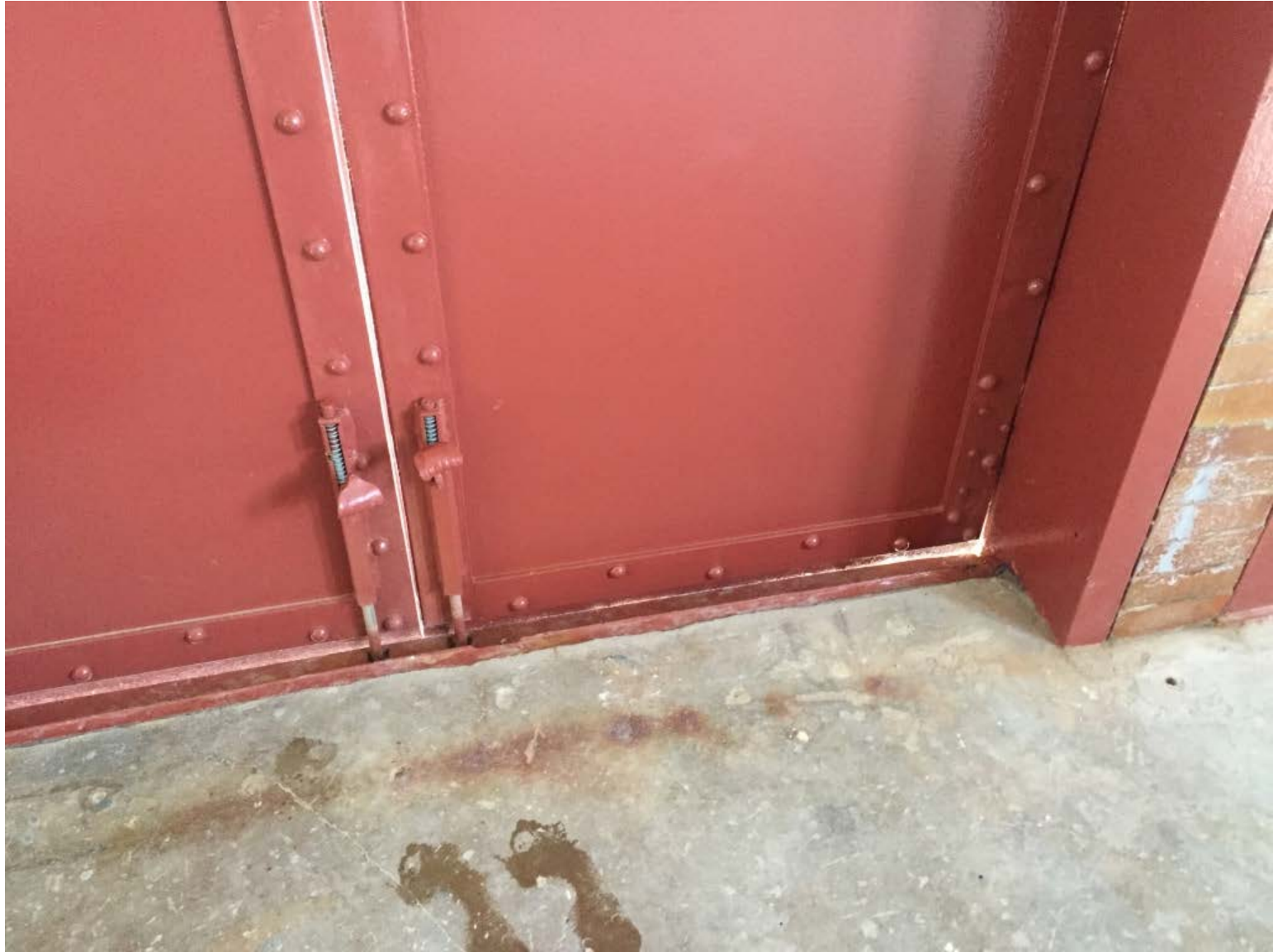
Replicated, hot-riveted doors installed, after painting.
