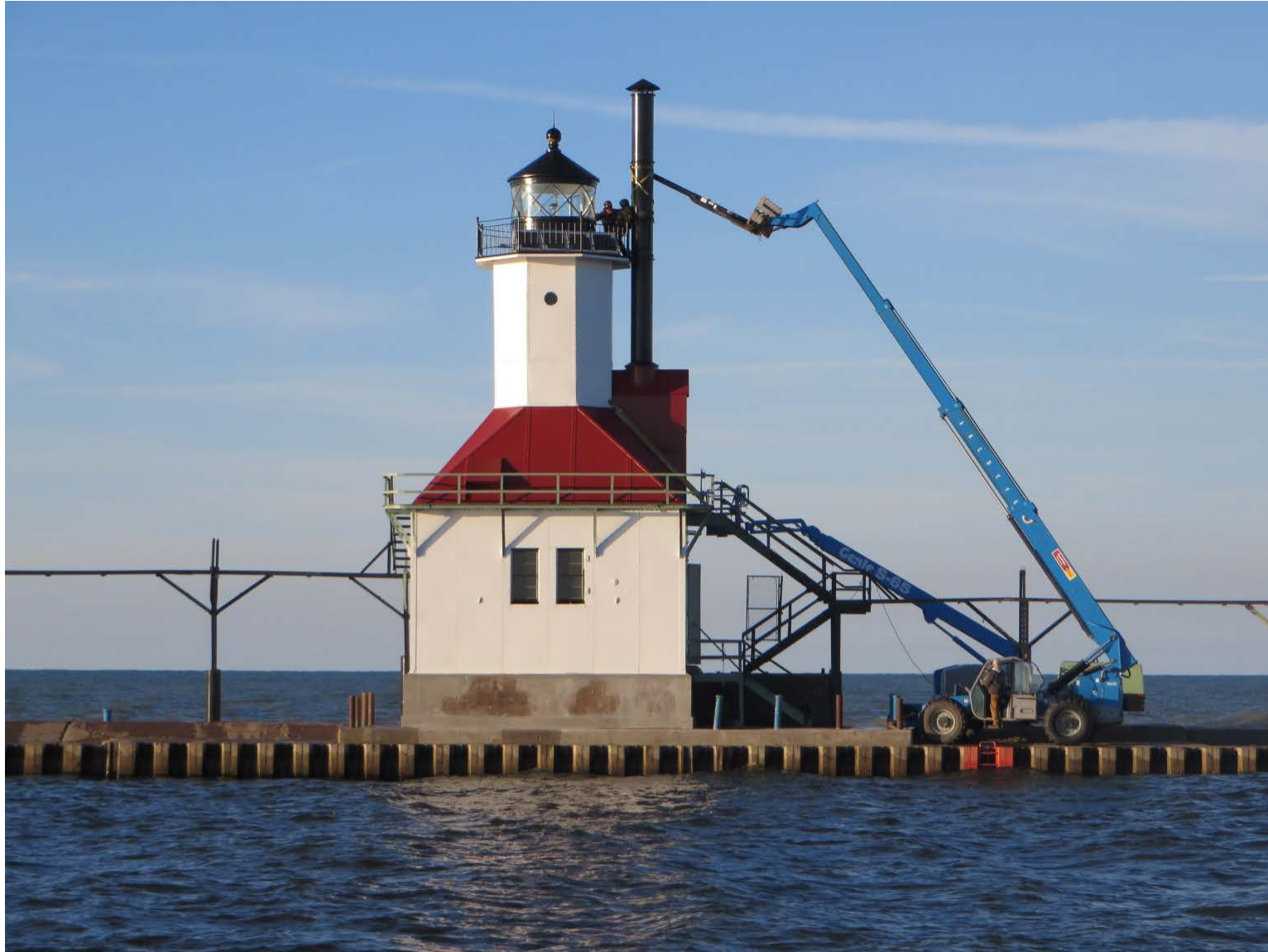
Installation of replica chimney. Lighthouse restoration mostly complete.
