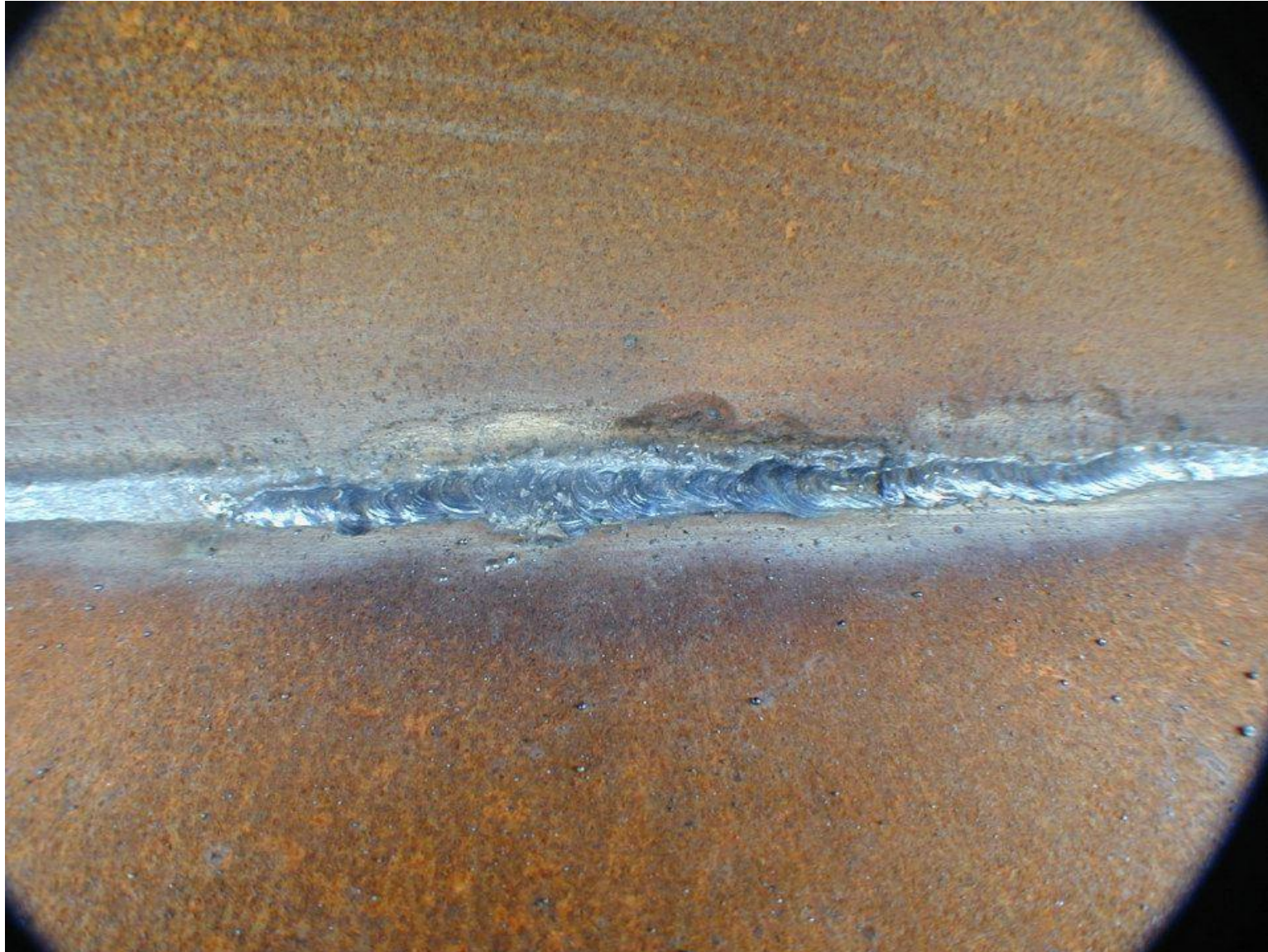
Pad welding repair in progress for section loss hidden inside a built-up beam at a corner.
