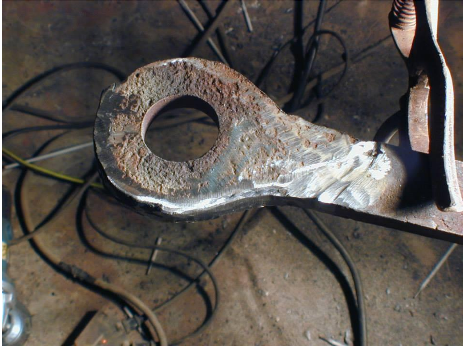
Pad welding repair in progress for deteriorated eyebar.
