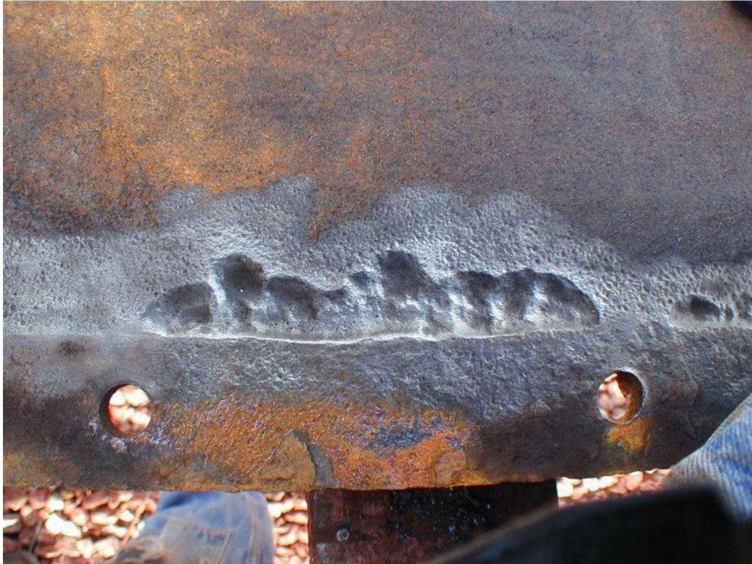
Section loss on floor beam, cleaned and ready for pad weld repair.
