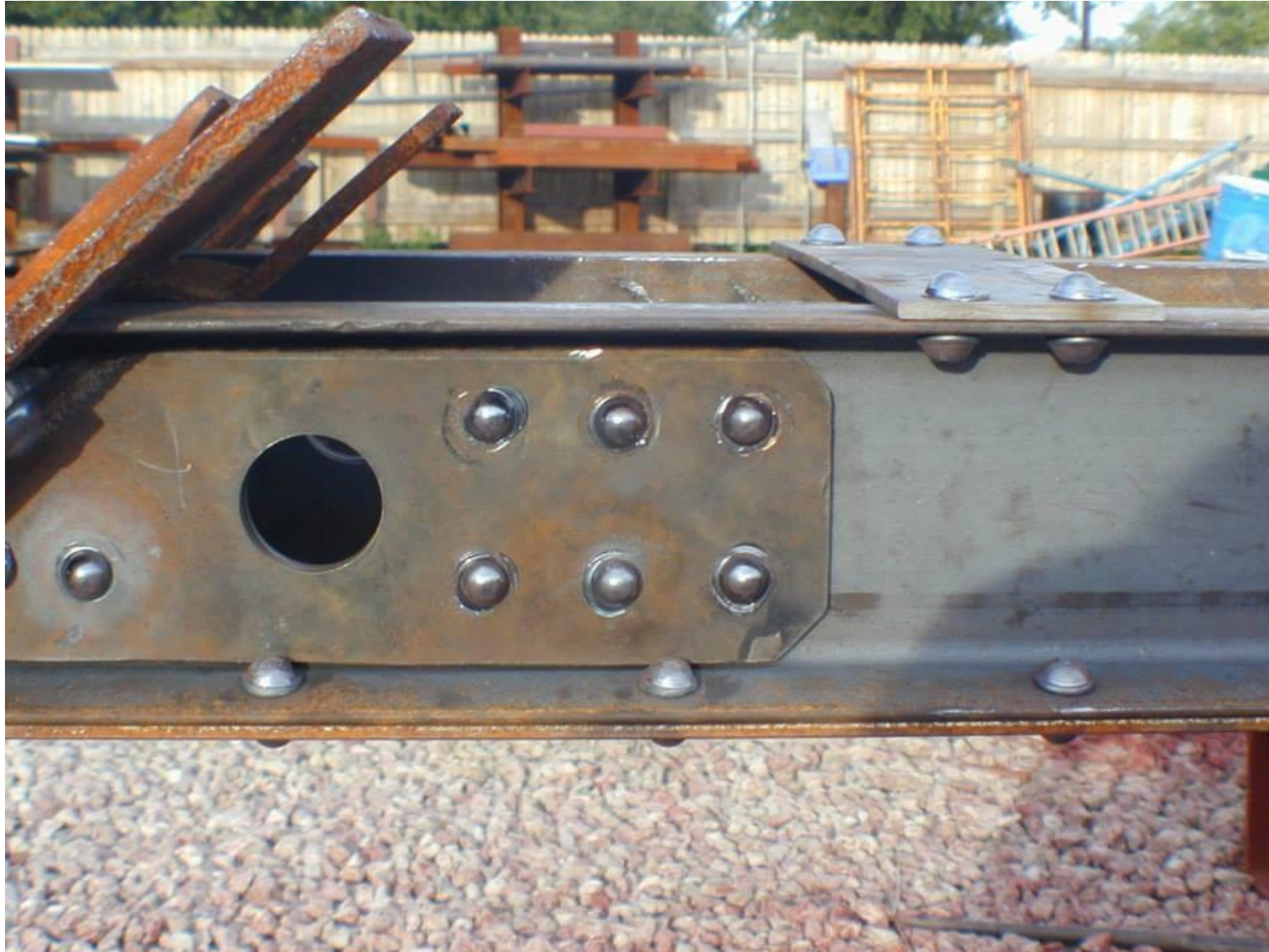
Restored end post showing newly driven rivets by Bach Steel.
