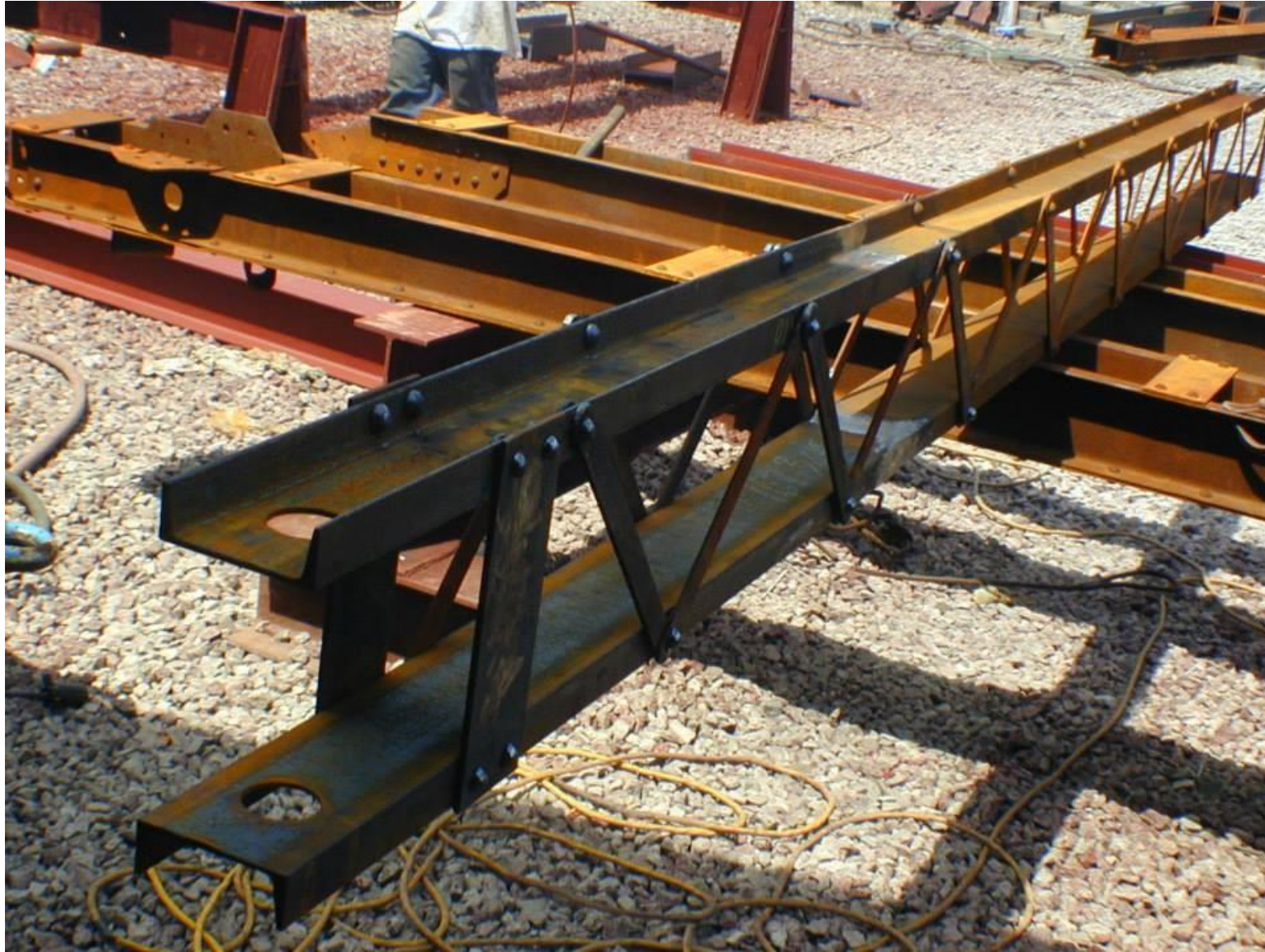
Restored vertical member. The left half is replicated, while the right half is original material.
