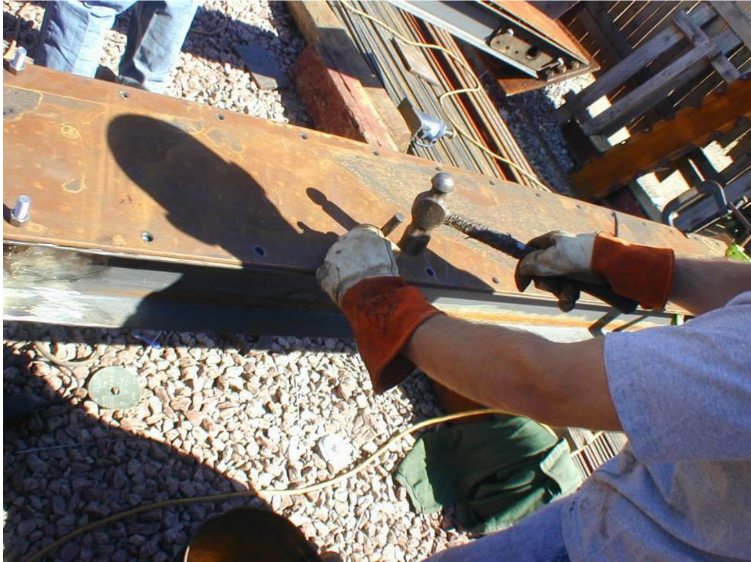
Using a locator punch to mark holes for drilling.
