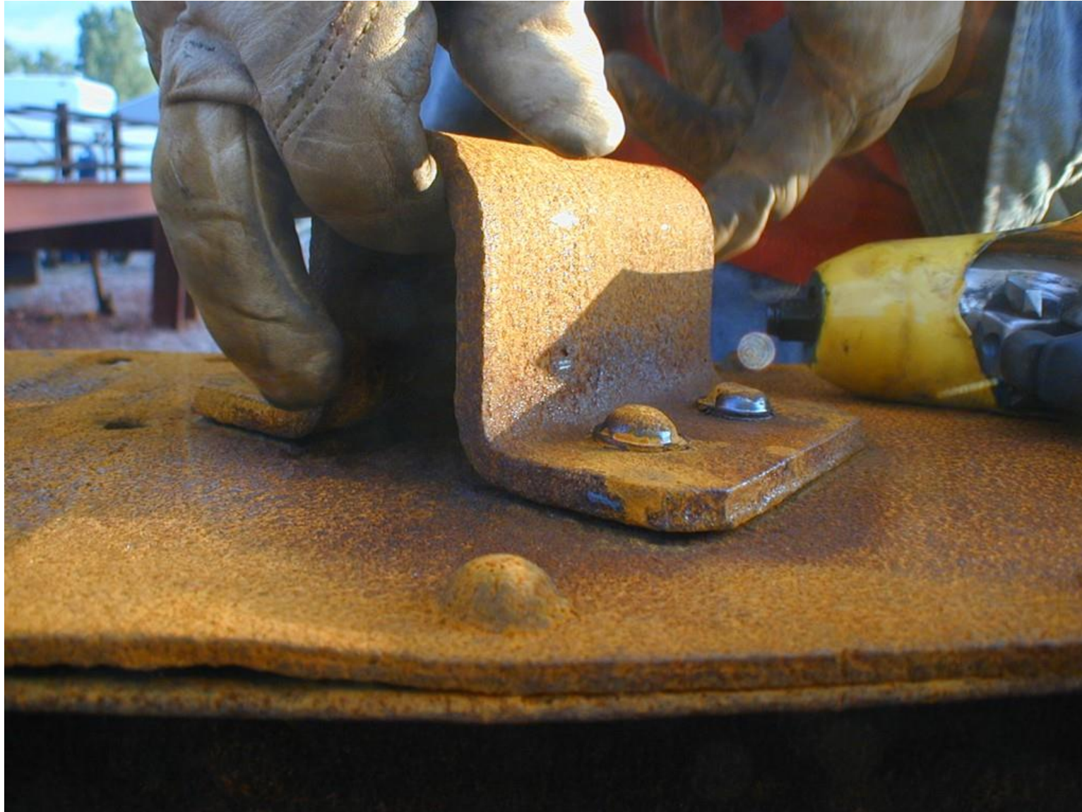
Newly riveted lateral bracing attachment on top chord.
