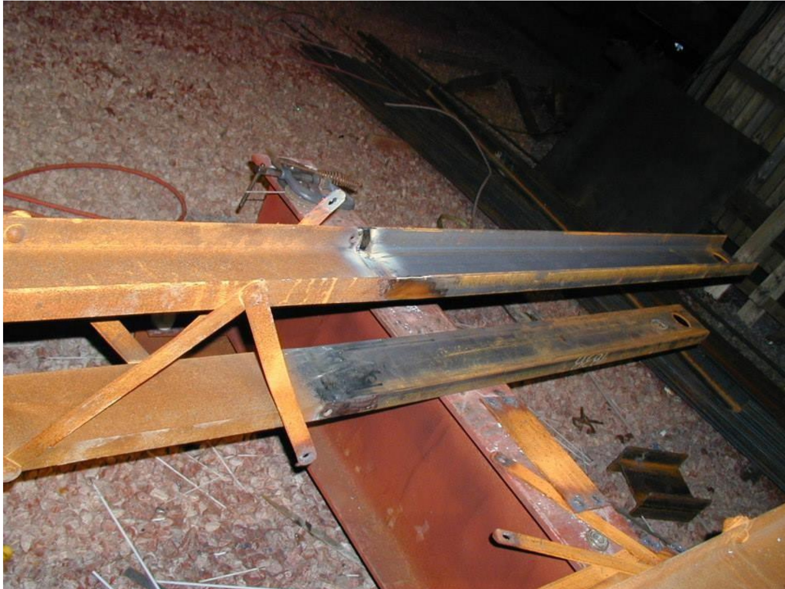
Repair in progress of a vertical member. Work included replication (including rivets) of a section of deteriorated vertical member which was welded on to the remaining original portion.
