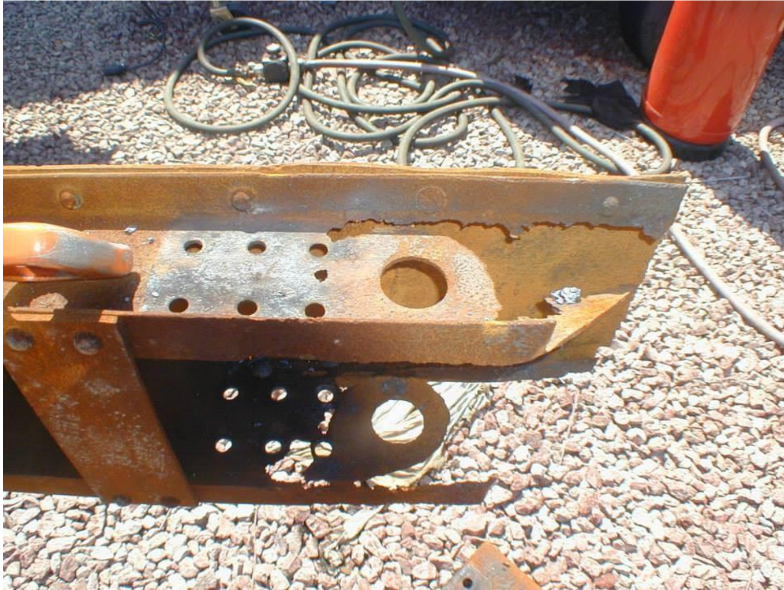
Condition of end post before restoration showing severe deterioration.
