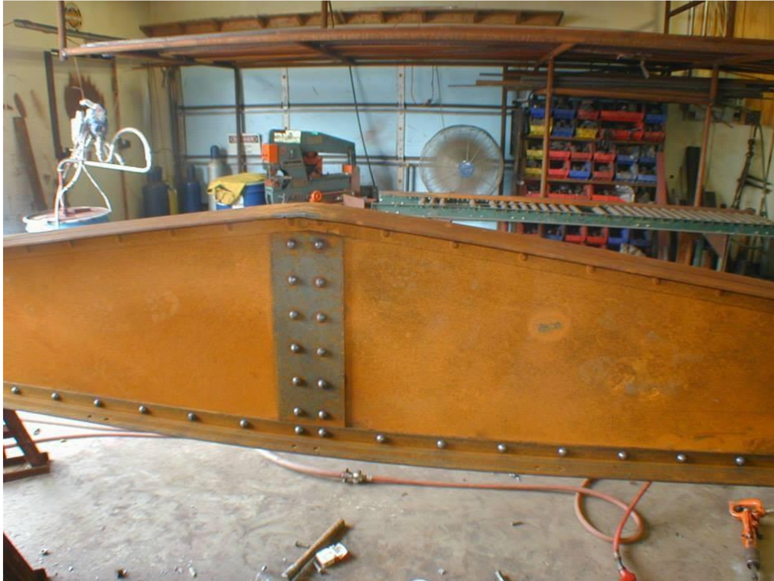
Repair of floor beam. The shiny rivets in the middle and on the lower portion of the photo are new rivets driven by Bach Steel.
