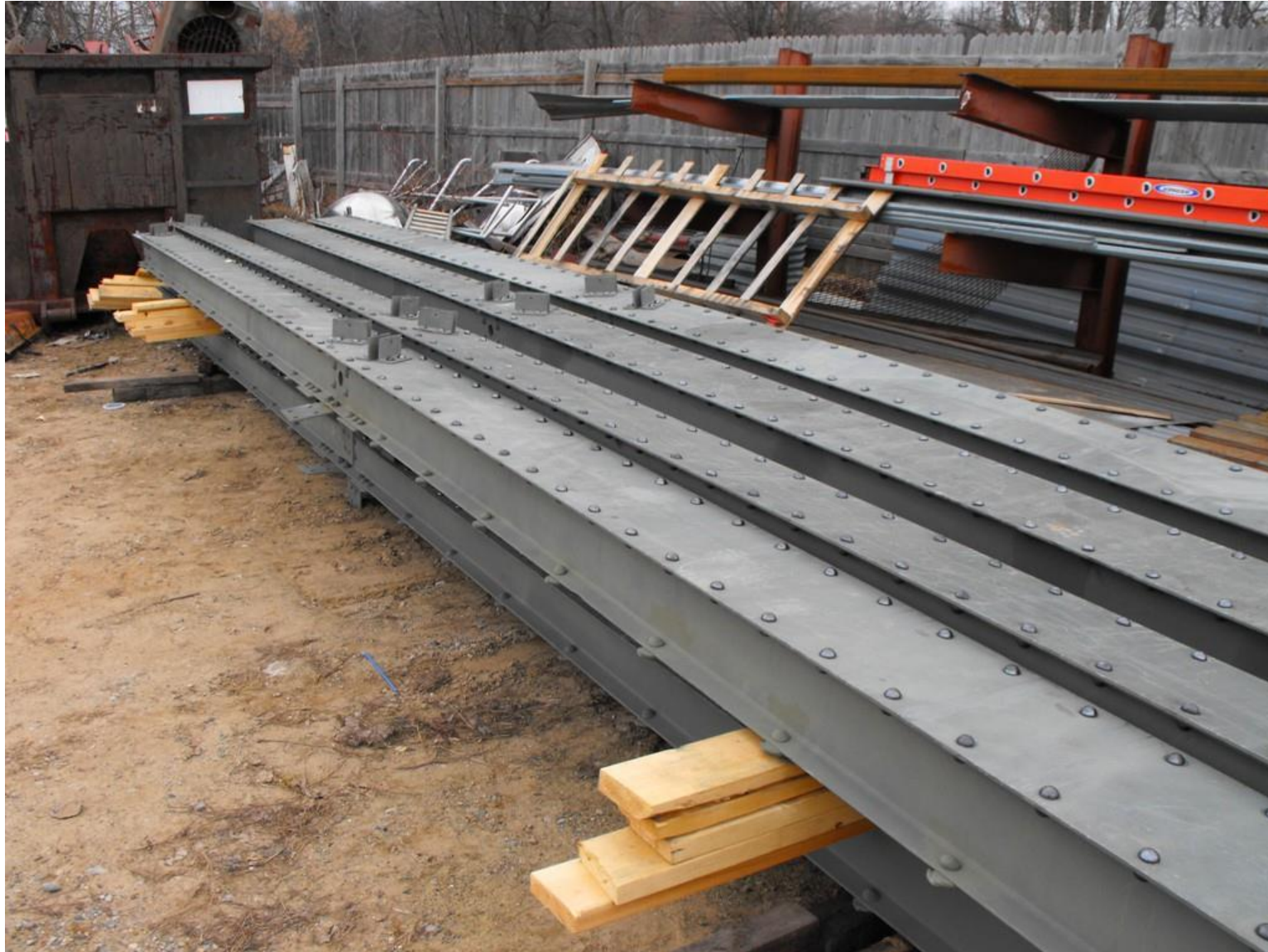
Newly driven rivets in a top chord of a truss bridge.
