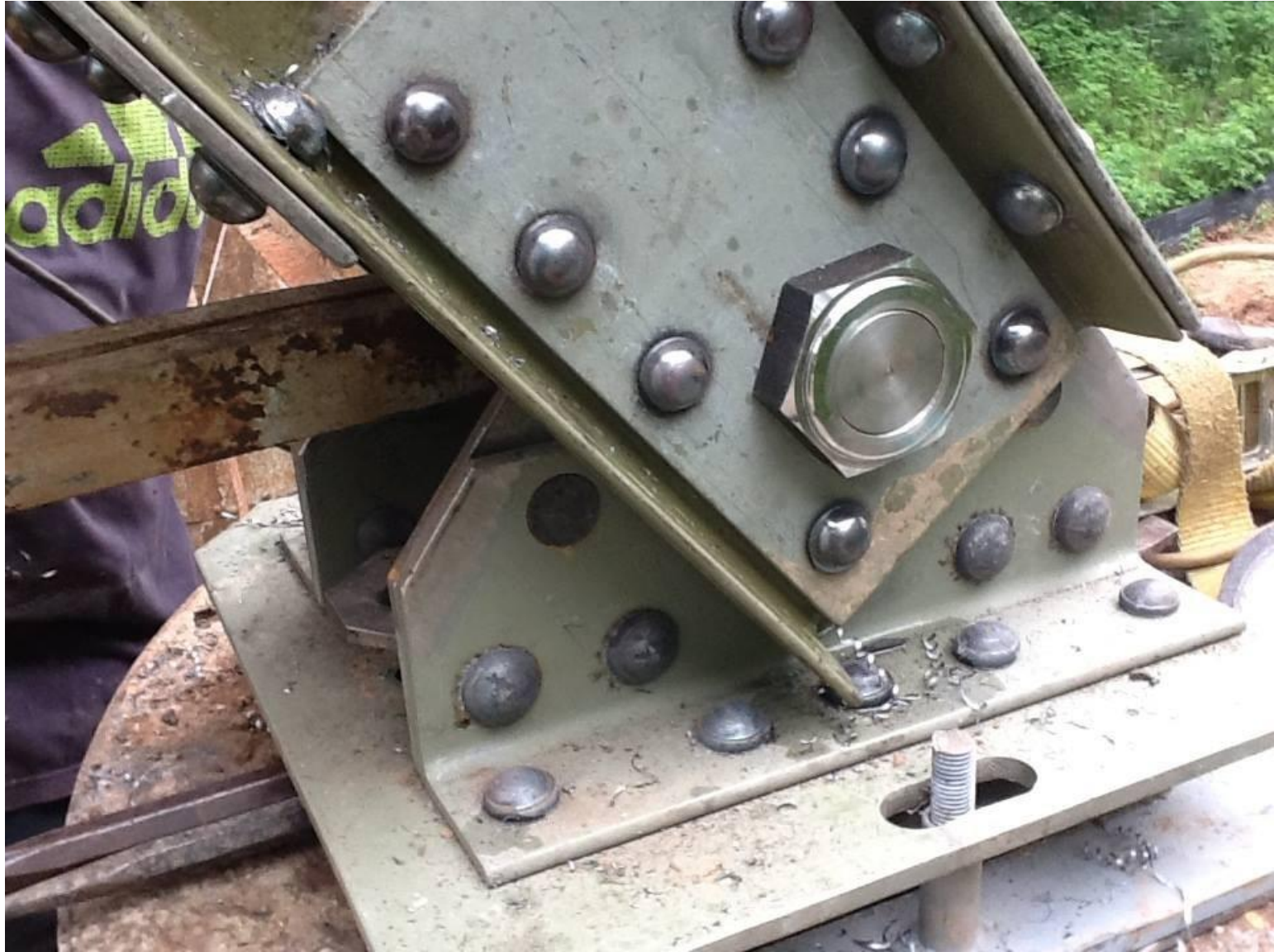
New rivets installed in a replicated truss bridge shoe.
