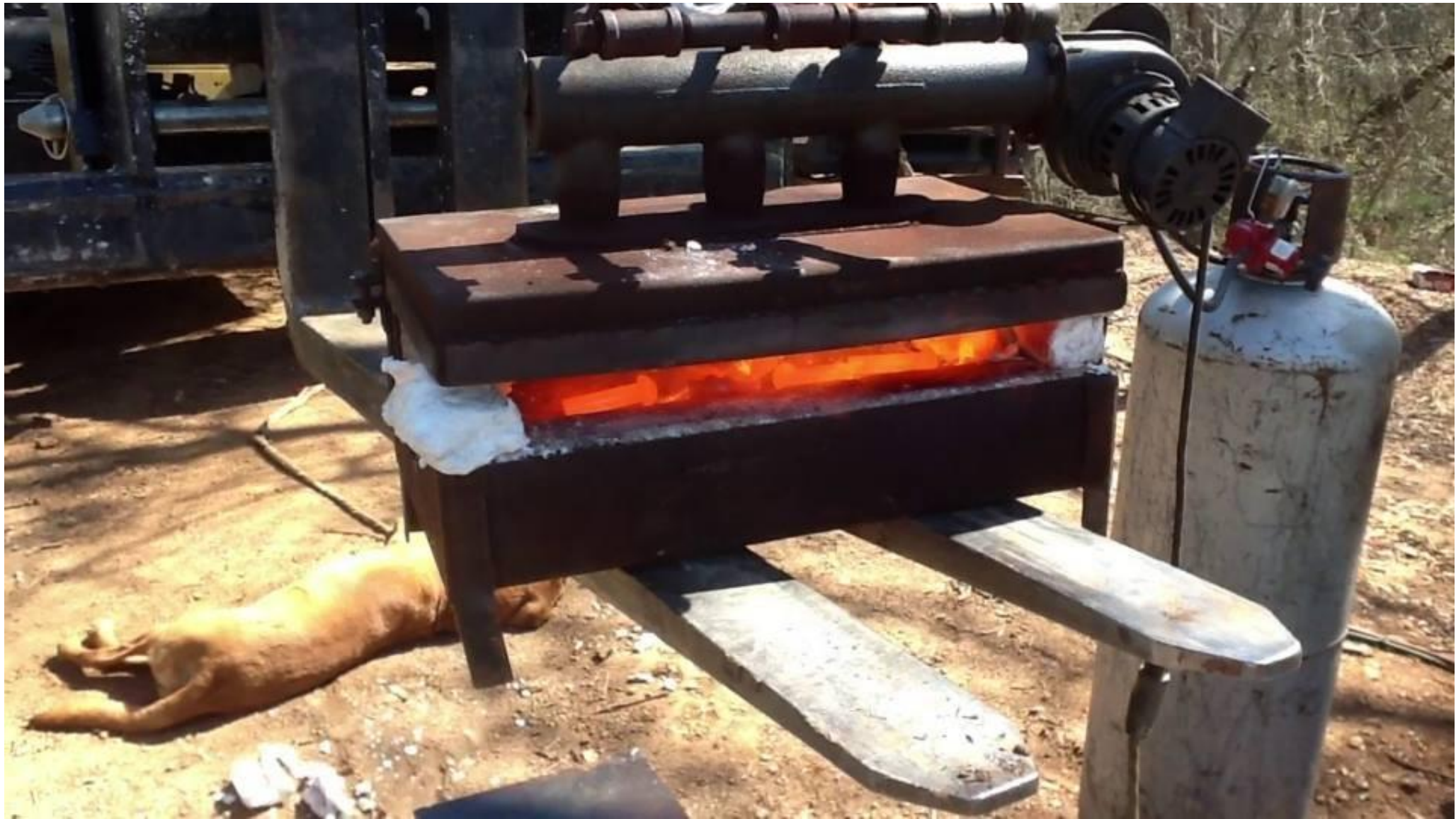
This is a forge, where rivets are heated to the proper temperature for driving.
