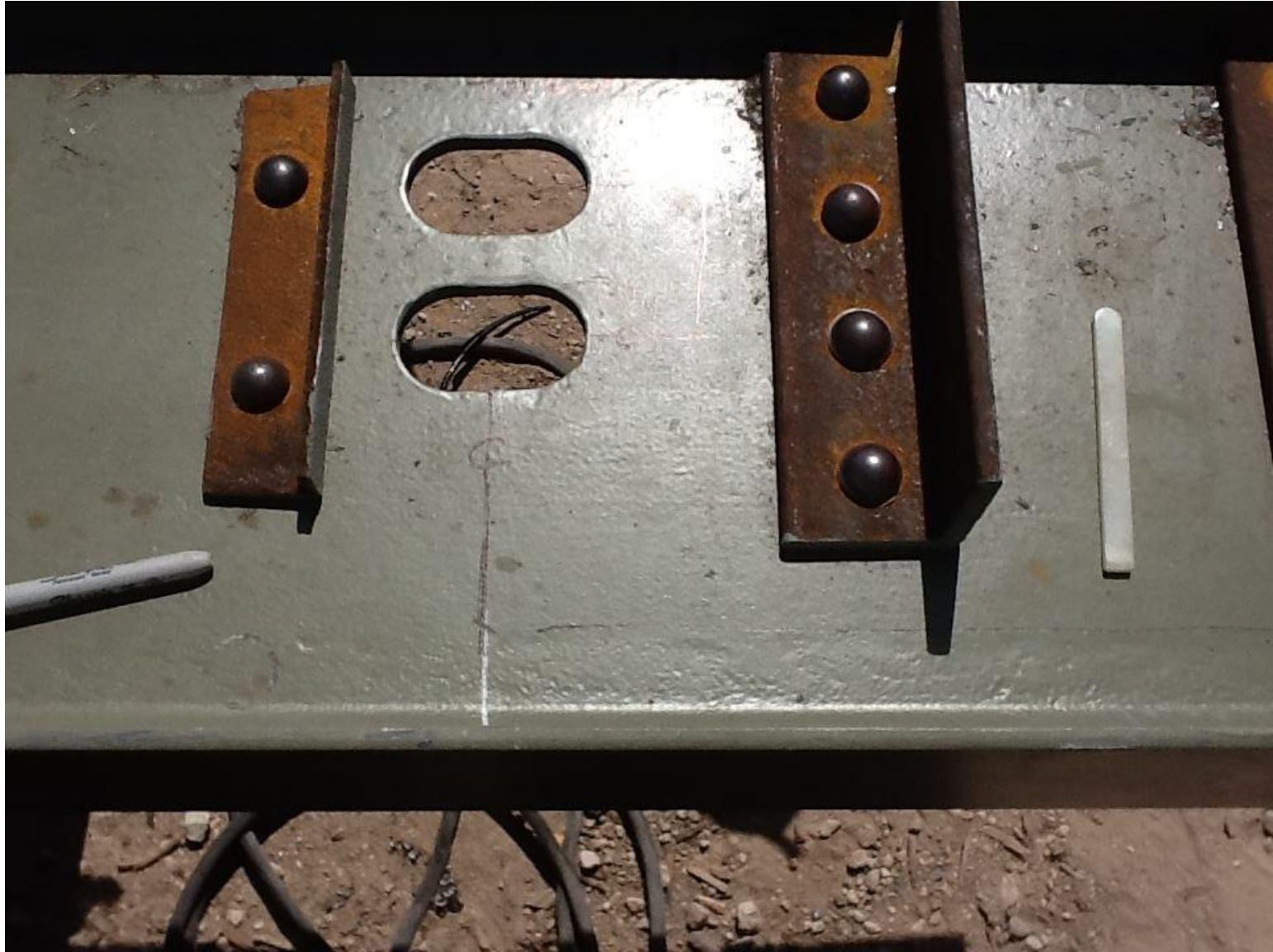
Newly riveted angles on floor beam.
