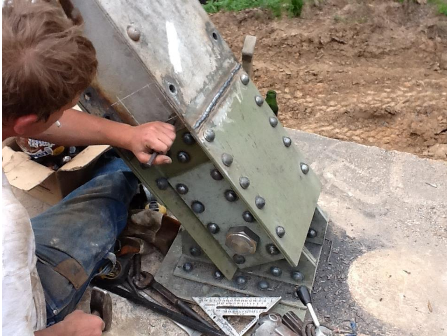
Replicated foot and base of end post shown after it was welded on to the original portion of the end post.
