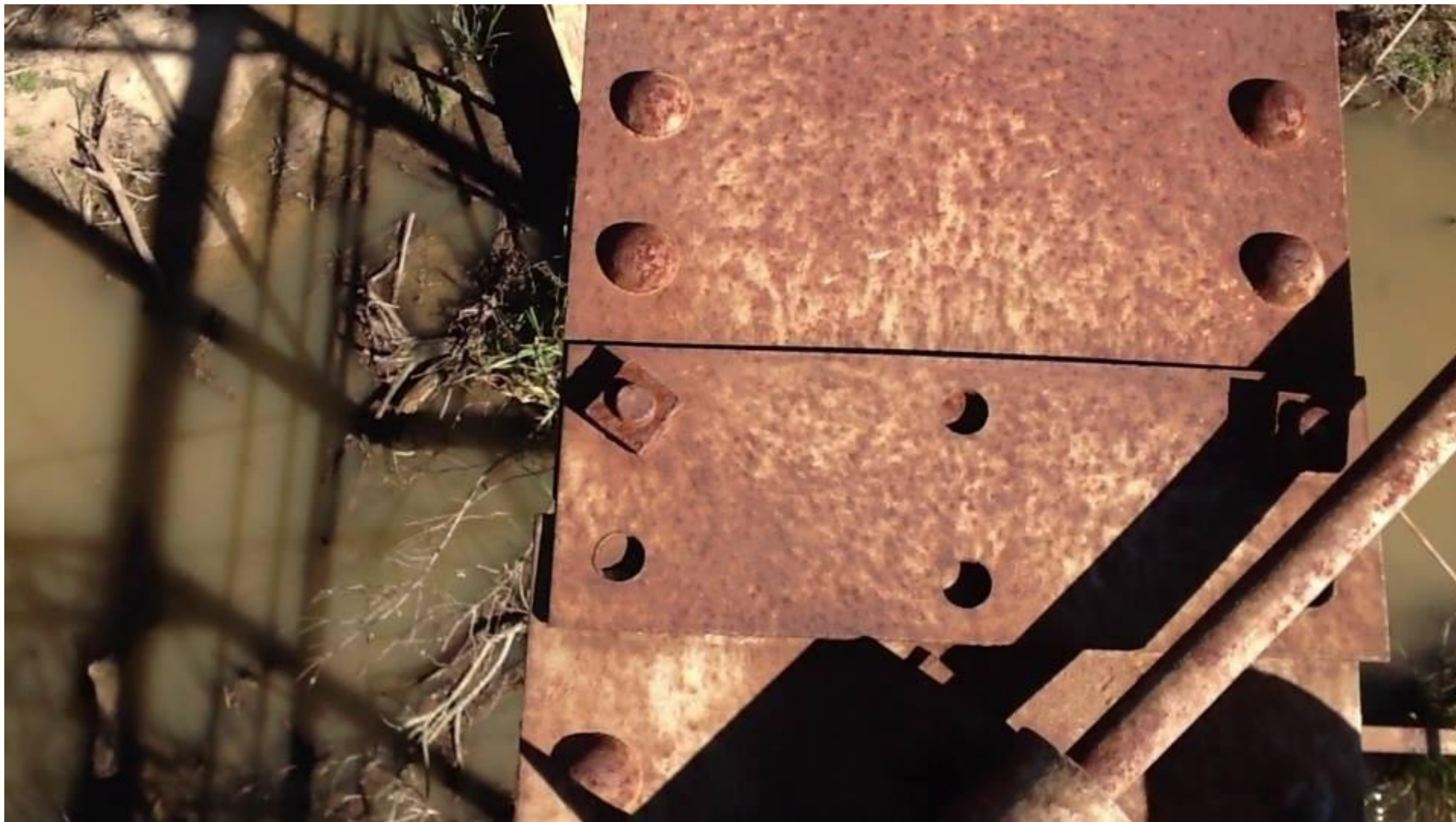
This bridge was relocated decades ago, and when it was re-erected, they did so poorly and only two nuts were put in on this splice plate. This was corrected during restoration.
