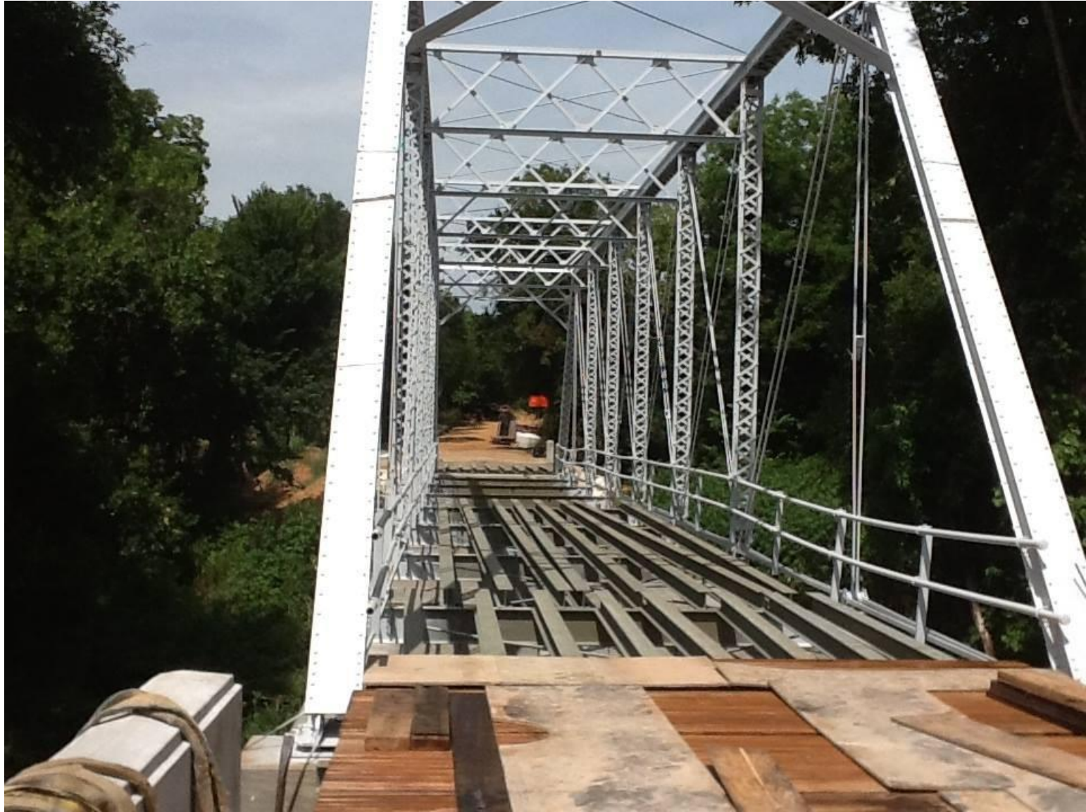
Truss restored, awaiting a deck
