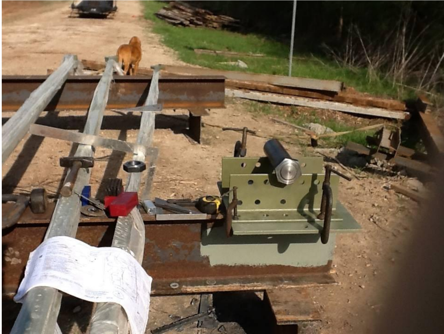
Replicating the foot of a bridge.
