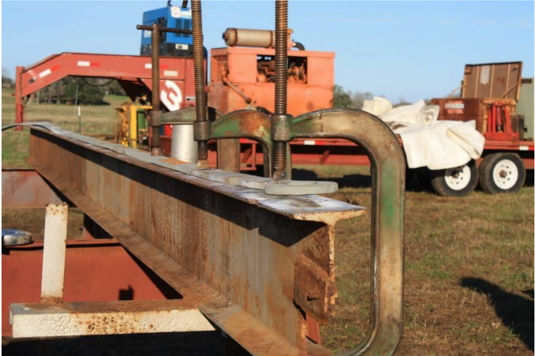
Straightening an eyebar.
