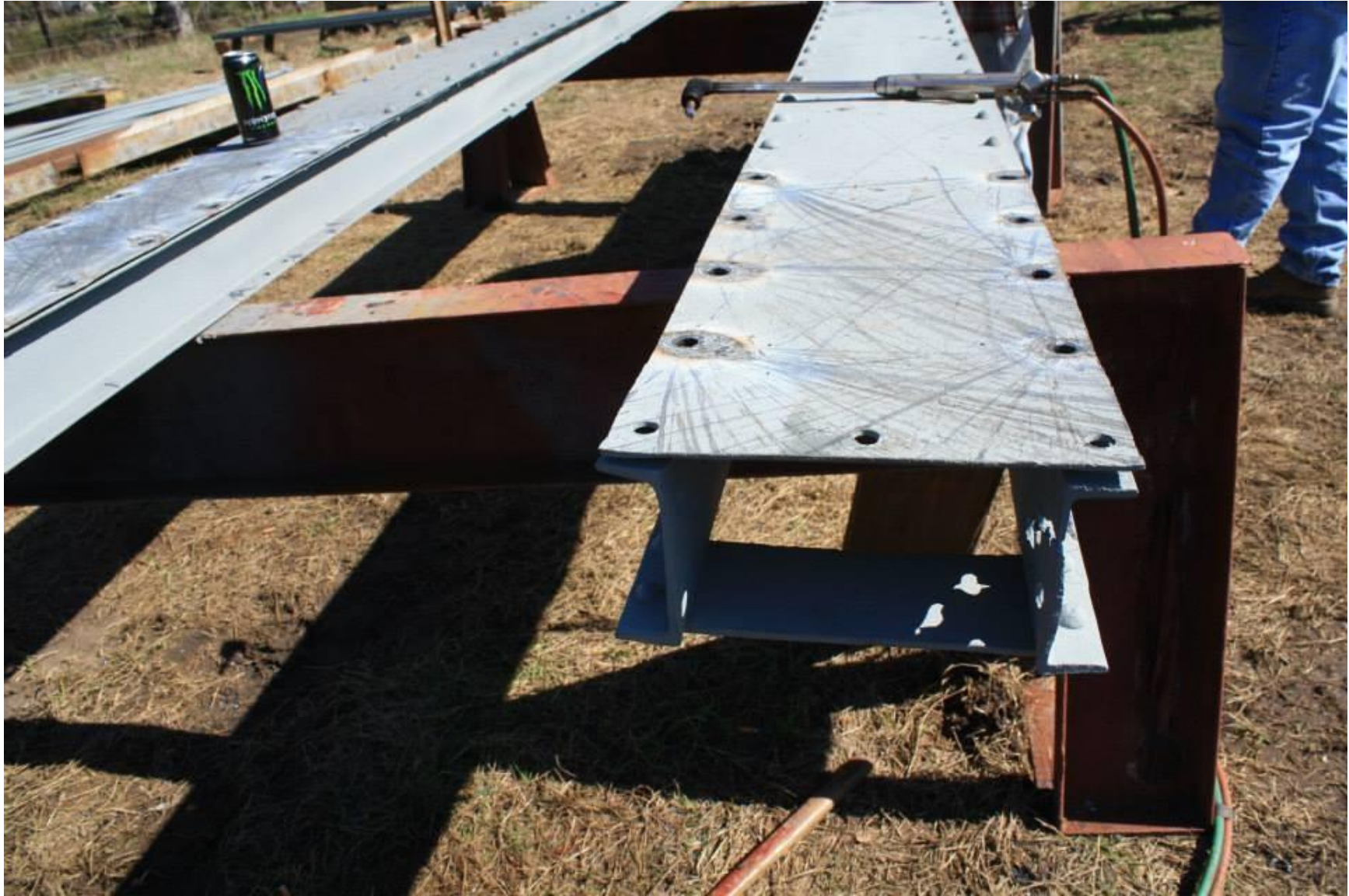
Cover plate after rivets were removed. Many contractors would have damaged the cover plate removing rivets in this manner, but Bach Steel knows how to do it without causing damage.
