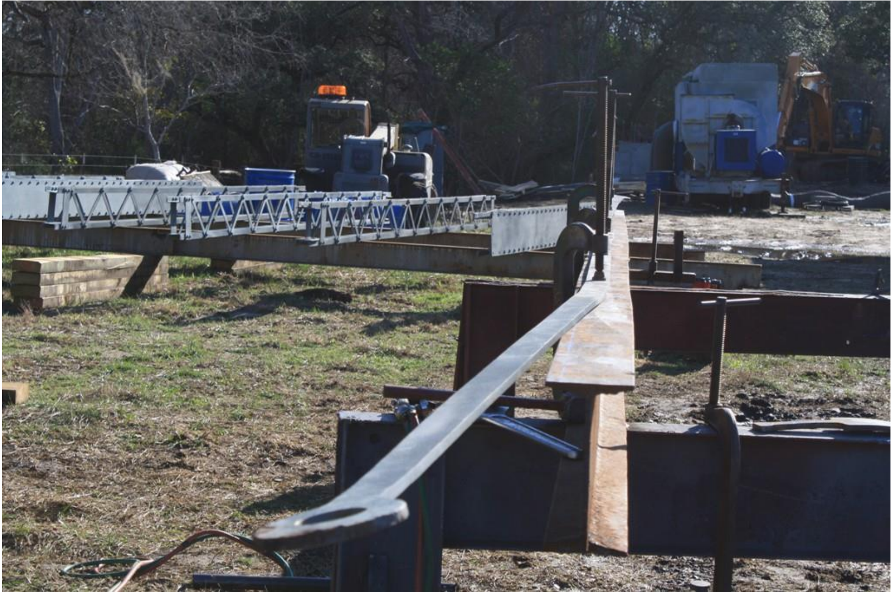
Severely bent eyebar prior to being straightened.
