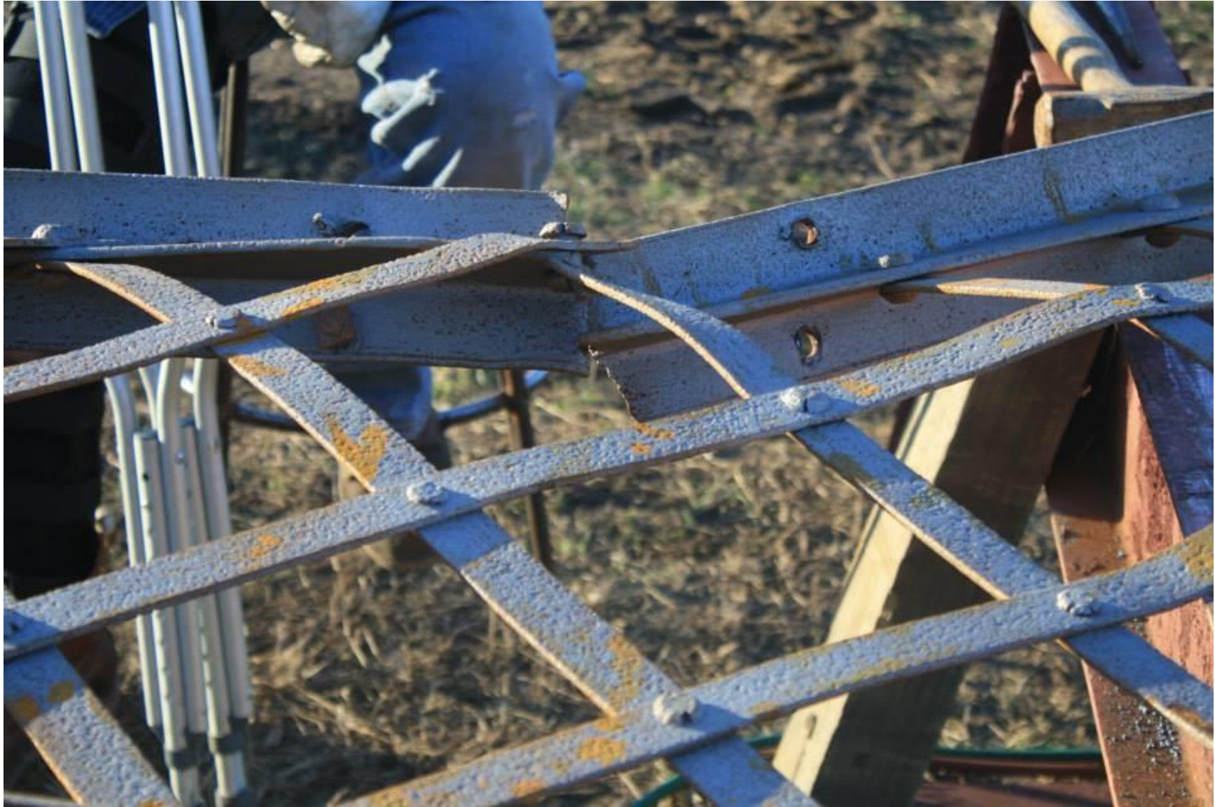
The portal bracing had extensive damage which was repaired.
