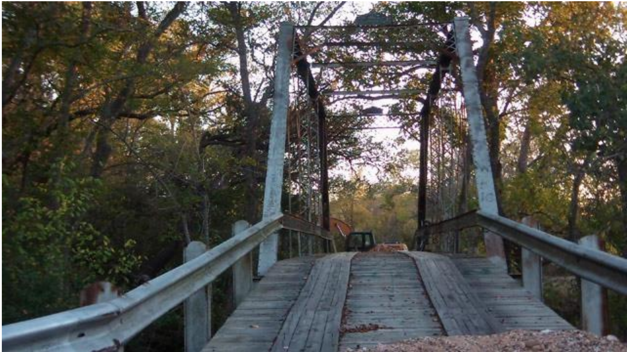
Bridge before restoration.
