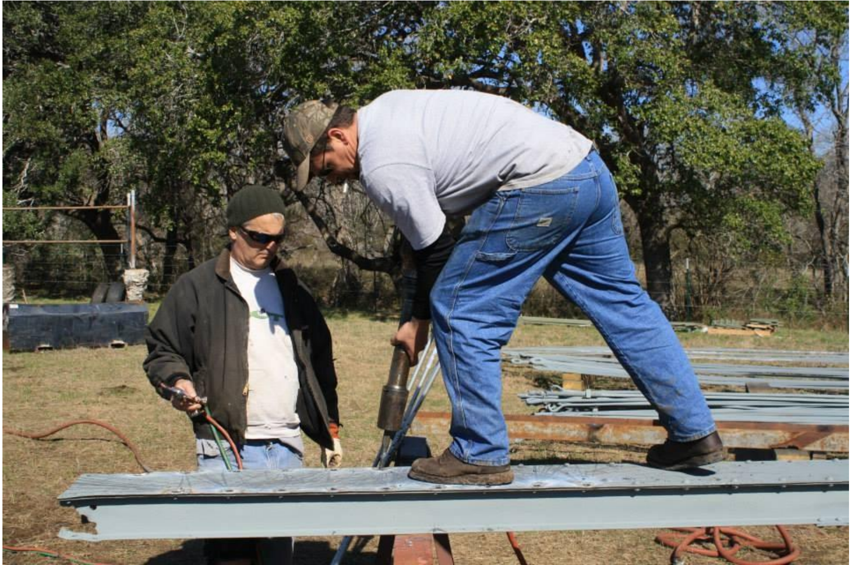
Removing rivets from cover plate.
