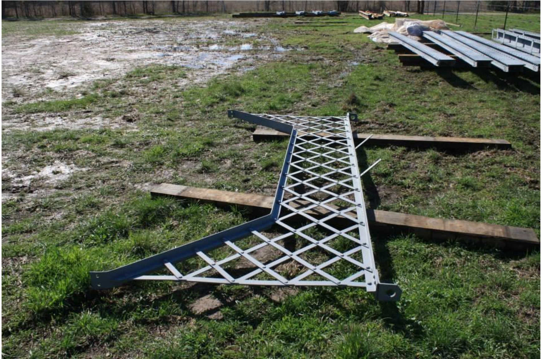
Restored portal bracing.
