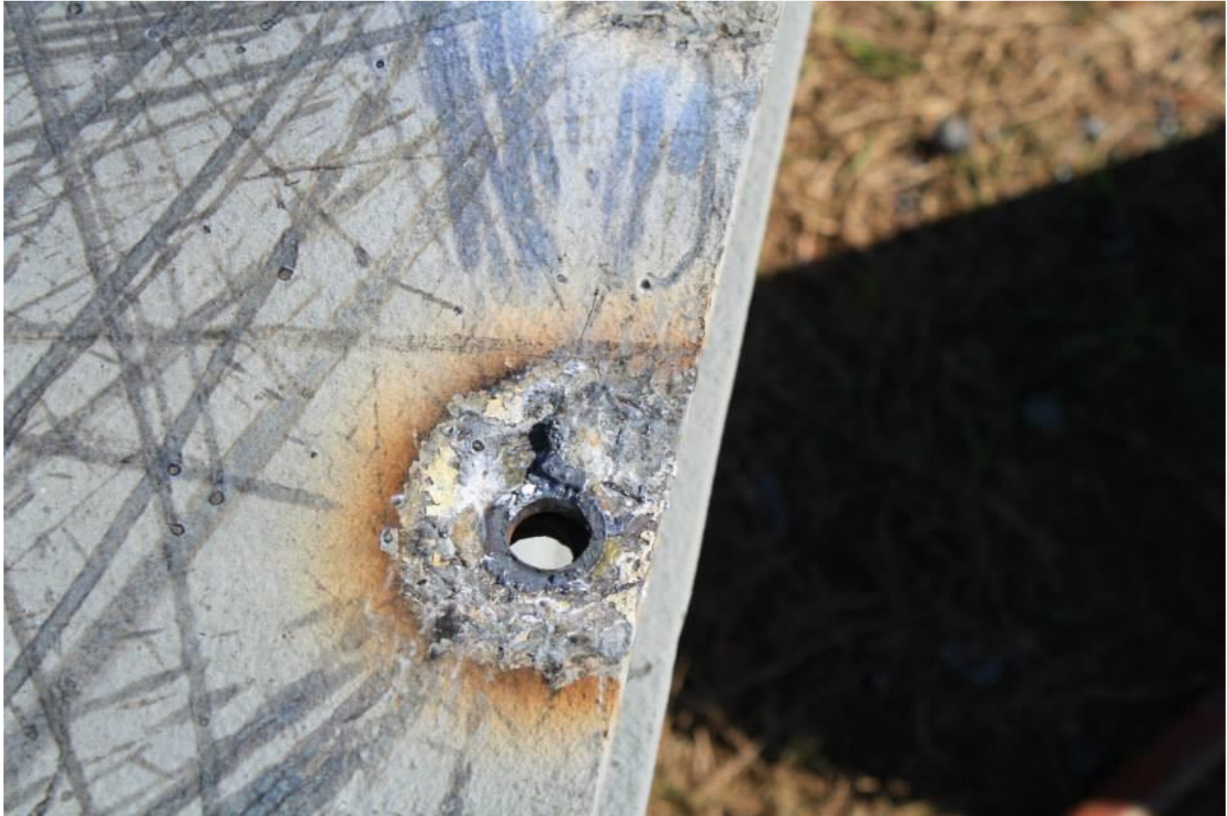
Cover plate after a rivet was removed. Many contractors would have damaged the cover plate removing rivets in this manner, but Bach Steel knows how to do it without causing damage.
