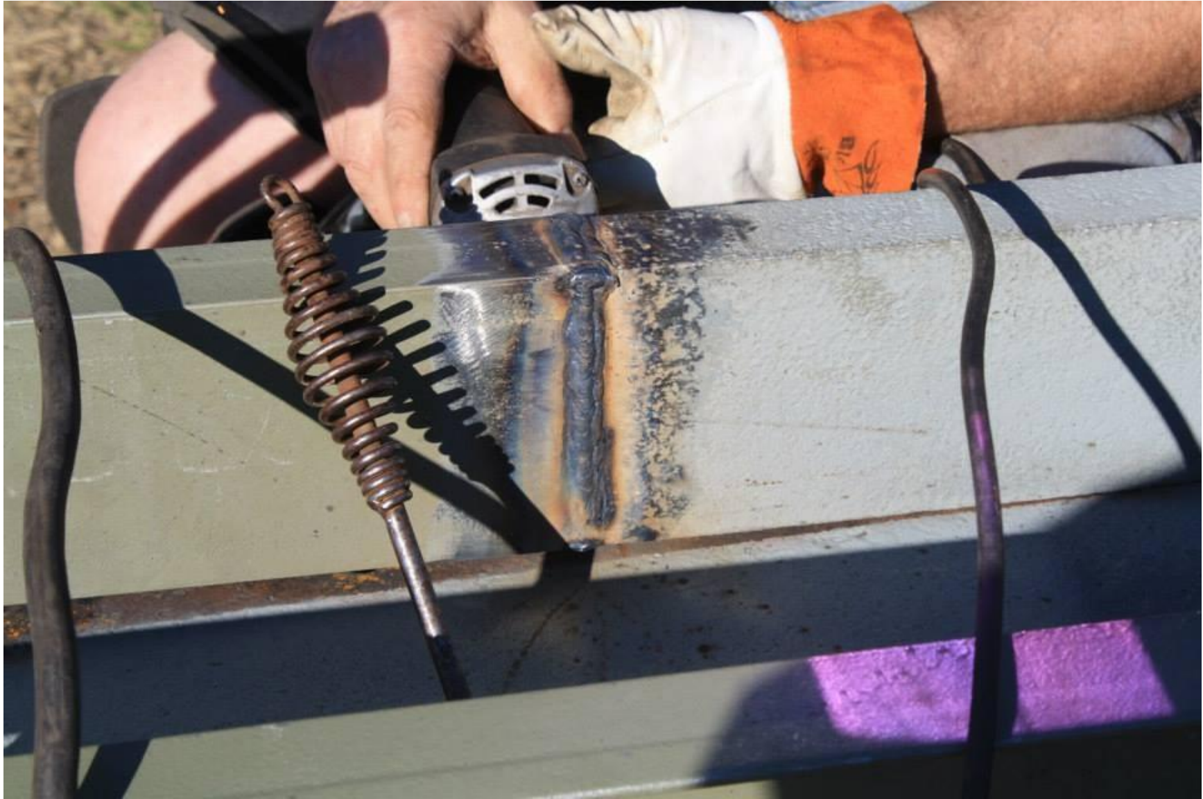
A replicated section of a beam is welded on to an original section of beam.
