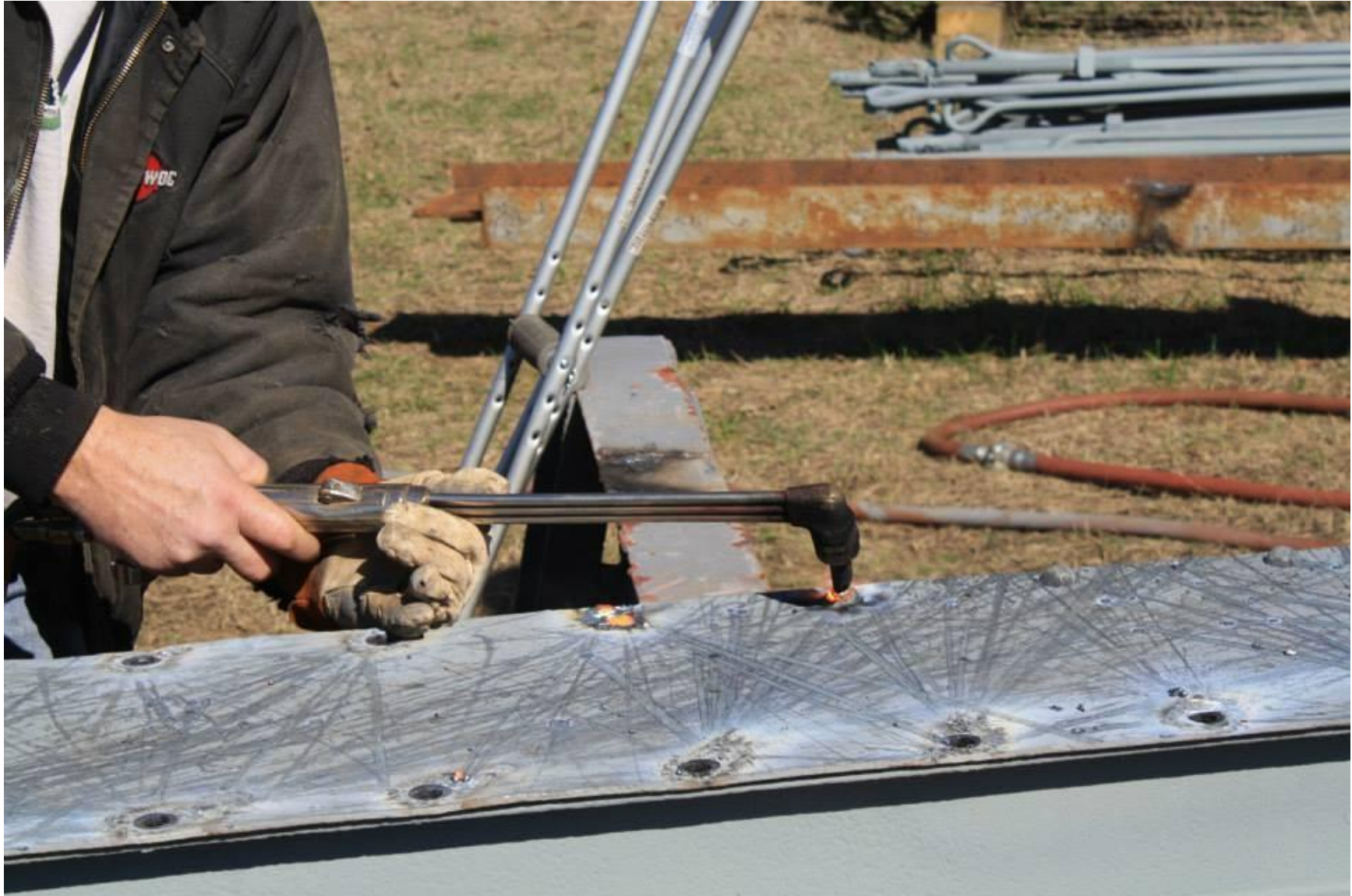
Using a cutting torch to remove rivets from a cover plate. Many contractors would have damaged the cover plate removing rivets in this manner, but Bach Steel knows how to do it without causing damage.
