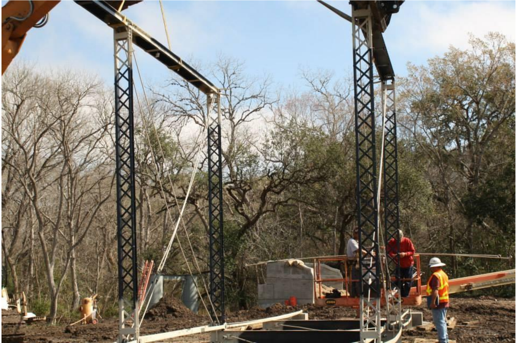
Reassembling the bridge.
