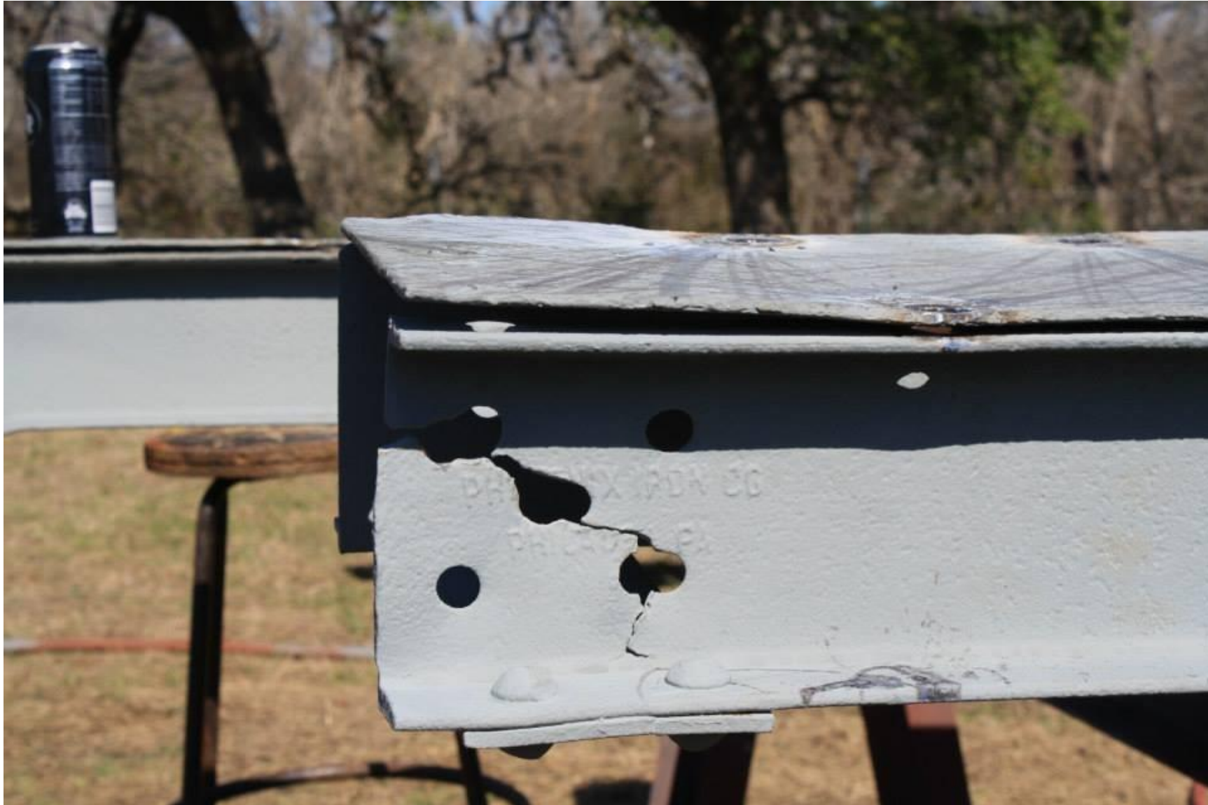
This detail shows a top chord section at the splice point. As originally built, this section was bolted to an adjacent section of top chord. Damage, clearly visible here, was what caused this bridge to be closed to traffic, initiating the restoration effort.
