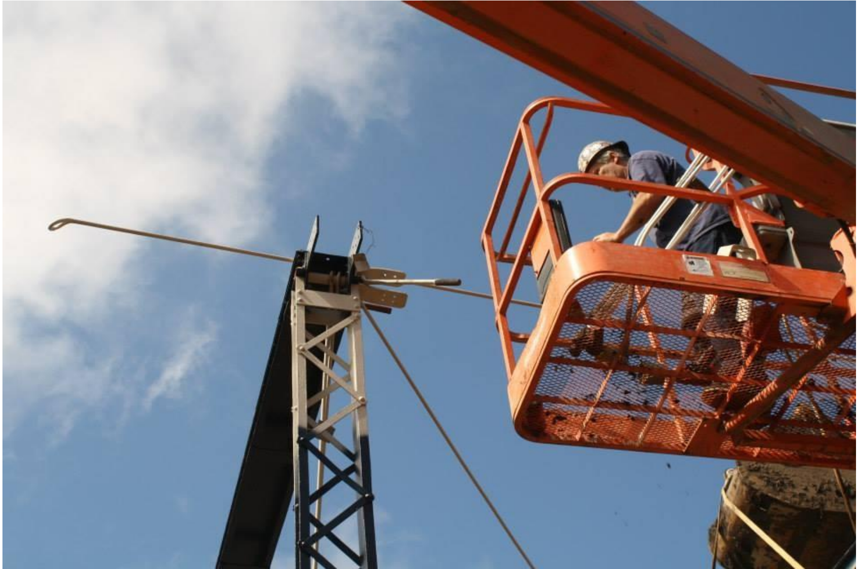
Reassembling the bridge.
