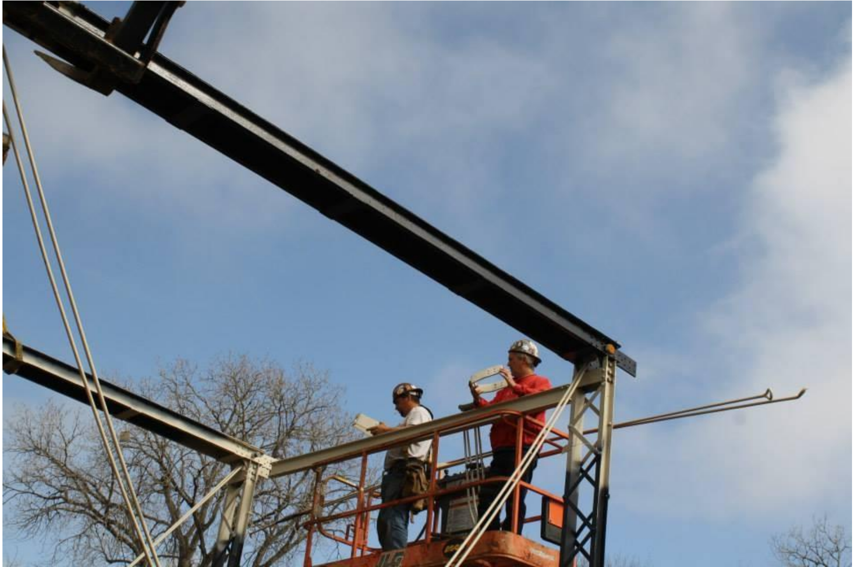
Reassembling the bridge.
