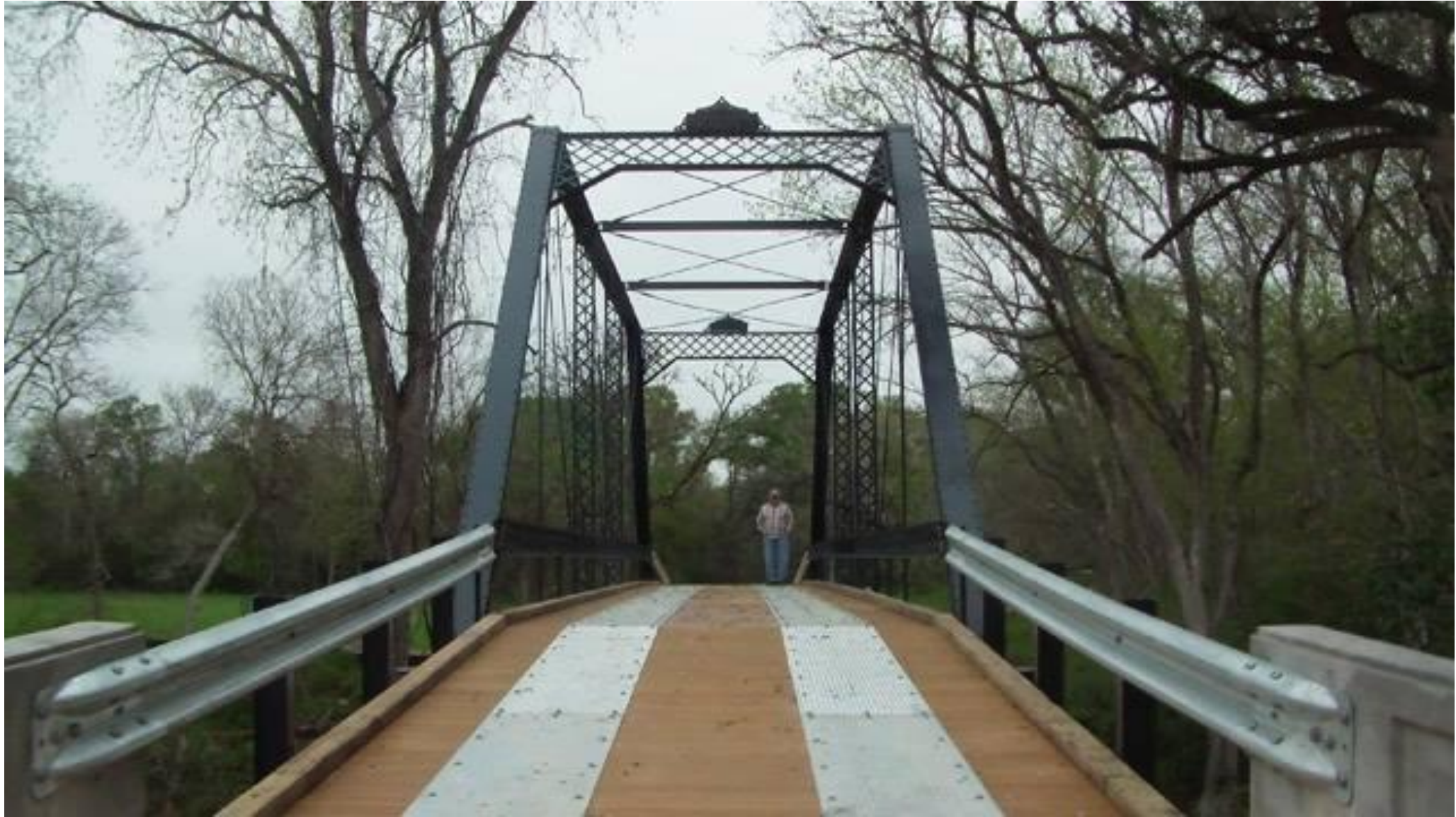
Bridge after restoration.
