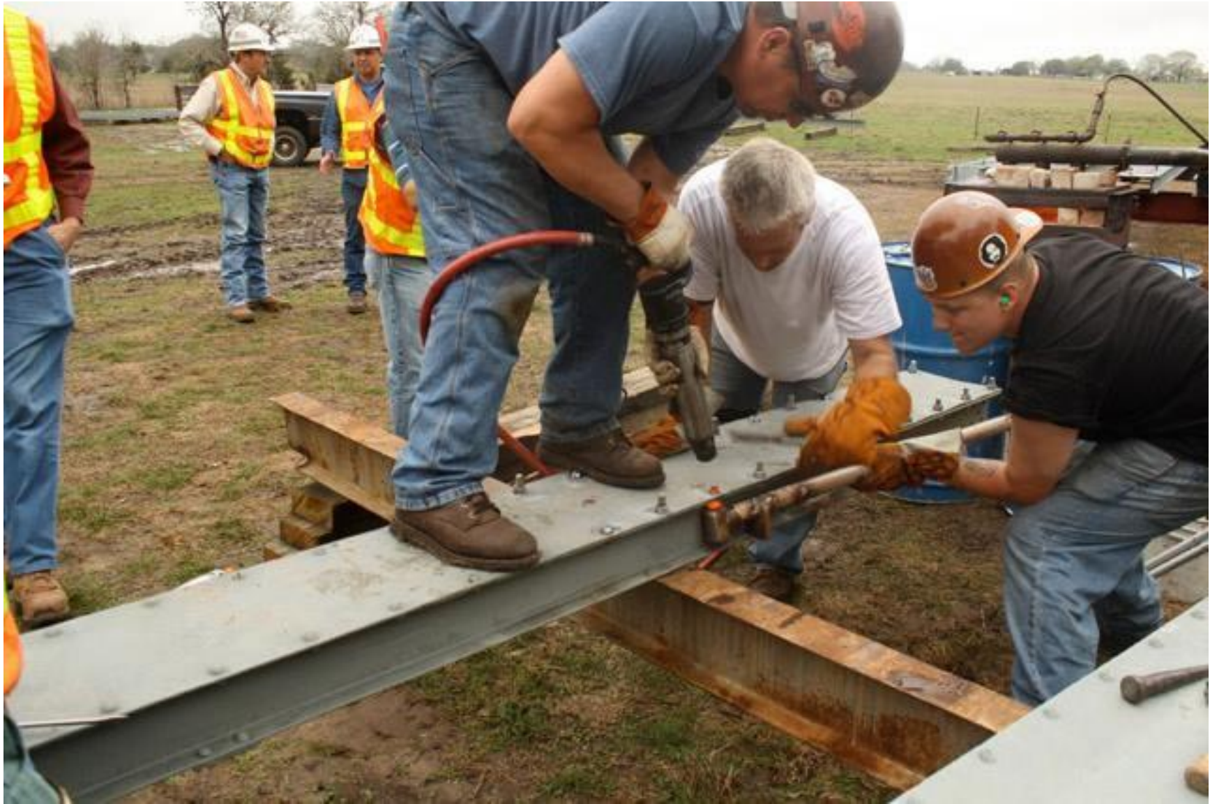
Riveting a cover plate.
