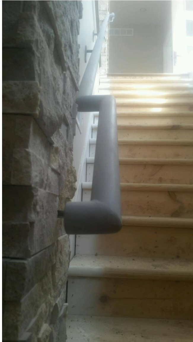
Completed installation of a custom-built contemporary residential steel railing.
