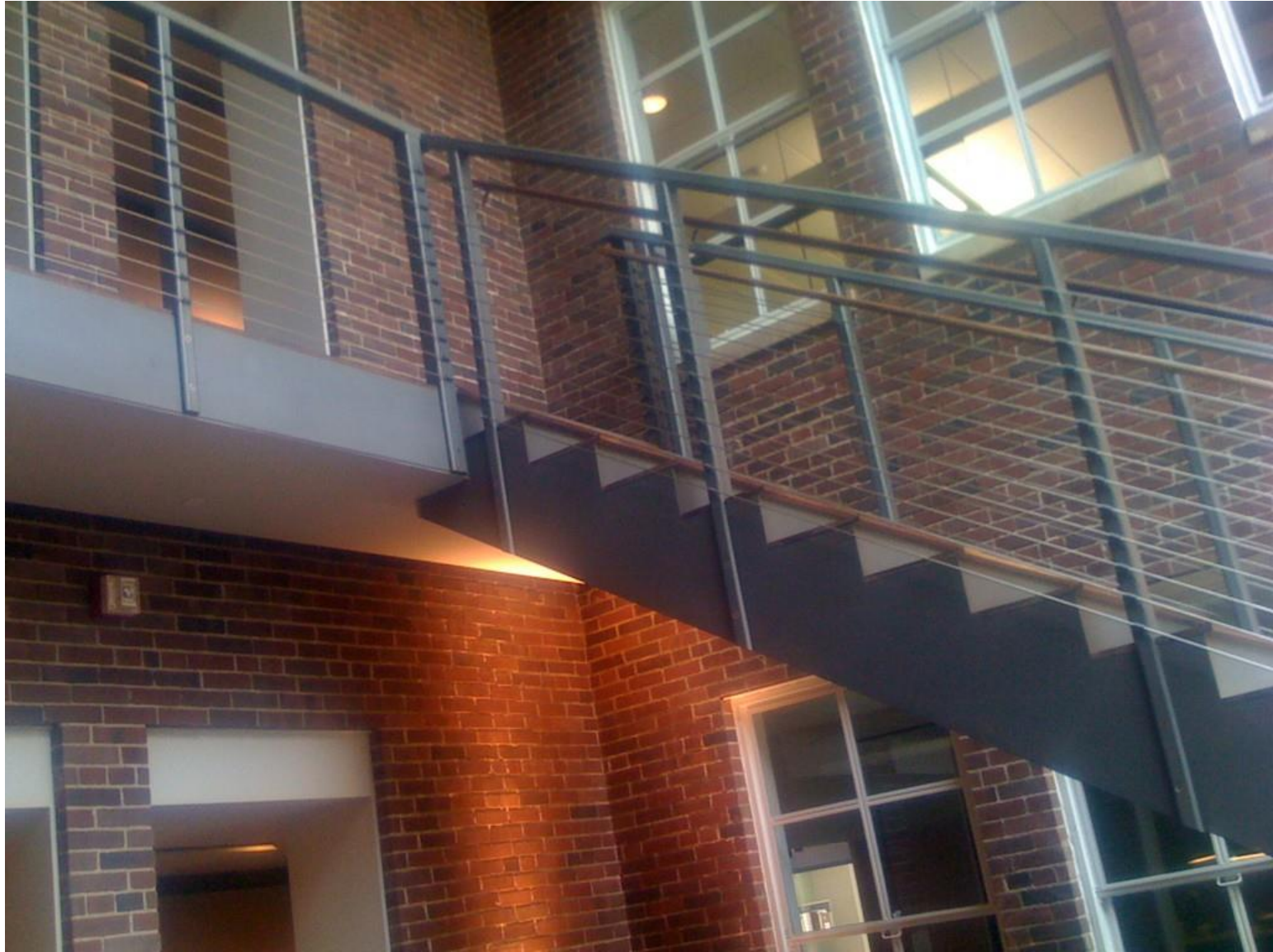
Custom fabricated modern railing by Bach Steel.
