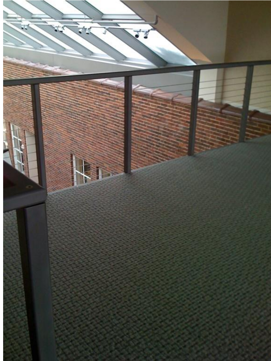
Custom fabricated modern railing by Bach Steel.
