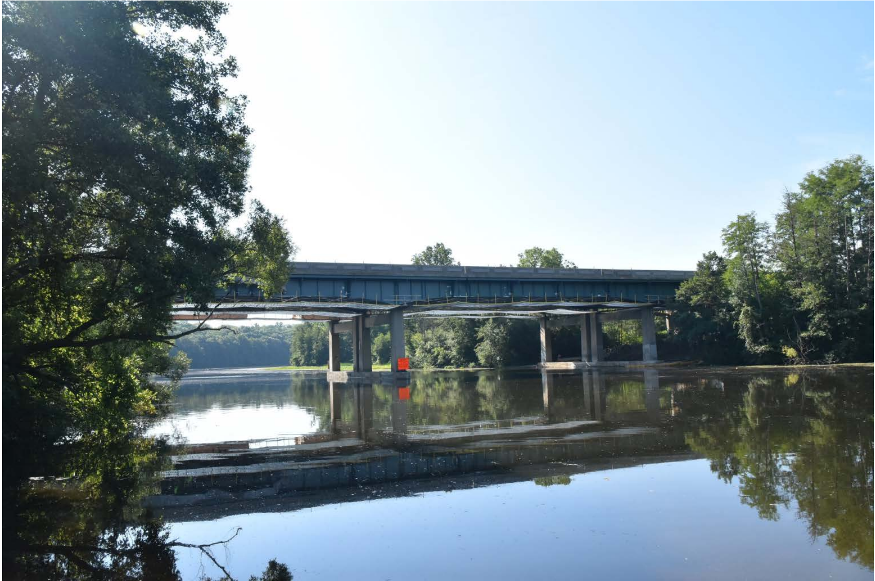
Overview of bridge.
