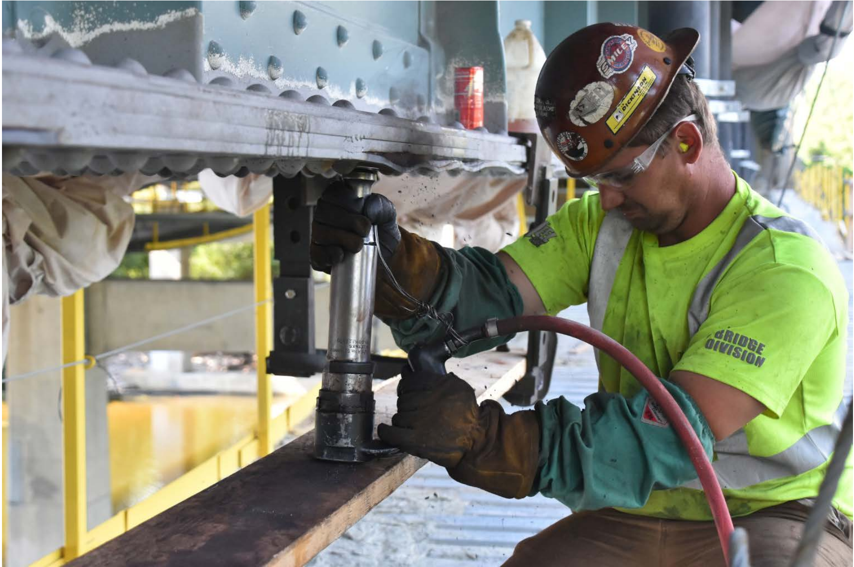
Driving the pack rust out.
