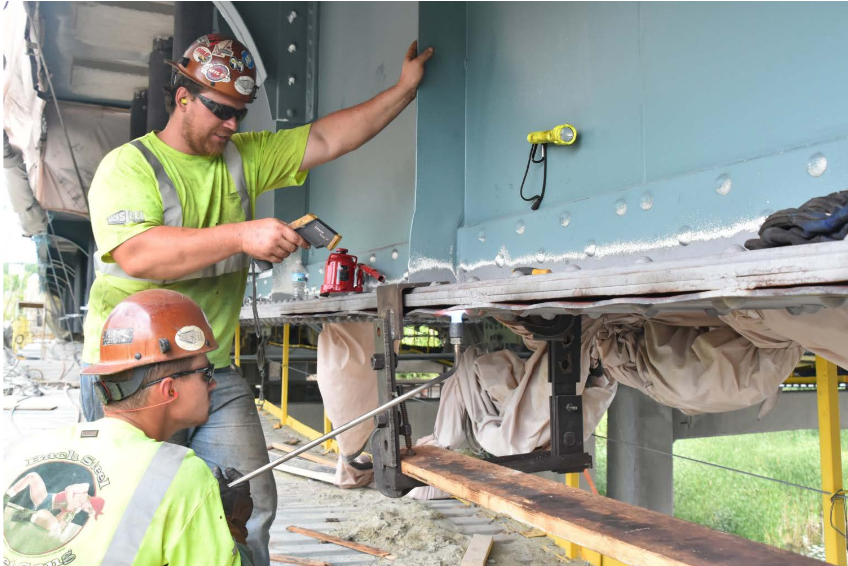
Careful temperature monitoring during heating was a requirement on this job.
