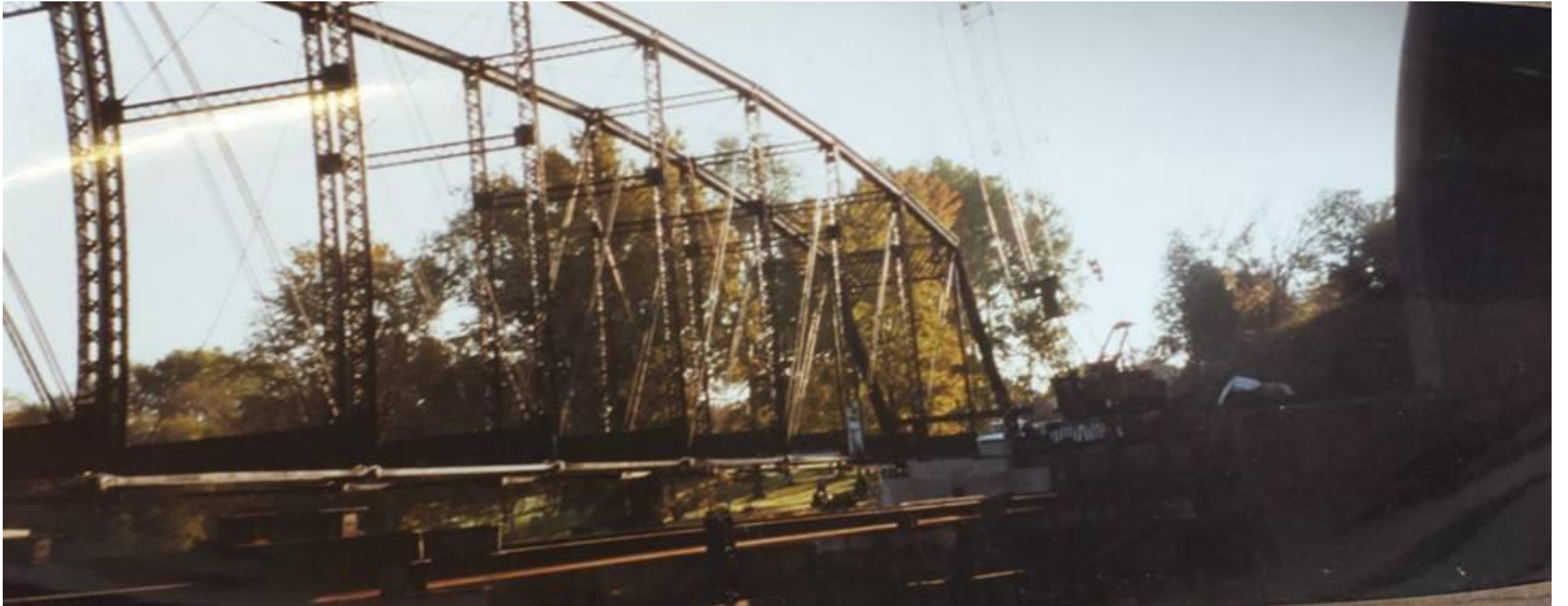
Erecting the bridge.
