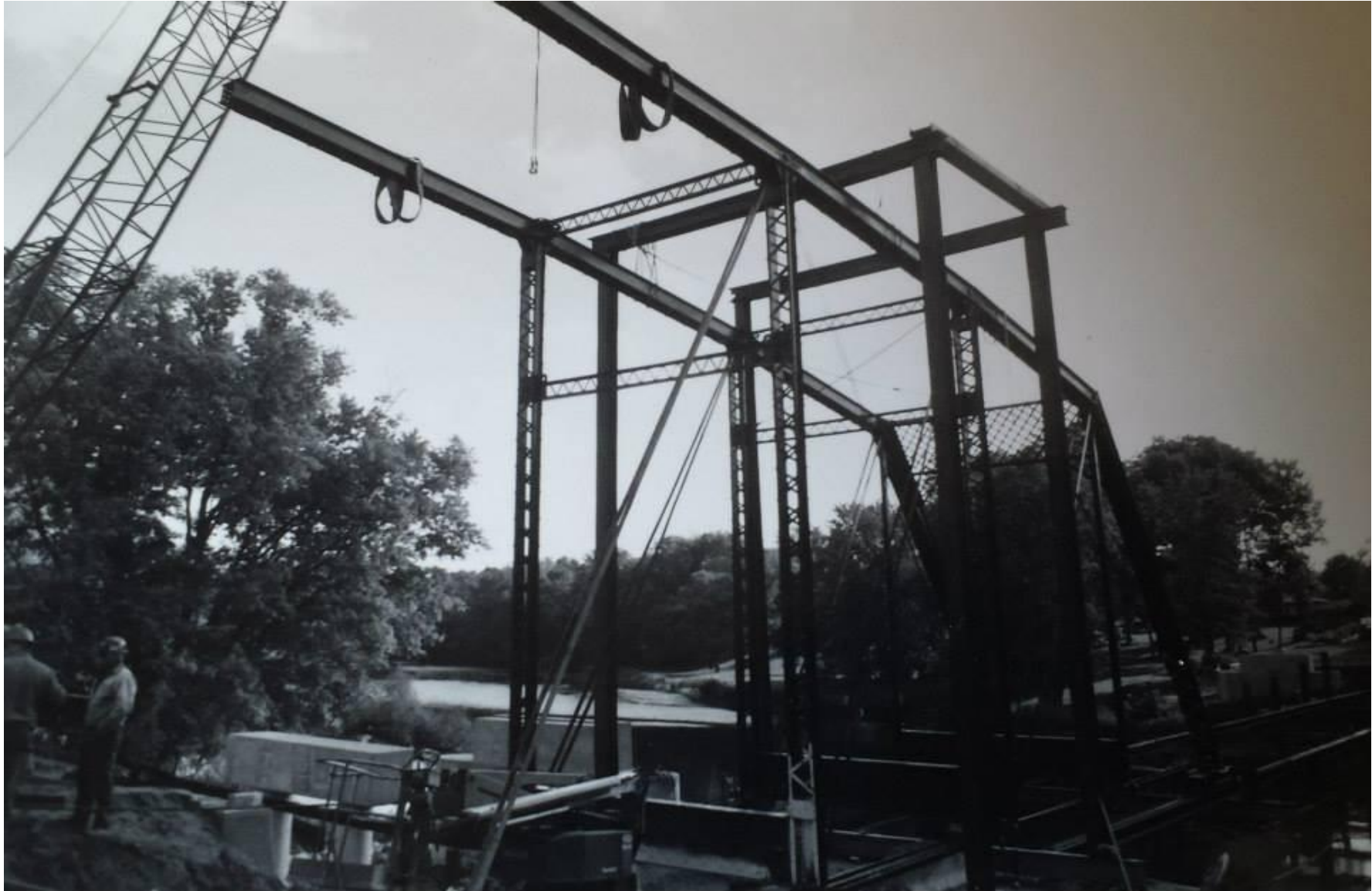
Erecting the bridge.
