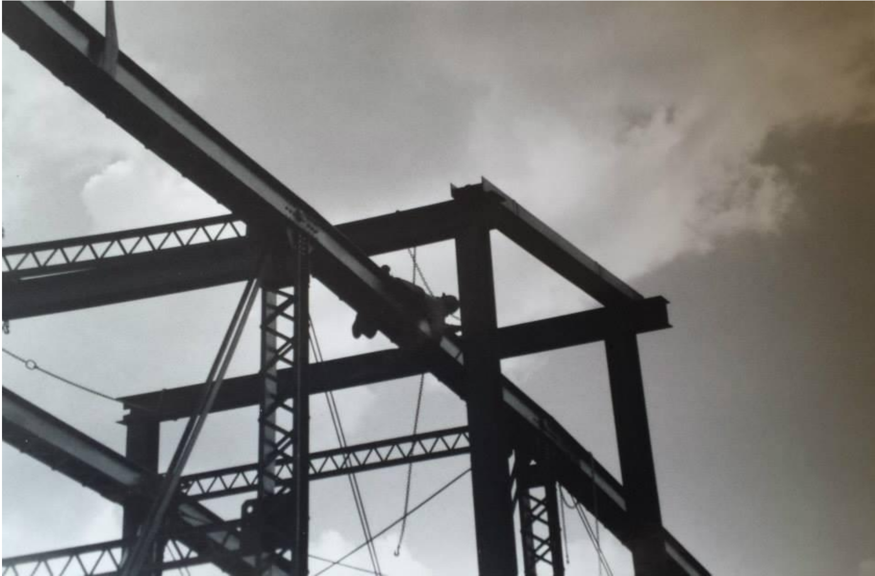
Erecting the bridge.
