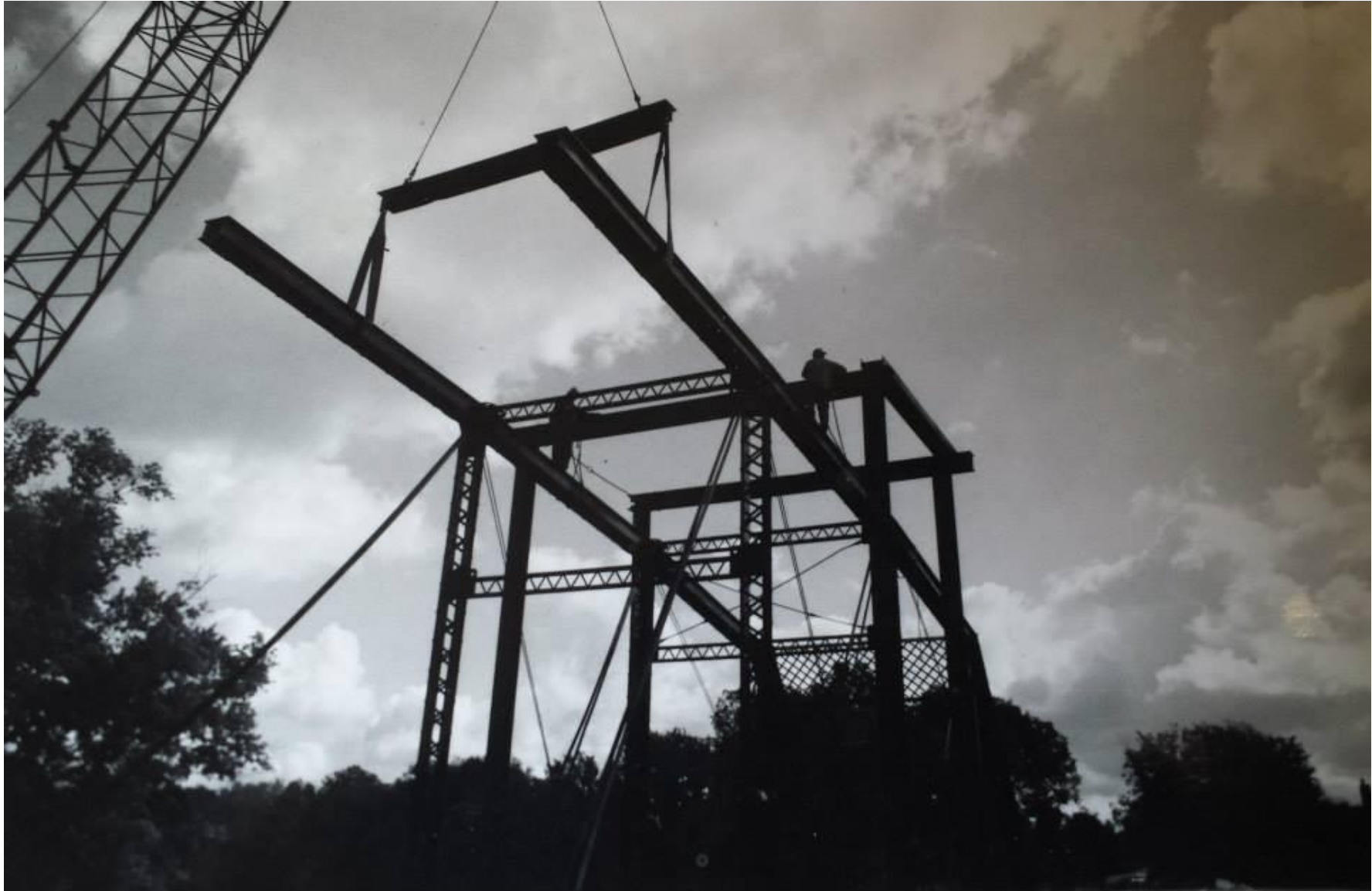
Erecting the bridge.
