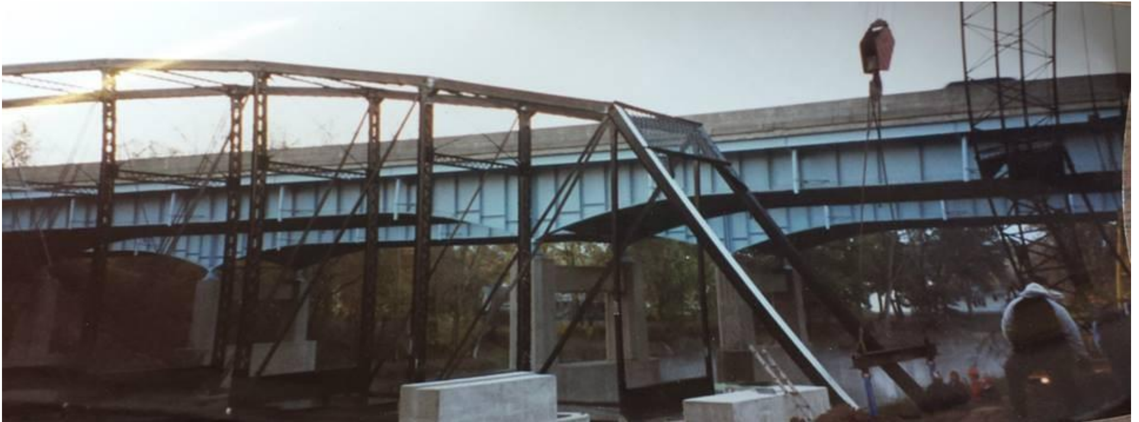
Here, the bridge is fully assembled on the tramway, and awaits being moved over to the adjacent pier.
