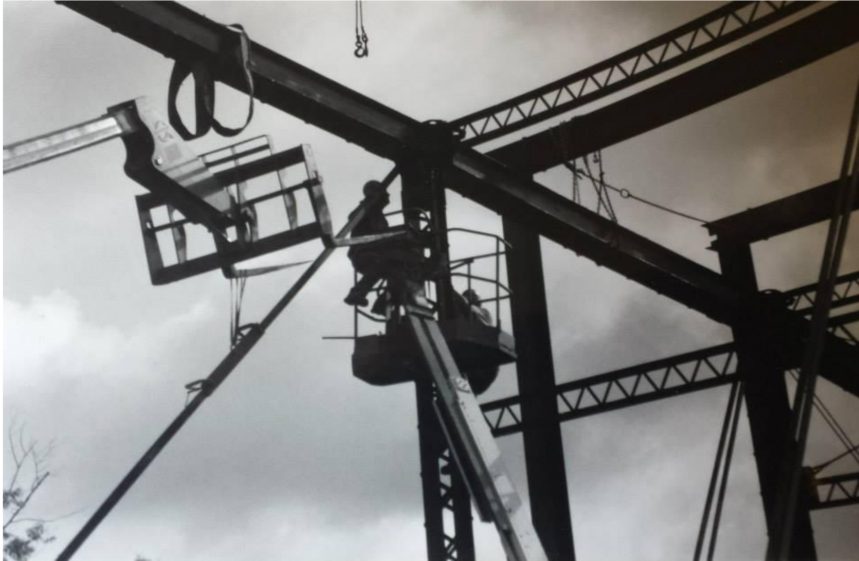
Erecting the bridge.
