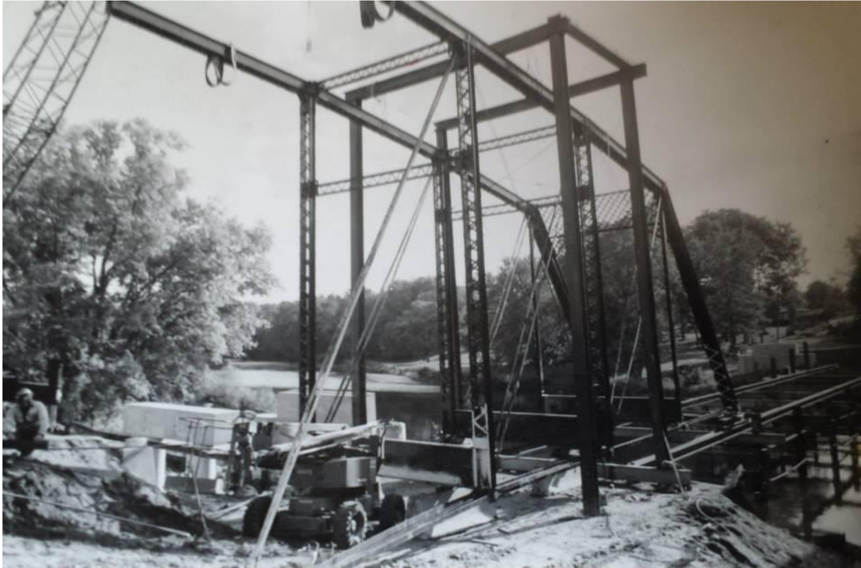
The bridge was erected in stages, one panel at a time, and moved out over the river on a tramway one panel at a time. Here a few panels have been erected.
