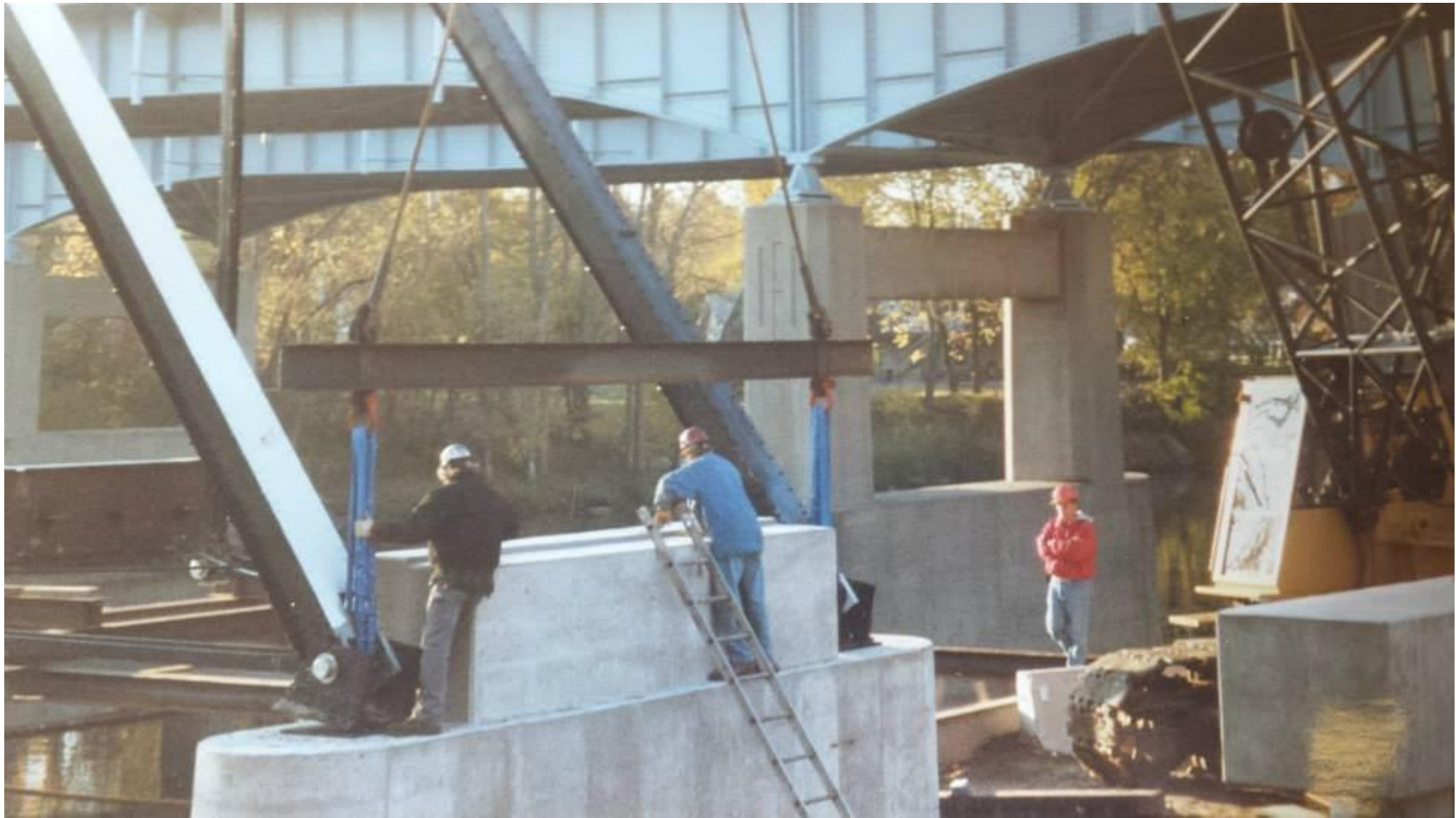
The bridge is positioned upon the new pier.
