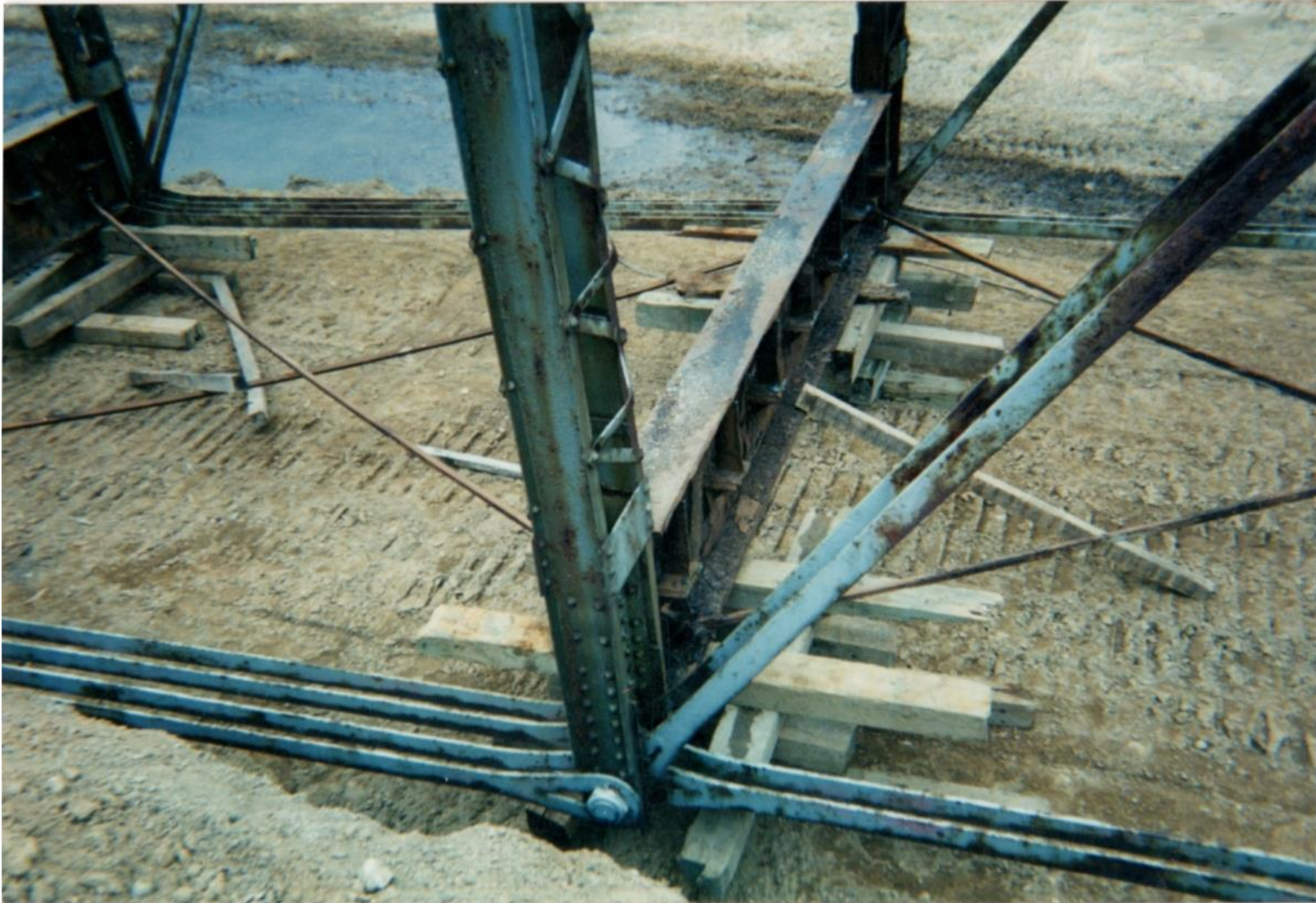
This photo shows the typical condition of the bridge after it was removed from its original location, before restoration.
