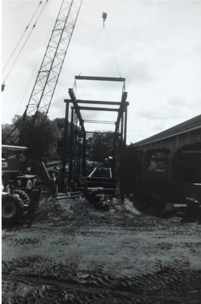
Erecting the bridge.
