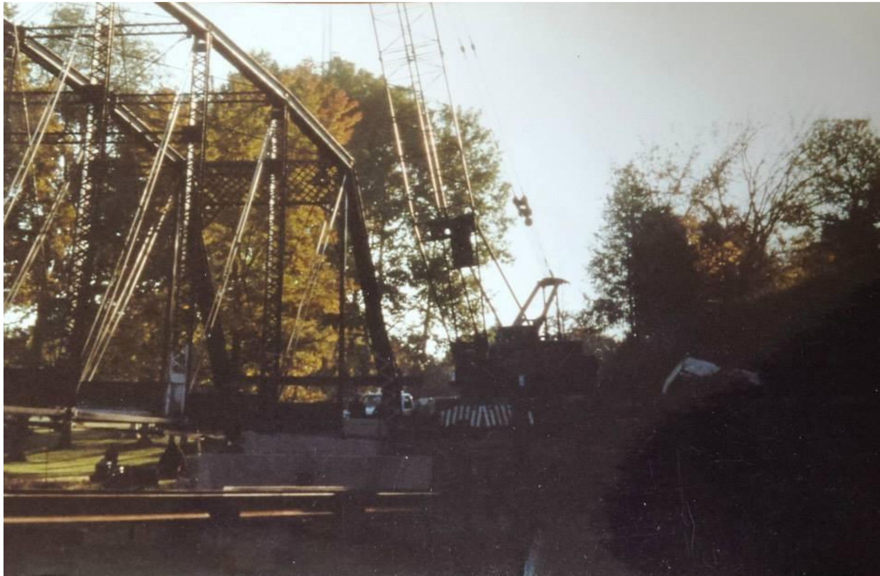
Erecting the bridge.
