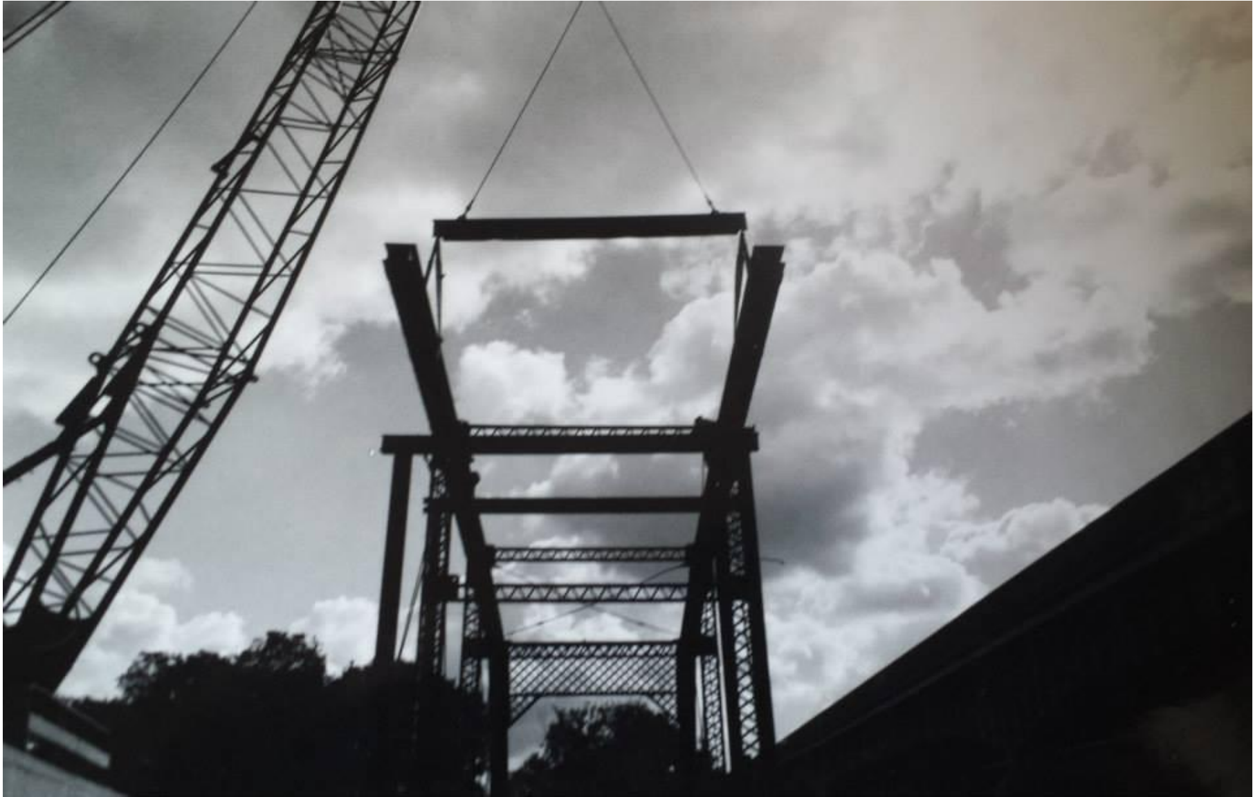
Erecting the bridge.
