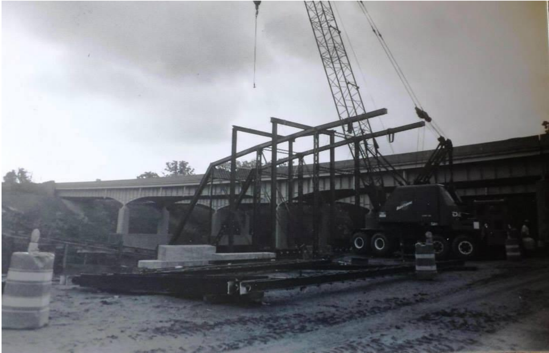
Erecting the bridge.
