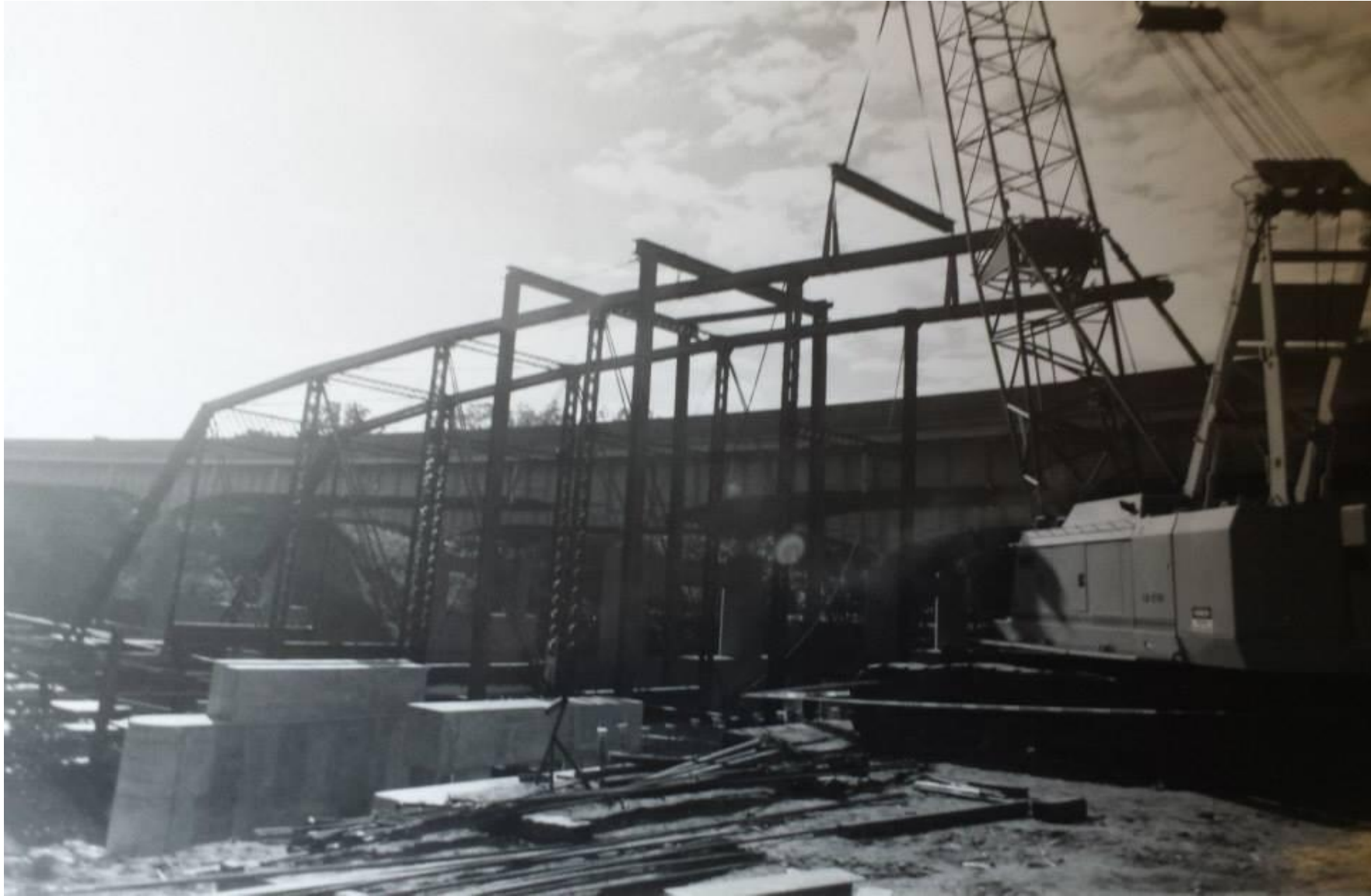
This photo shows the bridge after a substantial number of panels were erected.
