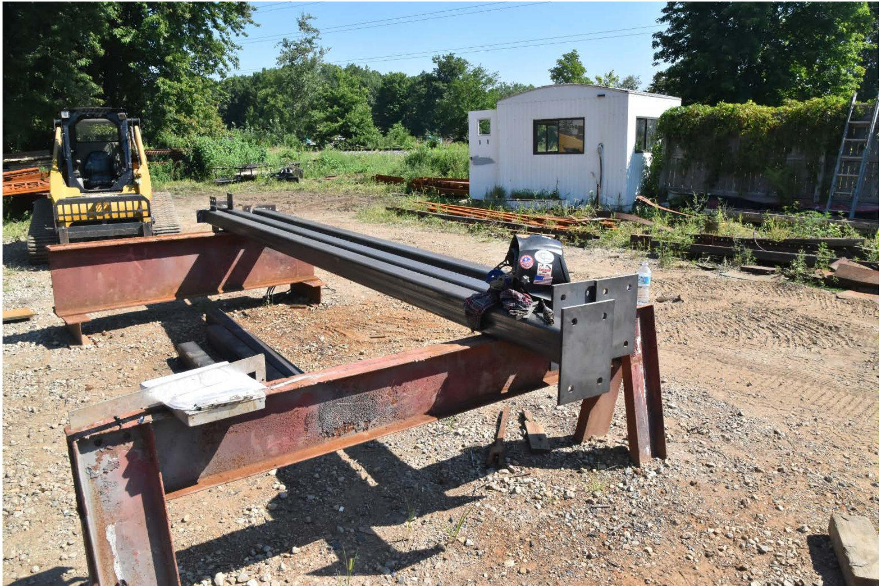
Columns and beams.
