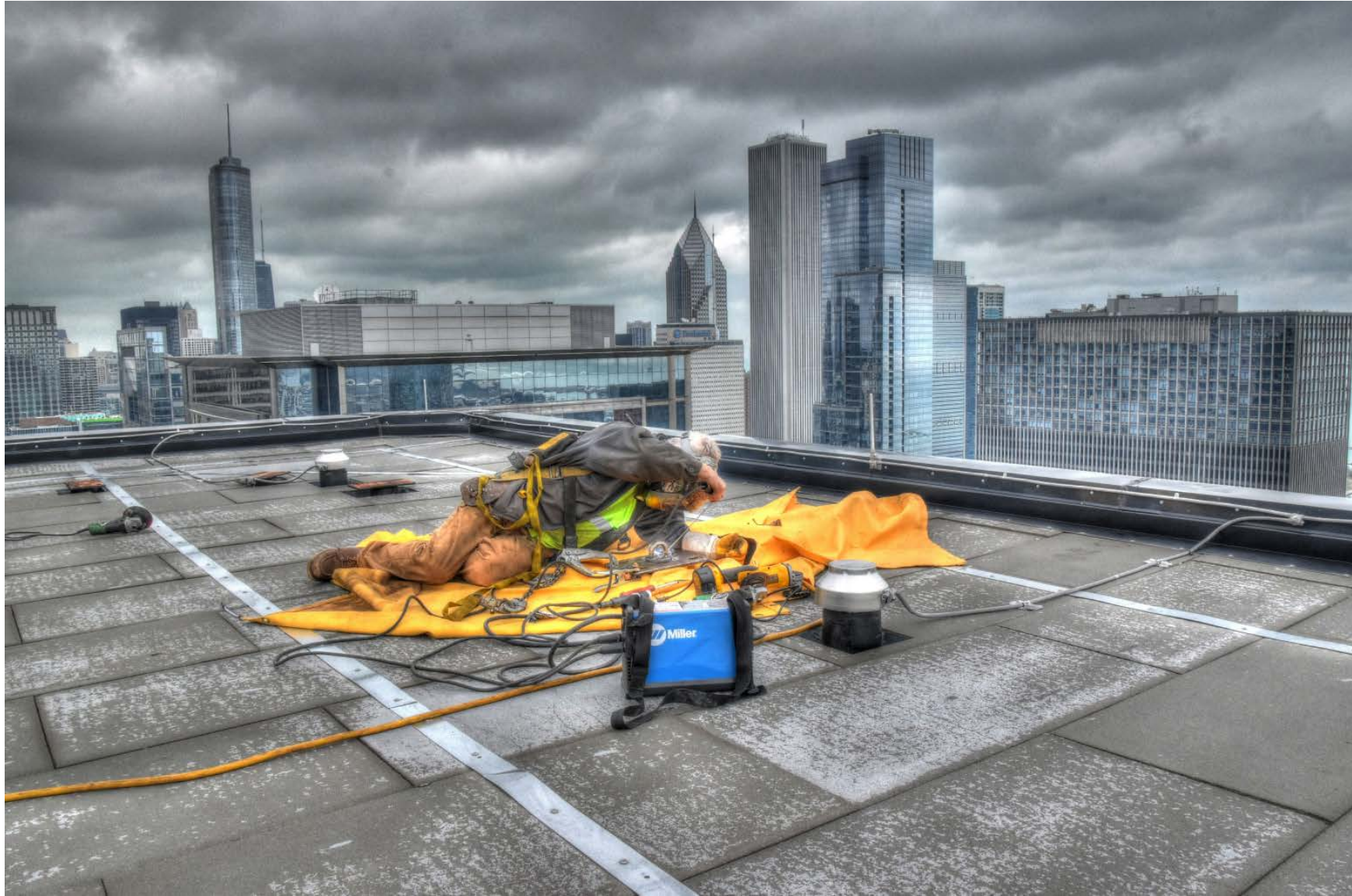
Welding anchors in place.
