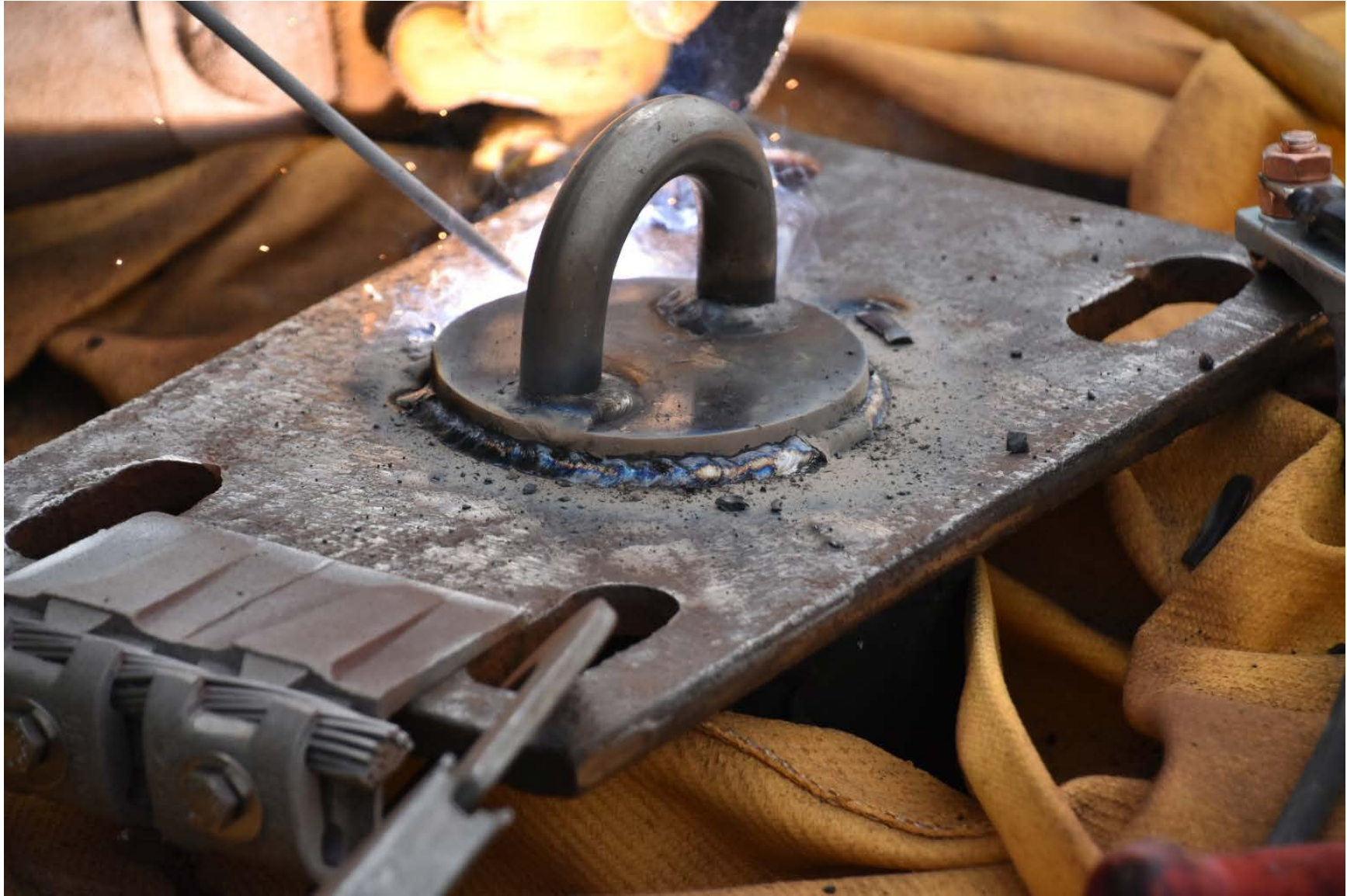
Welding anchors in place.
