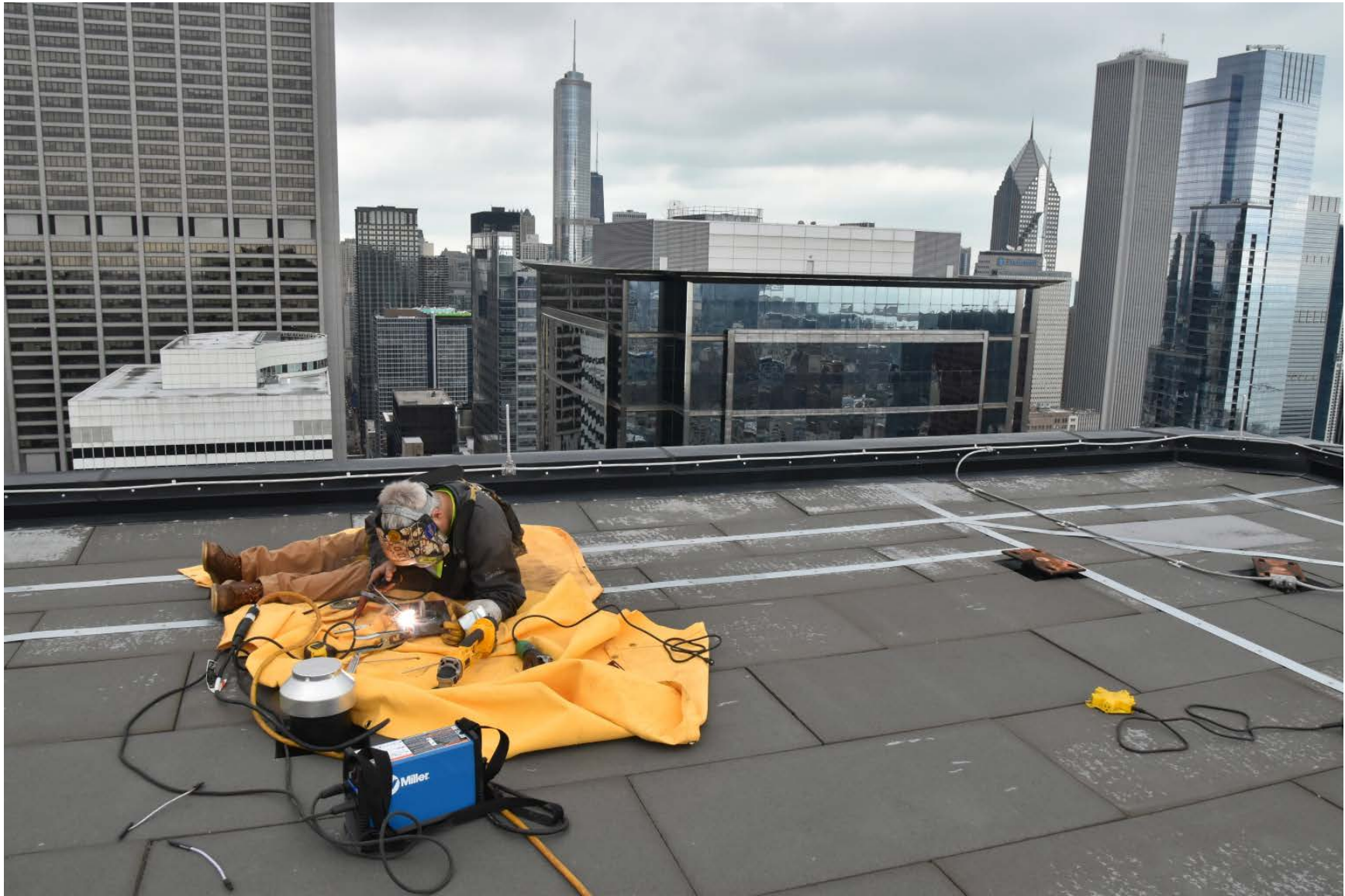
Welding anchors in place.
