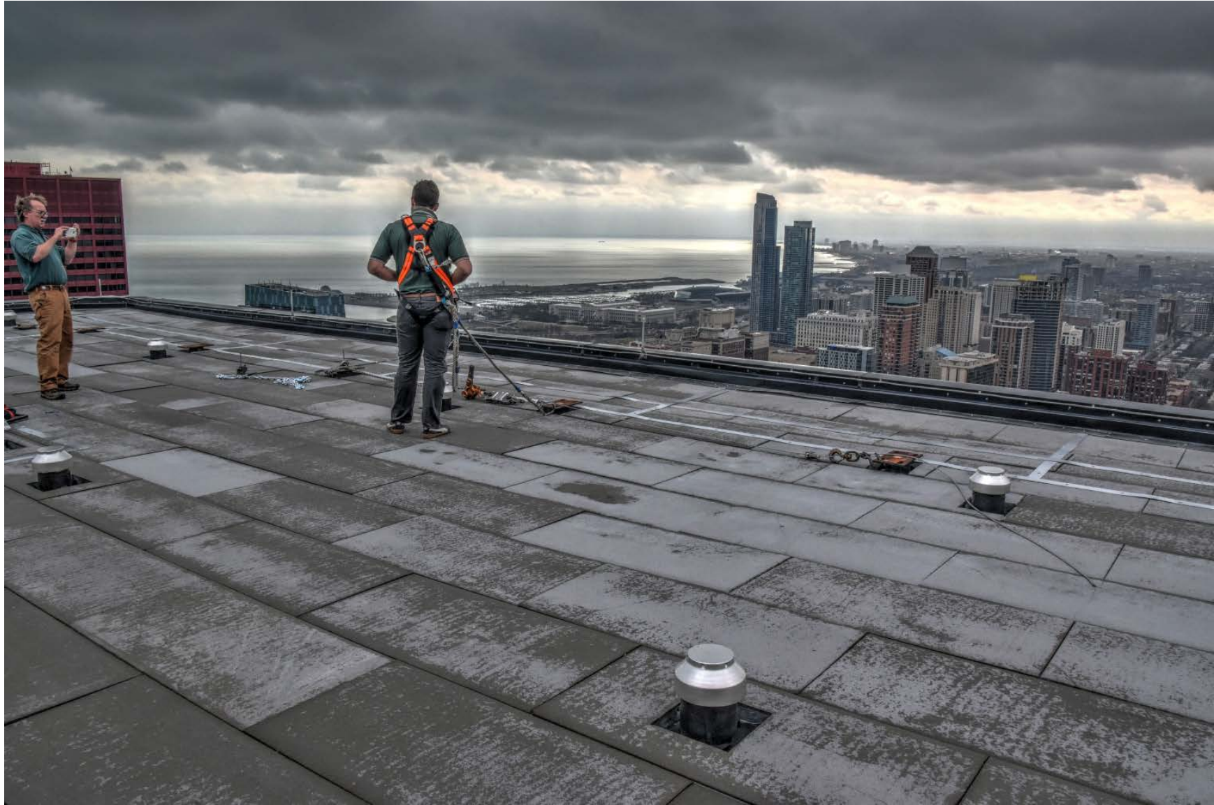
Testing of anchors after installation by Engineer.
