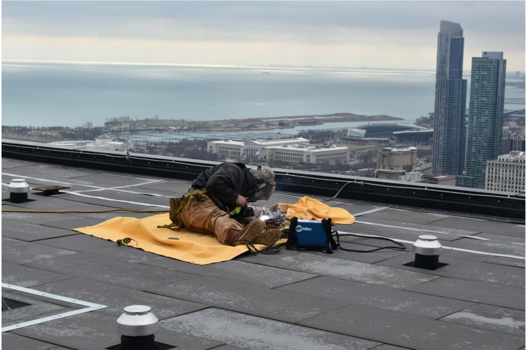
Welding anchors in place.
