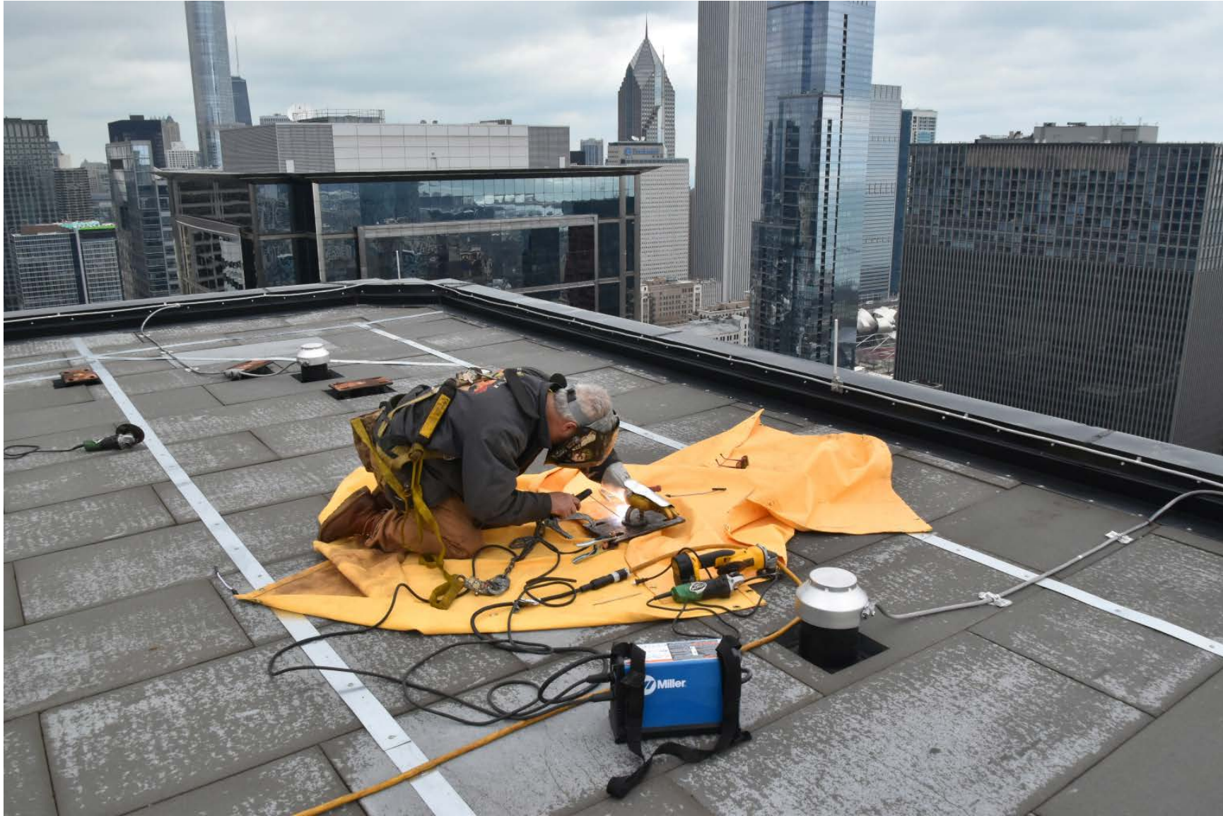
Welding anchors in place.
