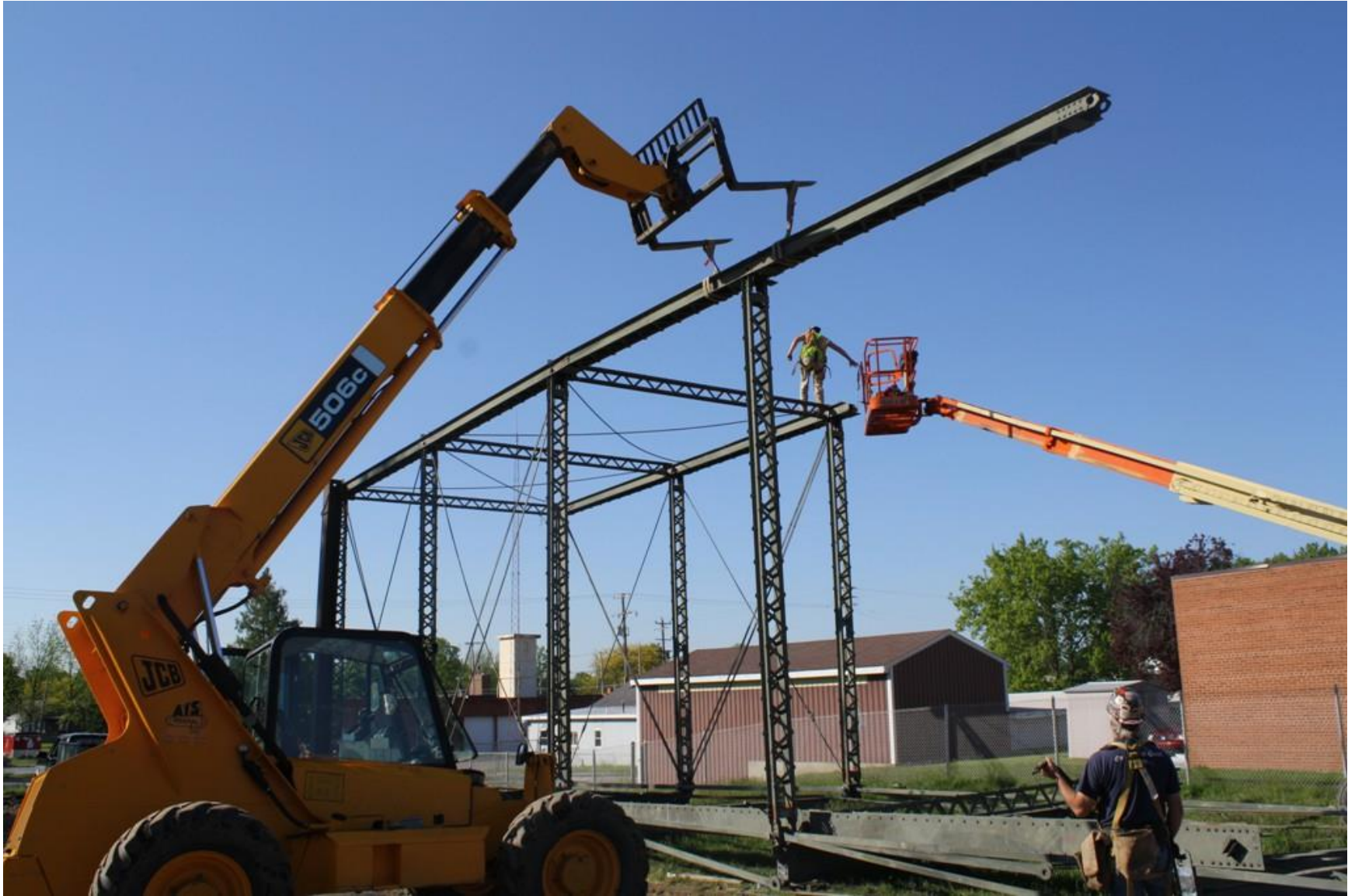
Reassembling the restored bridge.
