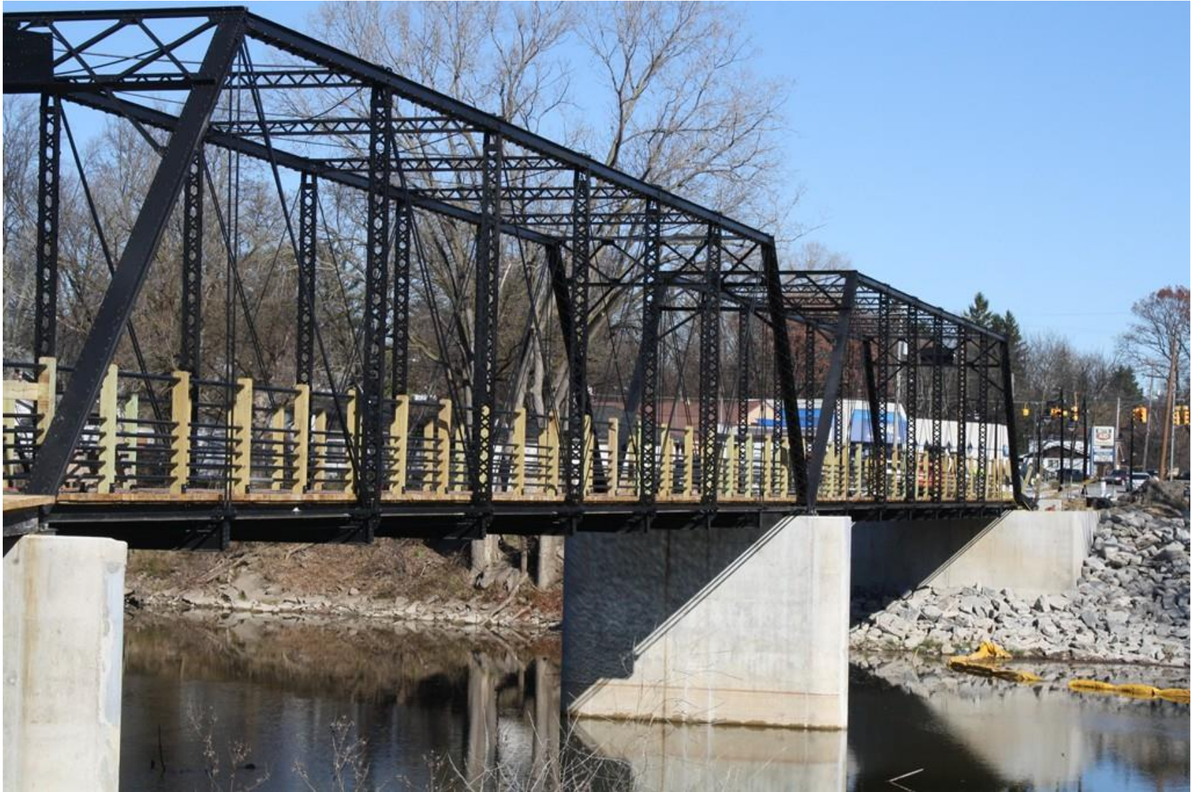
Bridge trusses after restoration and placement on the new substructure.
