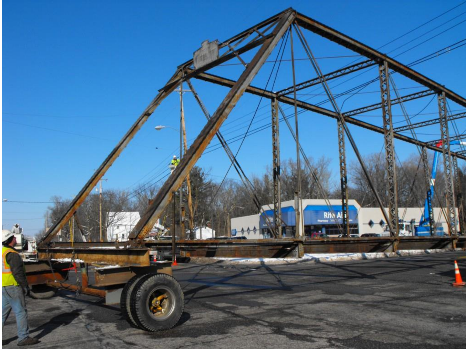
Moving the bridge down the street to where it would be dismantled.
