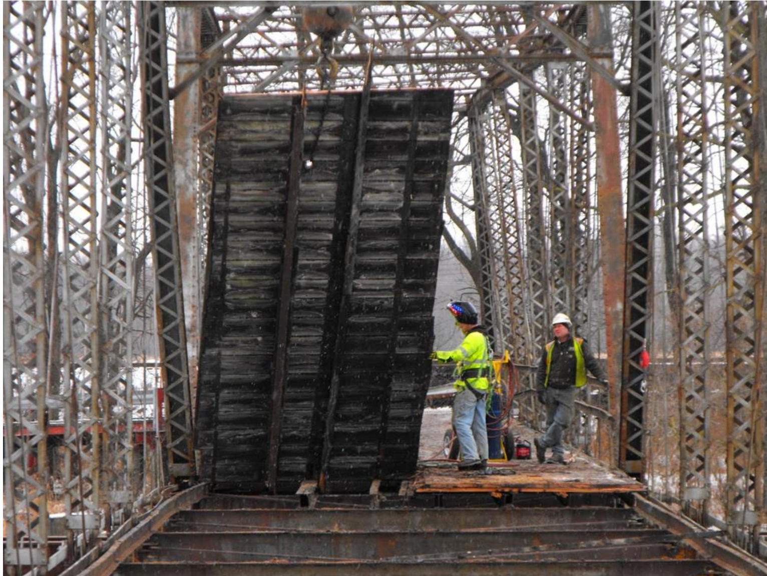
Removing the deck.
