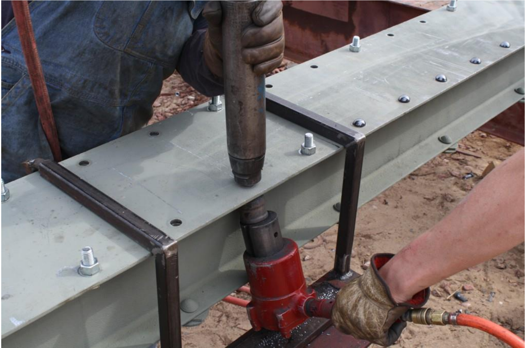
Driving a rivet into the top chord. The entire cover plate was highly deteriorated, so the old cover plate was removed and a thicker cover plate was riveted on in its place to the original channels.
