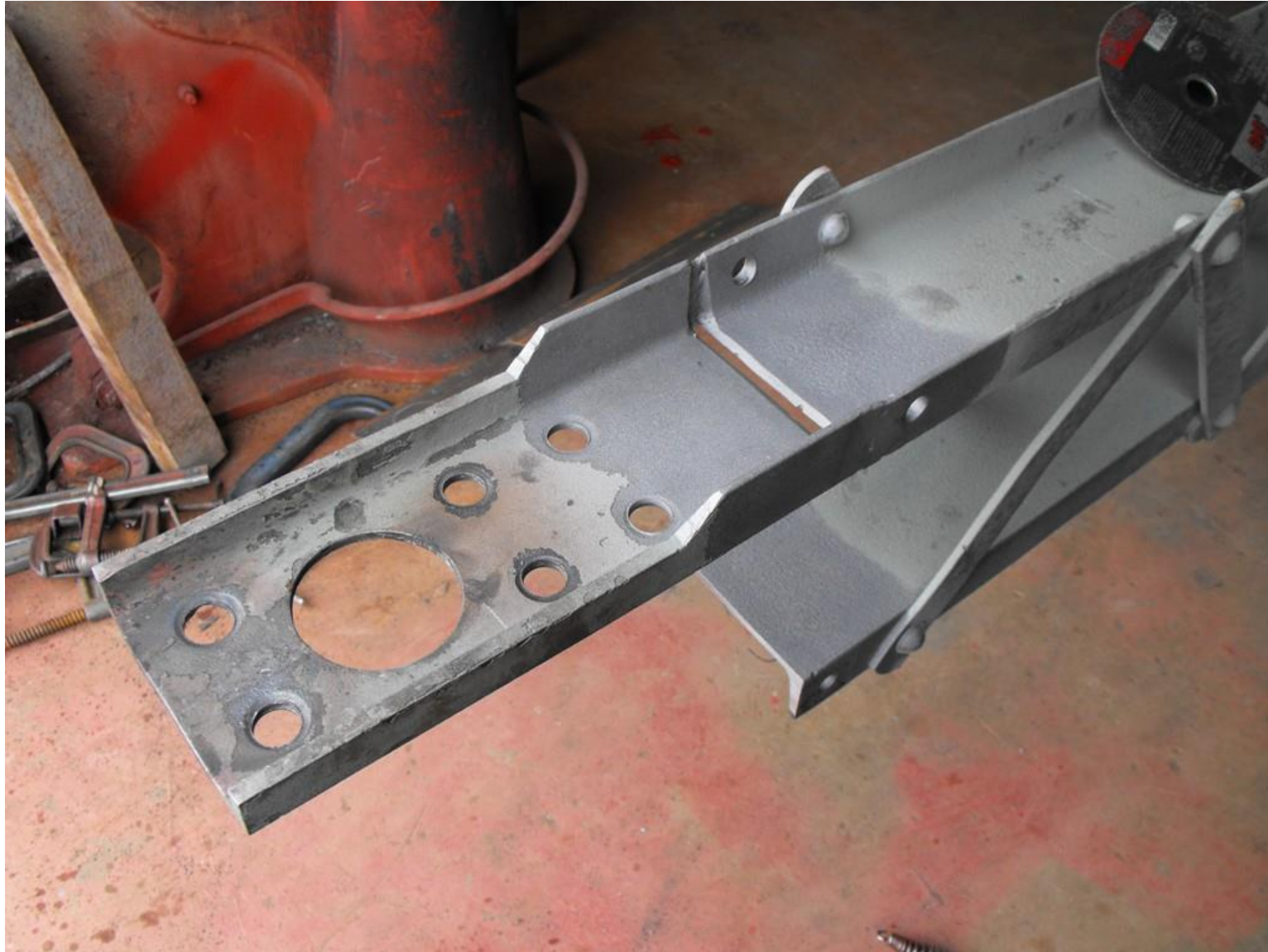
A replicated section of vertical member (to left) being welded onto the original portion of the member.
