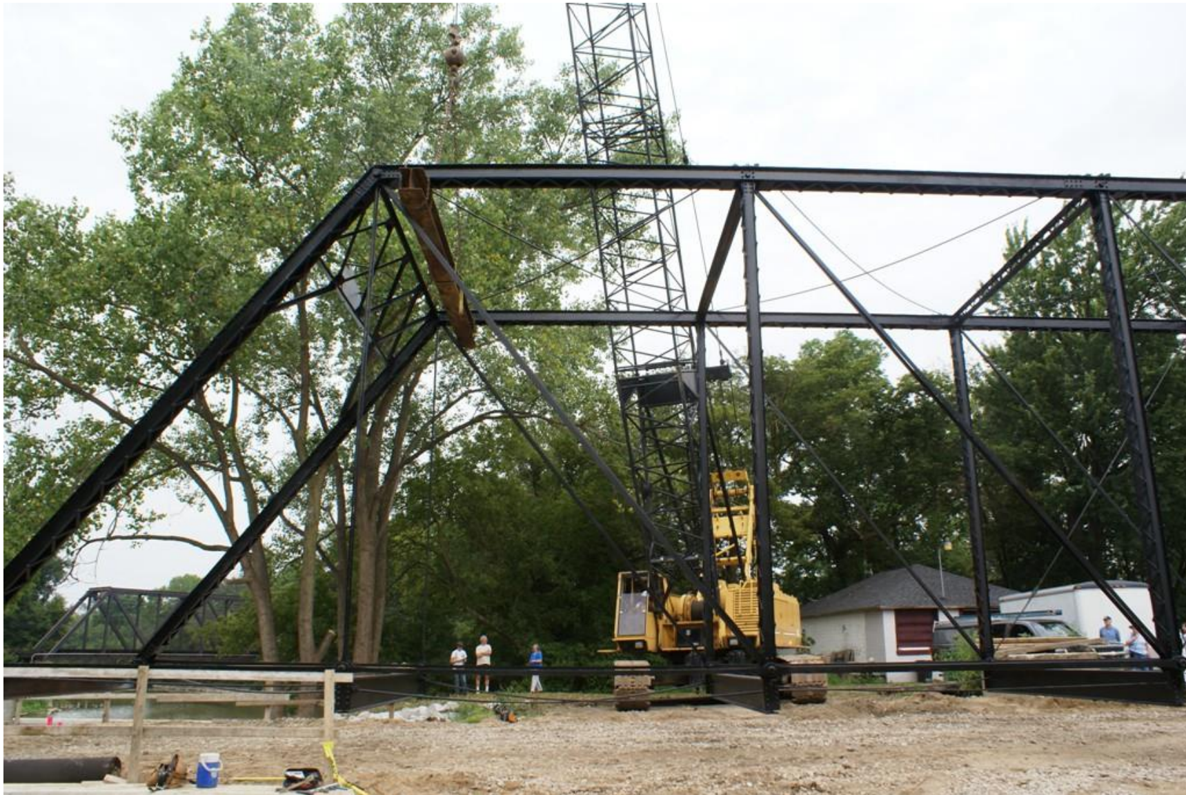
Preparing to lift a restored span back over the river.
