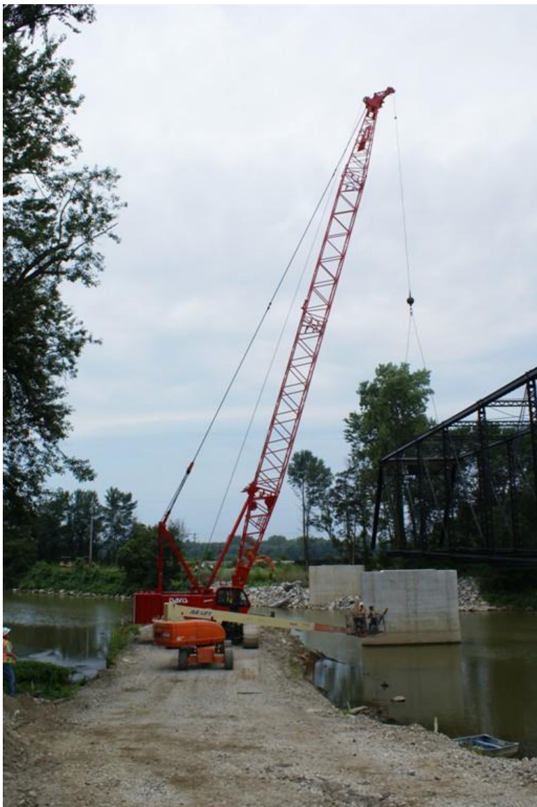
Lifting a restored span back over the river.
