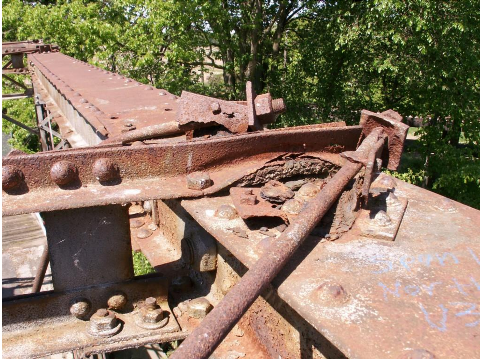
Bridge before restoration
