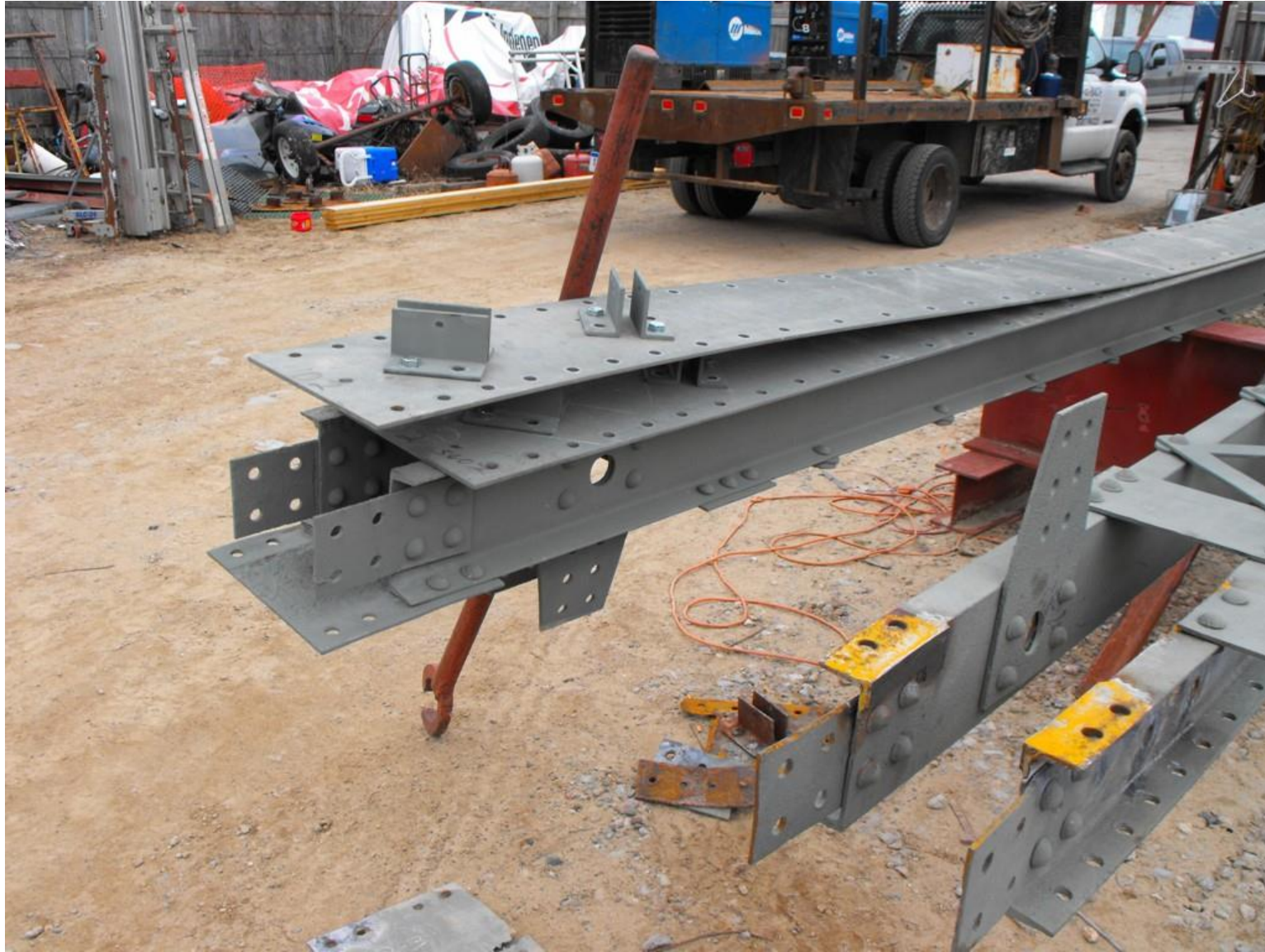
Sitting behind a vertical member is a section of top chord awaiting a new cover plate to be riveted onto it.
