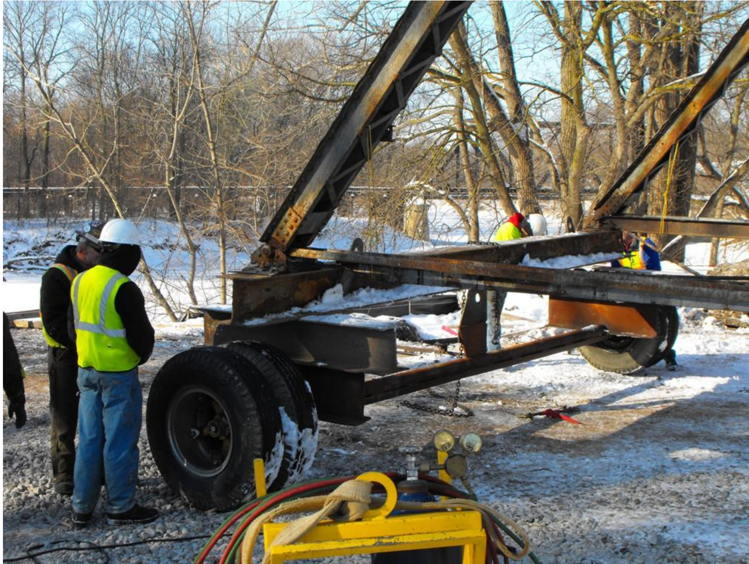
Preparing to move the bridge down the street to where it would be dismantled.
