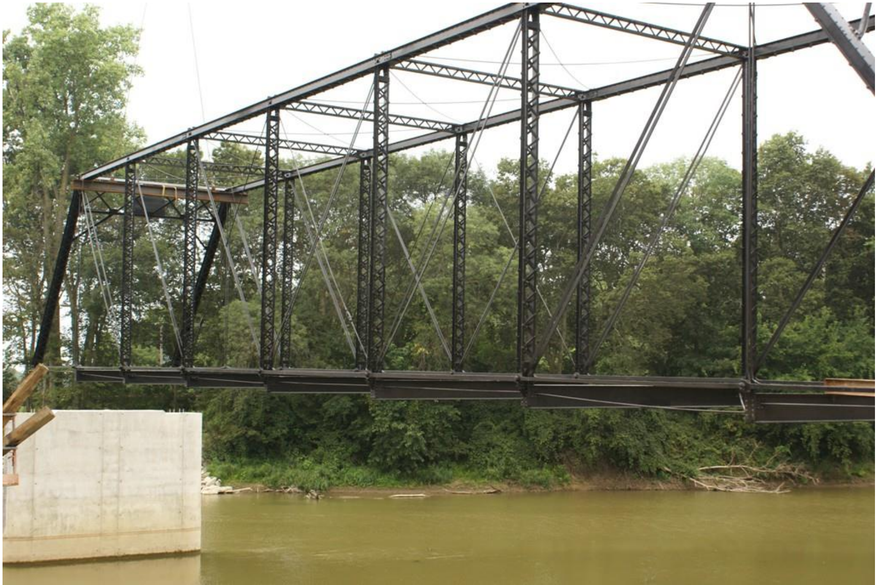
Lifting a restored span back over the river.
