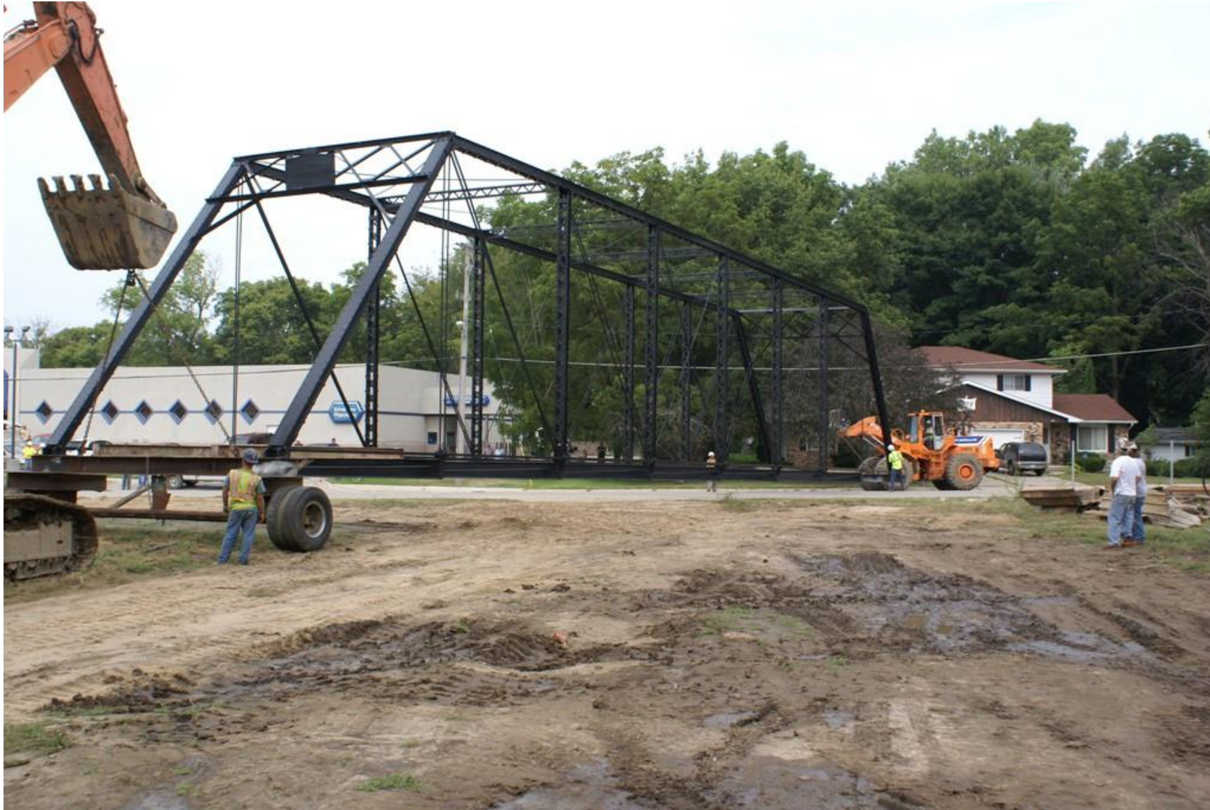
Moving a restored span back down the street back to the project site.
