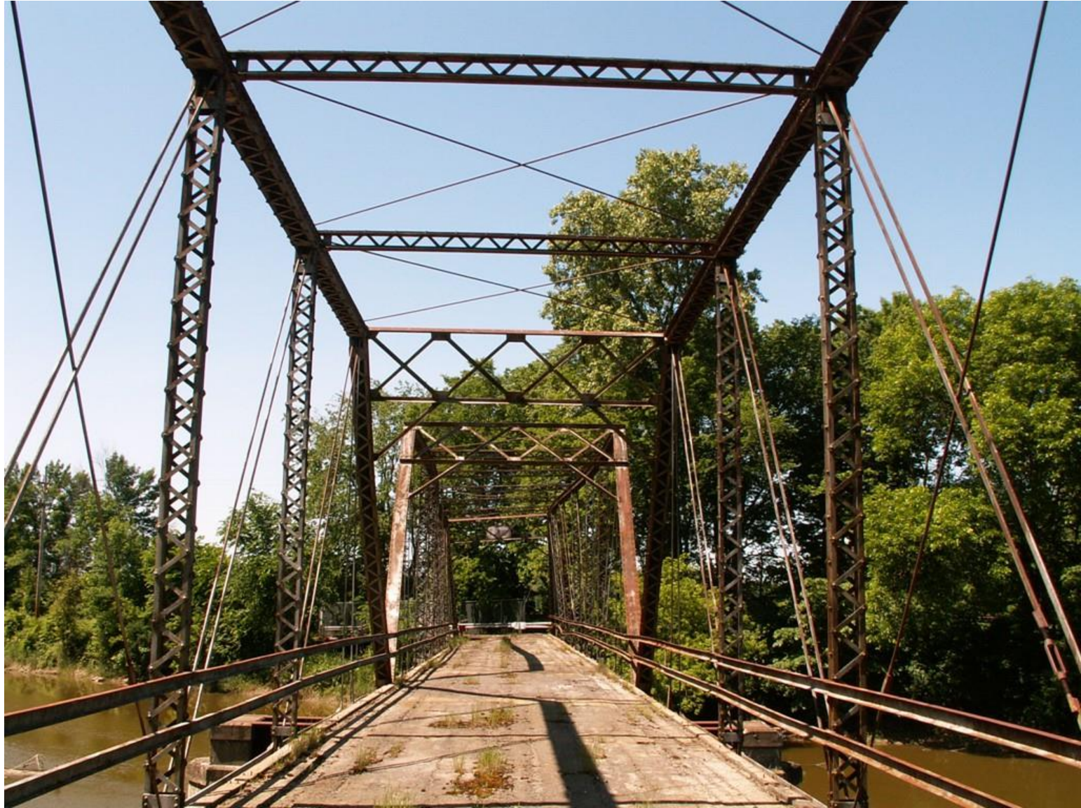
Bridge before restoration
