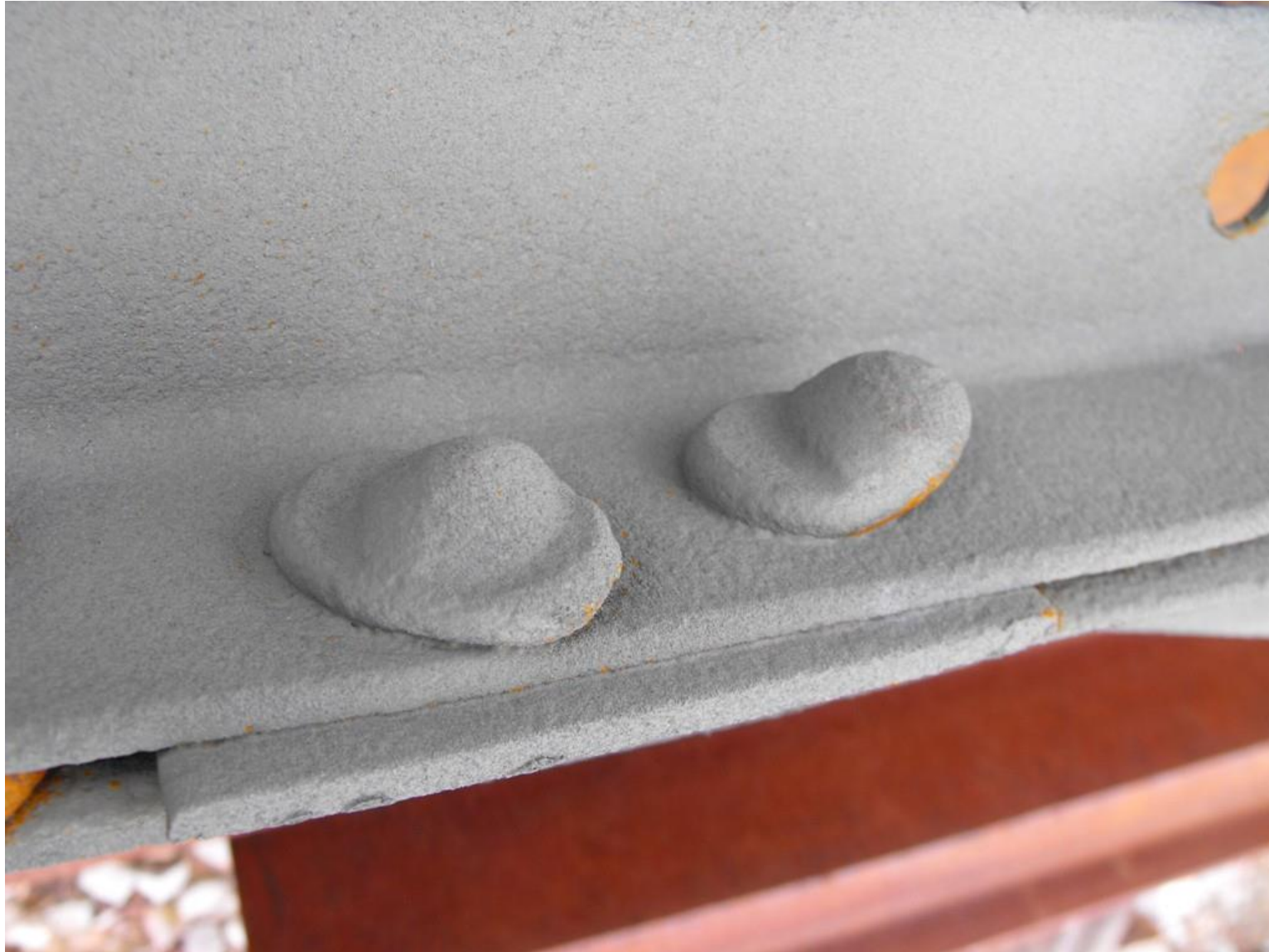
These are original rivets found on the Bridgeport Bridge that are obviously not driven very nicely. Yet, despite their imperfections, they worked for 100 years! The rivets driven by Bach Steel will look much nicer than these and will be ready for their century of service!
